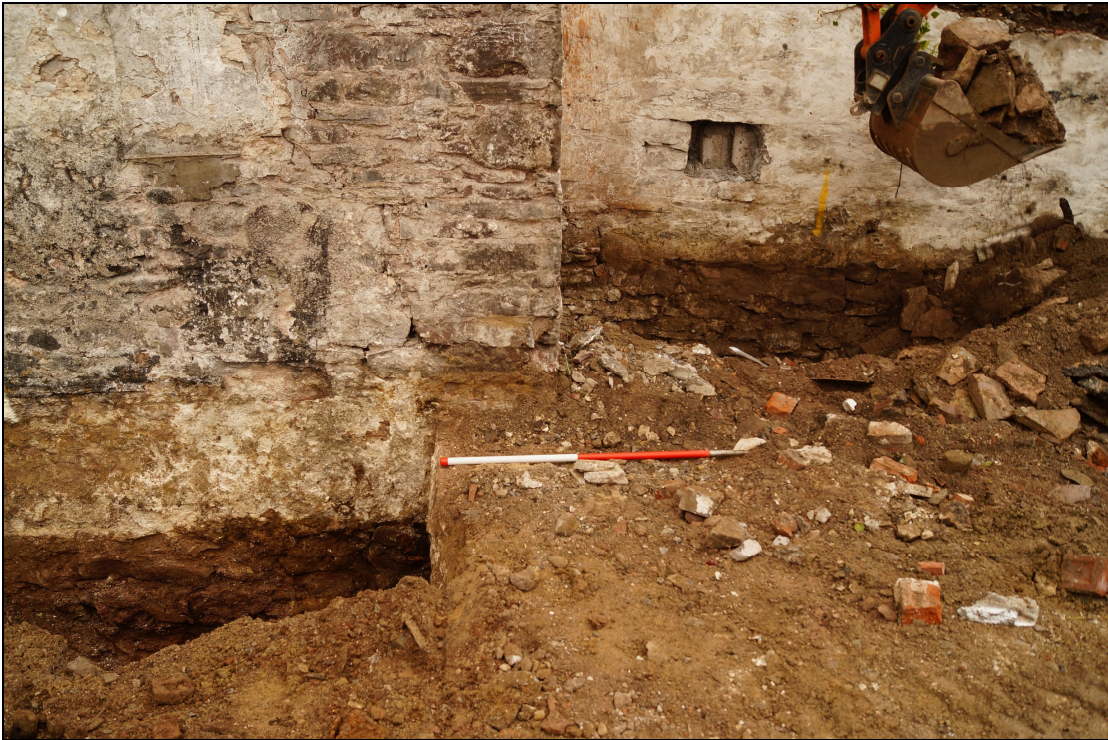
Plate 7: OPL2019_107, Western end of Trench A excavated alongside the adjoining wall of The Pelican to the south showing (008) looking south-southeast.
