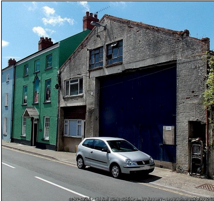
Figure 3: This photo taken by Jaggery in 2014 shows the bus depot building before it was demolished.
