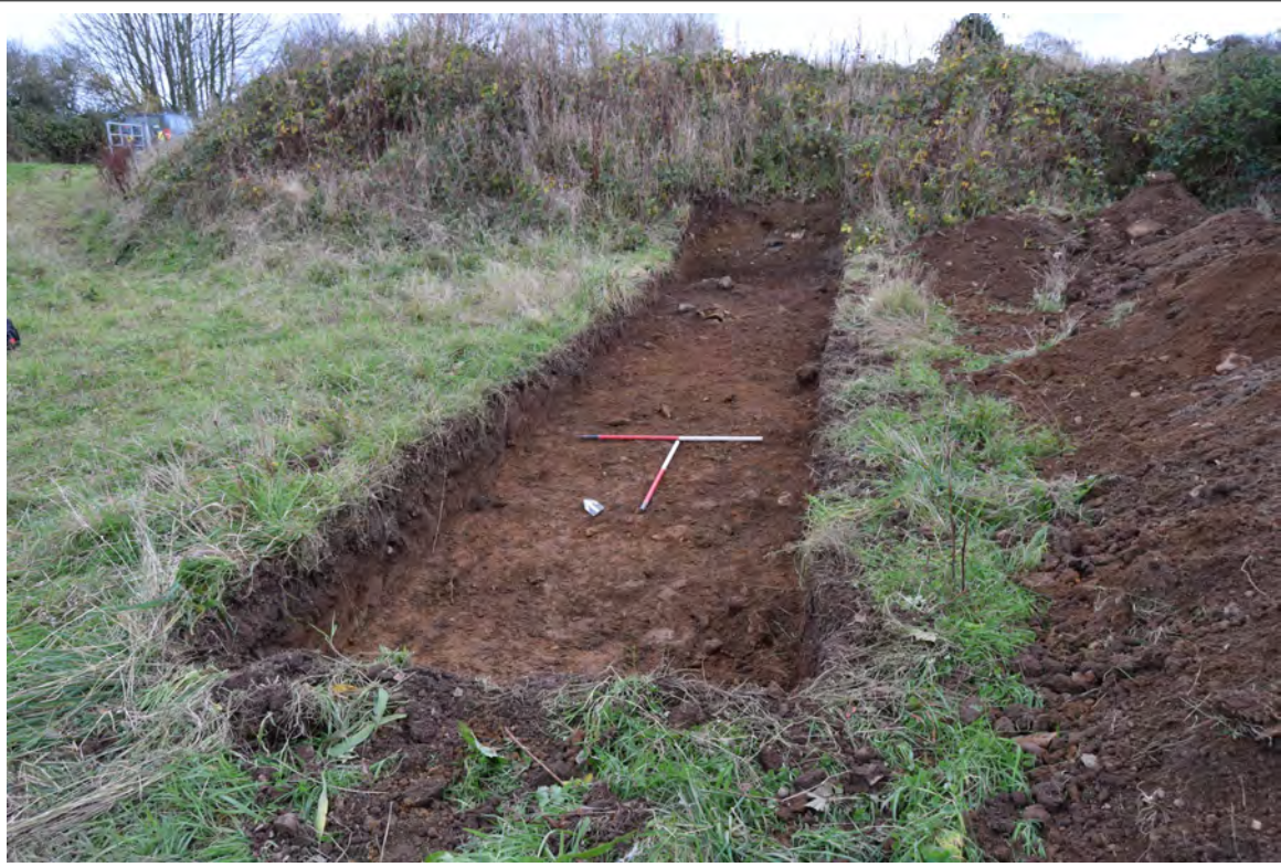
Plate 10. Trench 3, looking NE. Scales 2 x 1m
