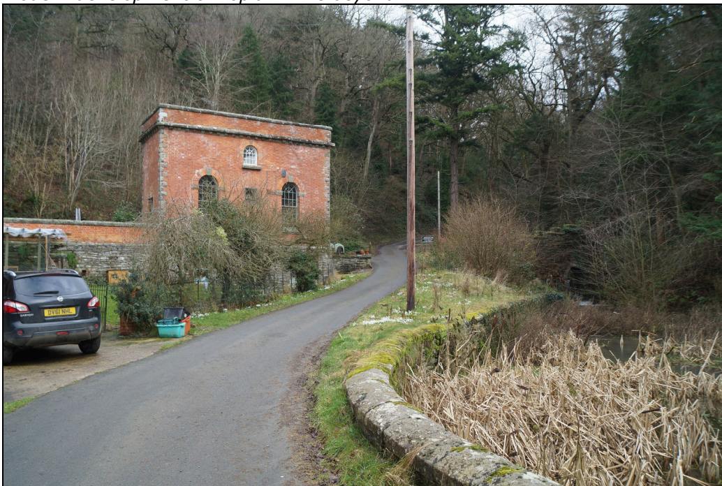
Plate 26: The view of the Old Cable House from the road, looking east-northeast. The leat and pool system is to the right. Park Cottage is just out of view to the left.
