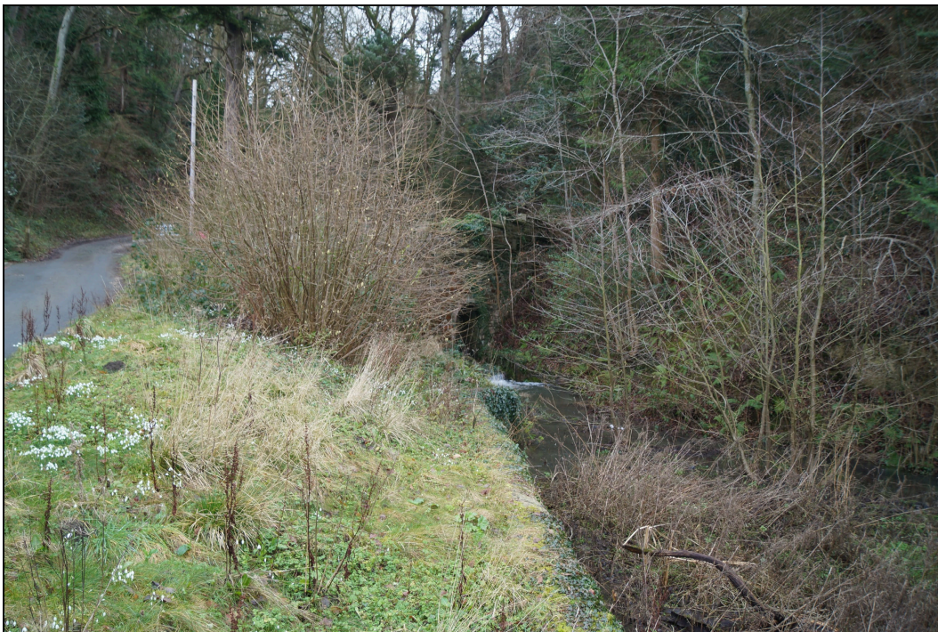
Plate 27: A view of the leat and pool system looking east-southeast.
