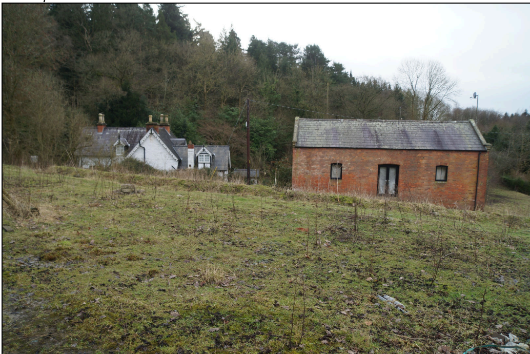
Plate 18: From the southern edge of the development area, looking south. The log cabins would be behind the viewer, Brook House Tank is to the right and Brook House to the left.
