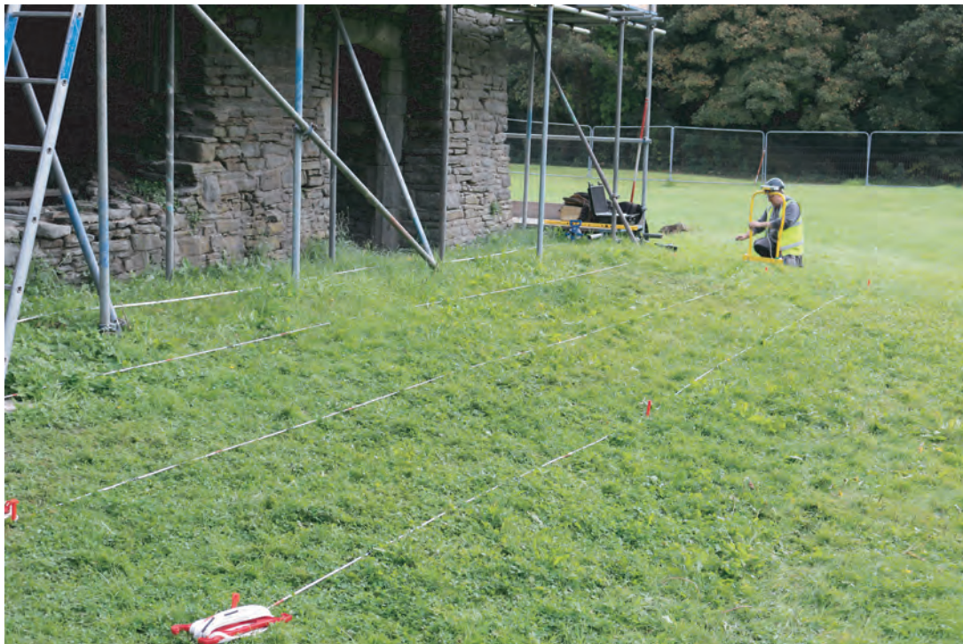
Plate 08. Area 2 - Working shot. Laying out the survey grid and equipment preparation. Looking eastward.
