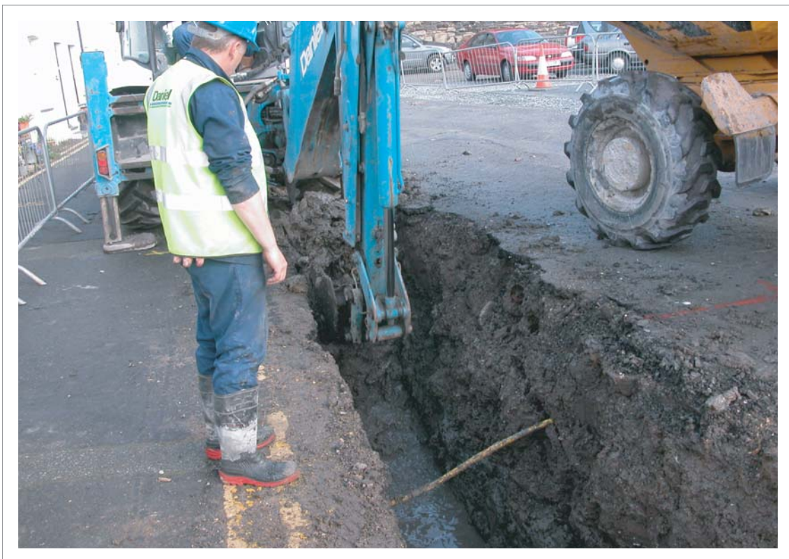
Plate 2: Conwy Quay works
