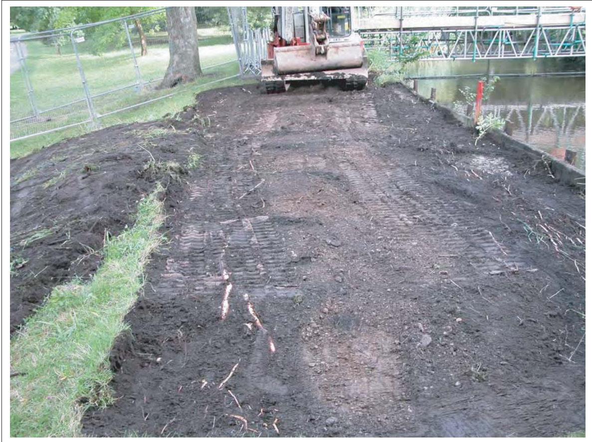
Plate 1: Excavated area, Bute Park Bridge, facing west. Width 3.5m, Length 13.5m
