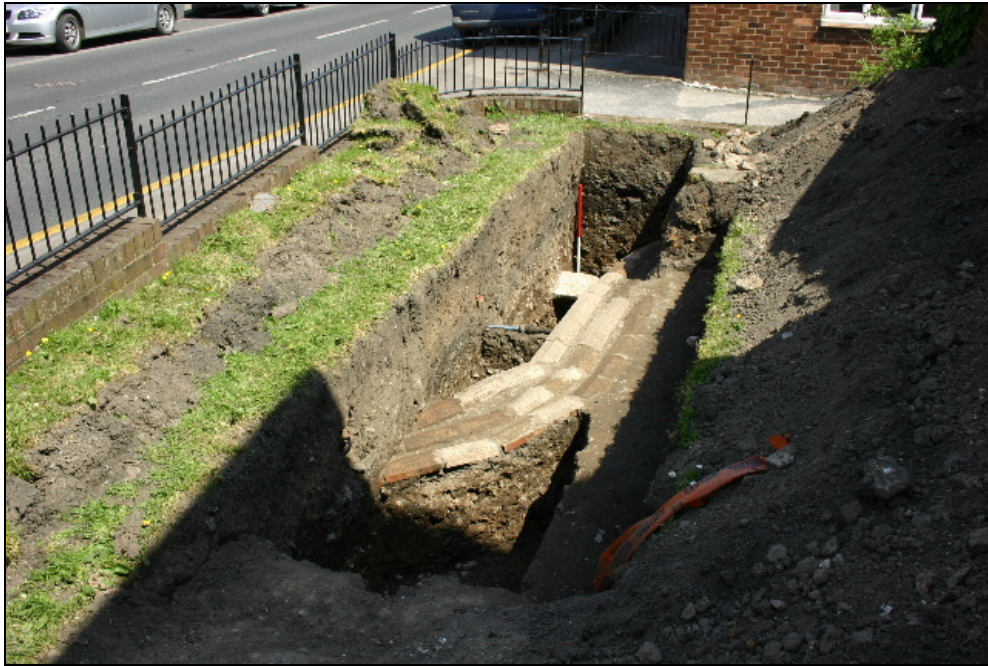
Fig. 11. Trench 2, viewed from the south-west. Photo CPAT 3460-0036
