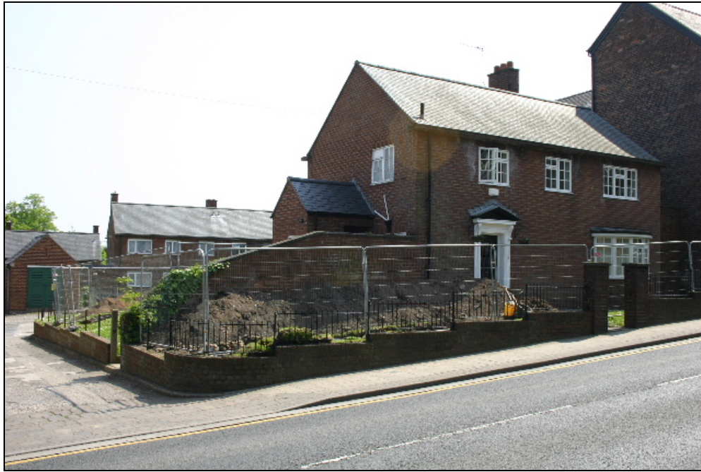
Fig. 2 View of 52 Vale Street. Photo CPAT 3460-0019
