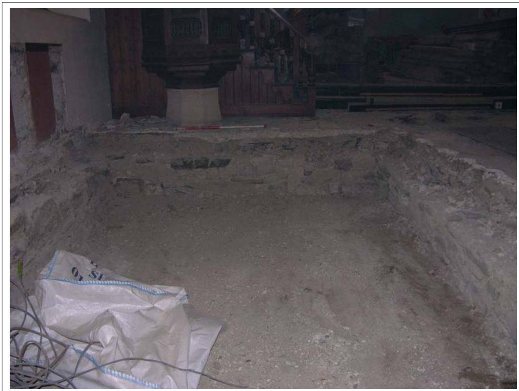
Plate 5: View of exposed foundation masonry below pulpit. Scale 1x1m
