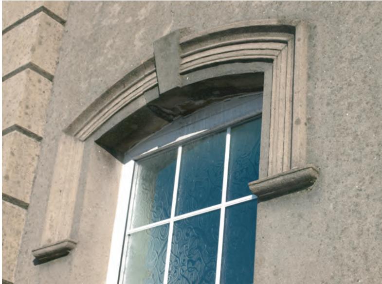
Plate 19. Siloh Chapel (1910). Detail of ground floor window moulding.. Looking north.
