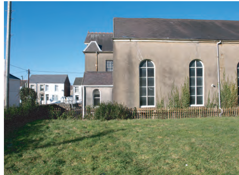
Plate 24. Siloh Chapel (1894). East facing elevation with porch and 1910 chapel in background. Looking westward.
