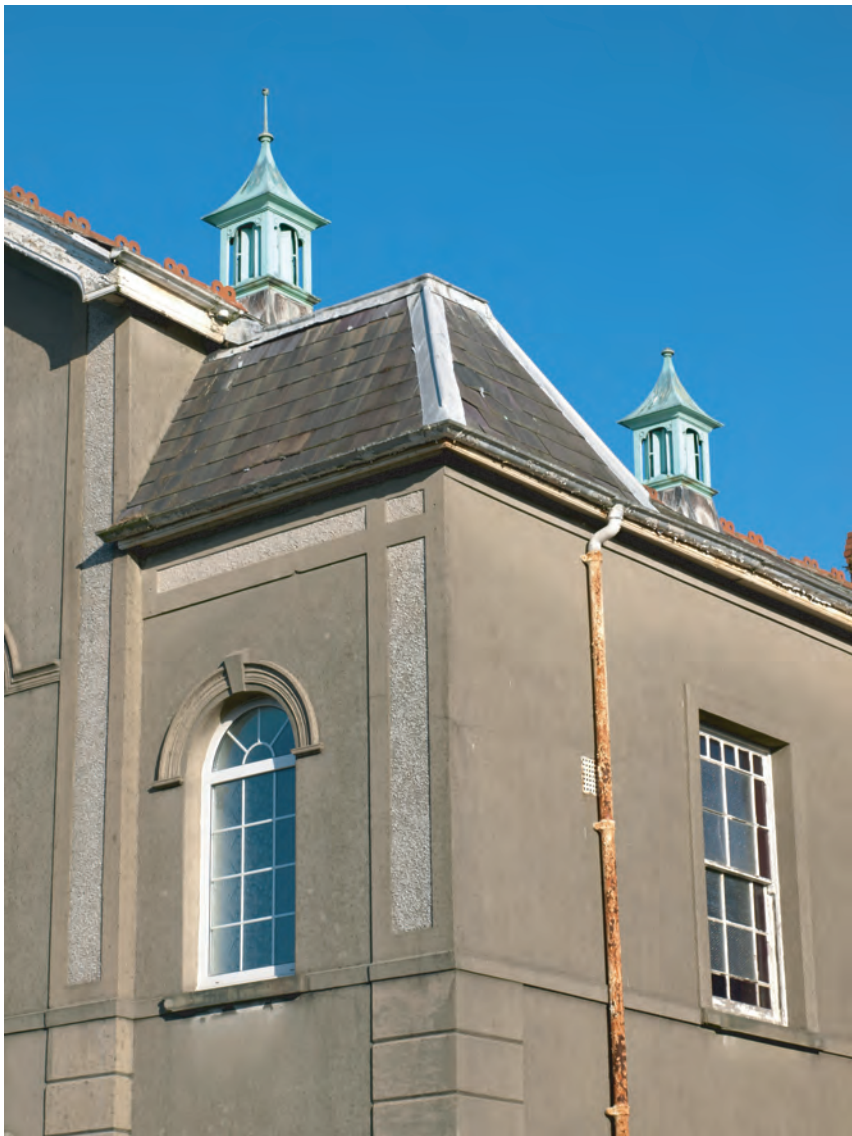
Plate 12. Siloh Chapel (1910). Detail shot of roof features. Looking northwest.
