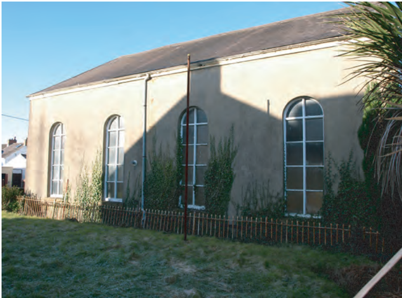
Plate 23. Siloh Chapel (1894). East facing elevation. Looking west.
