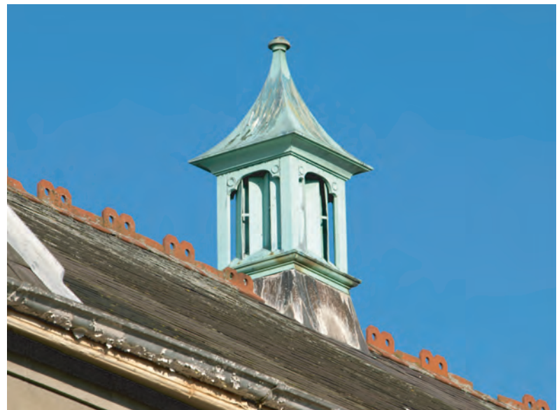
Plate 18. Siloh Chapel (1910). Detail of copper roof air vent cowling. One of two. Looking northwest..
