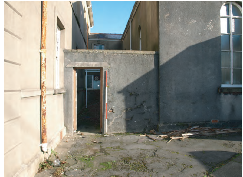
Plate 20. Siloh Chapel (1894 and 1910). Area linking the two chapel together. Looking northwest.
