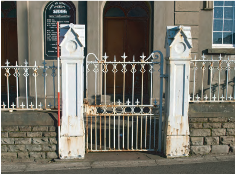
Plate 15. Siloh Chapel (1910). Detail of cast iron gateposts at front of chapel. Looking northeast.
