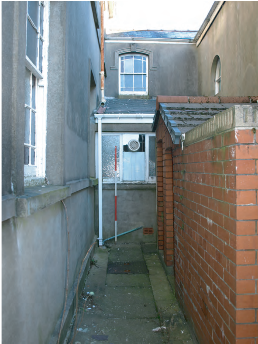
Plate 29. Siloh Chapel (1894). Kitchen at extension elevation. Looking northeast.
