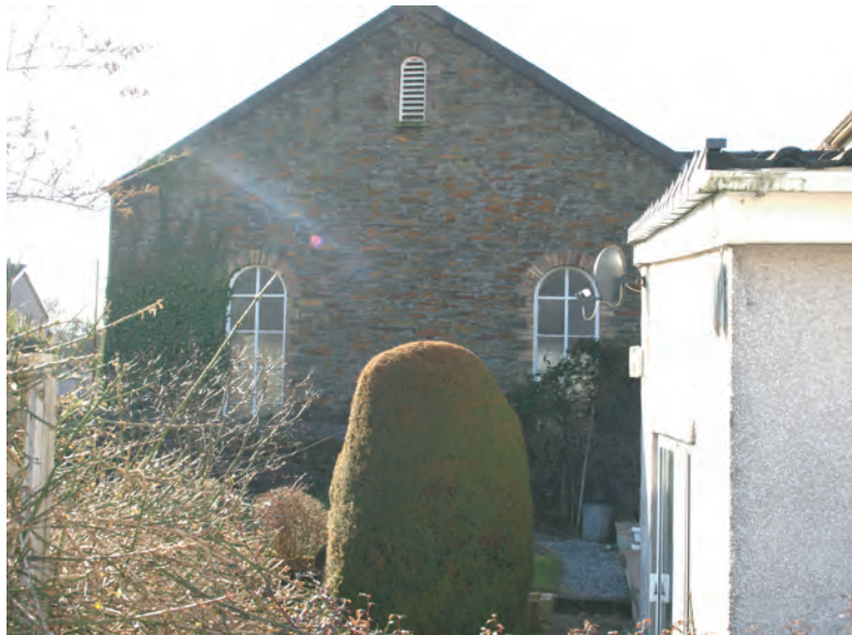
Plate 25. Siloh Chapel (1894). Rear northeast facing elevation Looking southeast.
