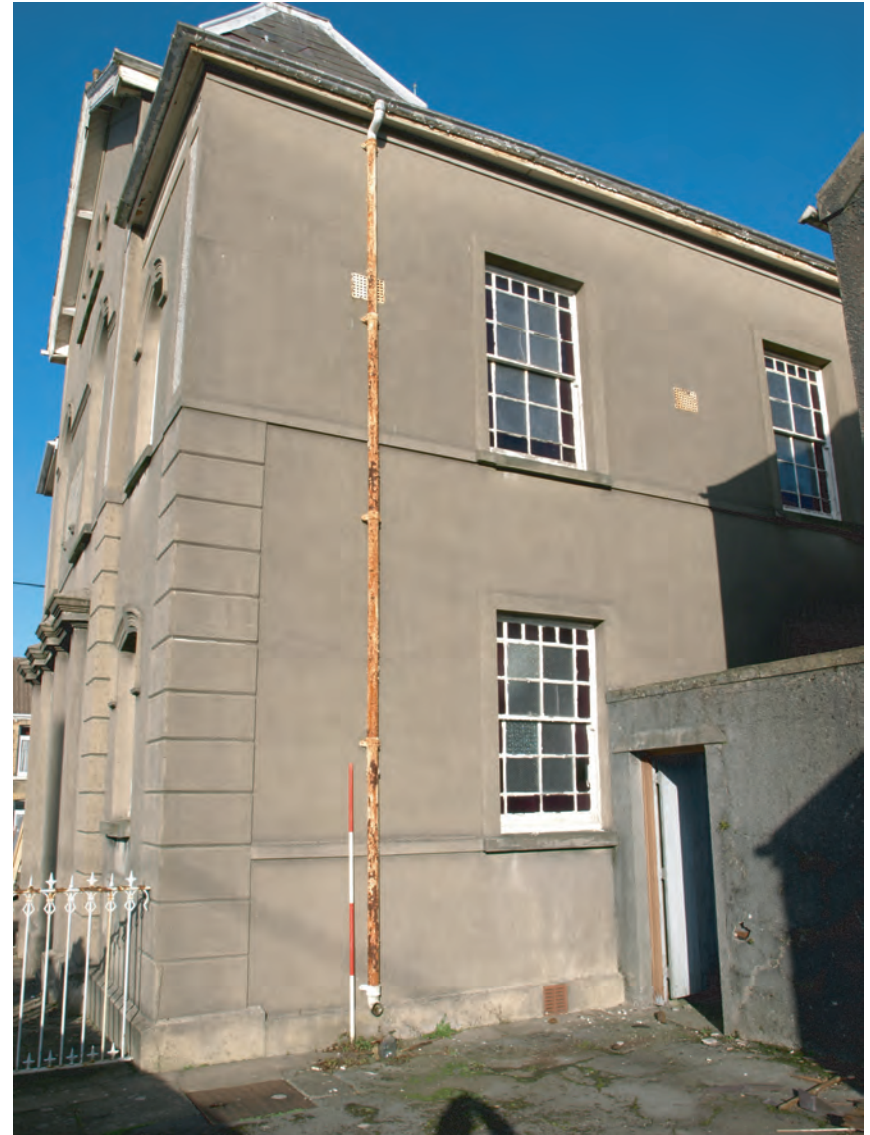
Plate 10. Siloh Chapel (1910). East facing elevation. Looking northwest.
