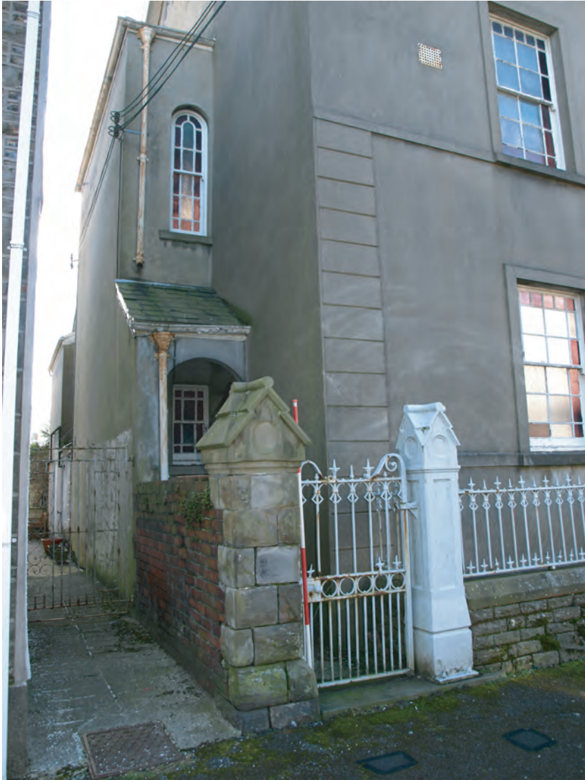
Plate 9. Siloh Chapel (1910). Looking eastward.
