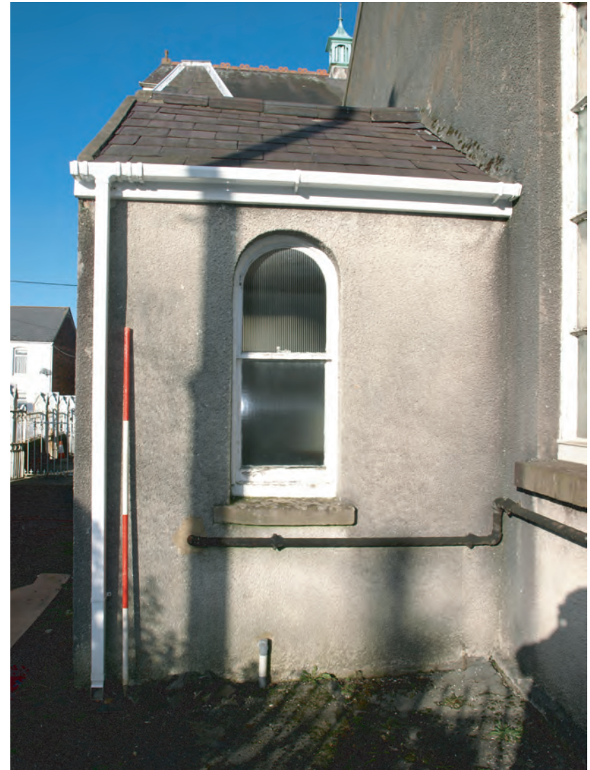
Plate 28. Siloh Chapel (1894). Detail of porch elevation. Looking northwest.
