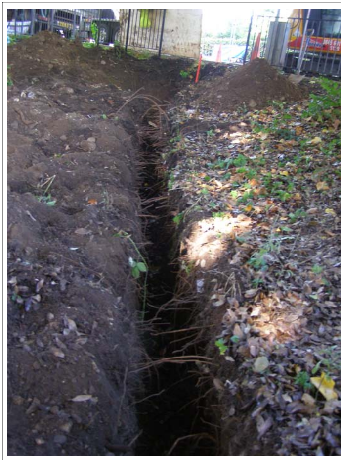
Plate 4: View along trench 3.
