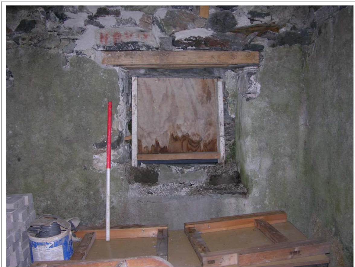
Plate 29: View of blocked window within Building two, Scale 1x1m
