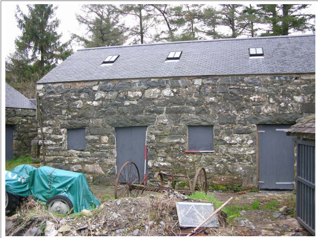
Plate 22: External view of front of Building two, Scales 1x1m & 1x2m
