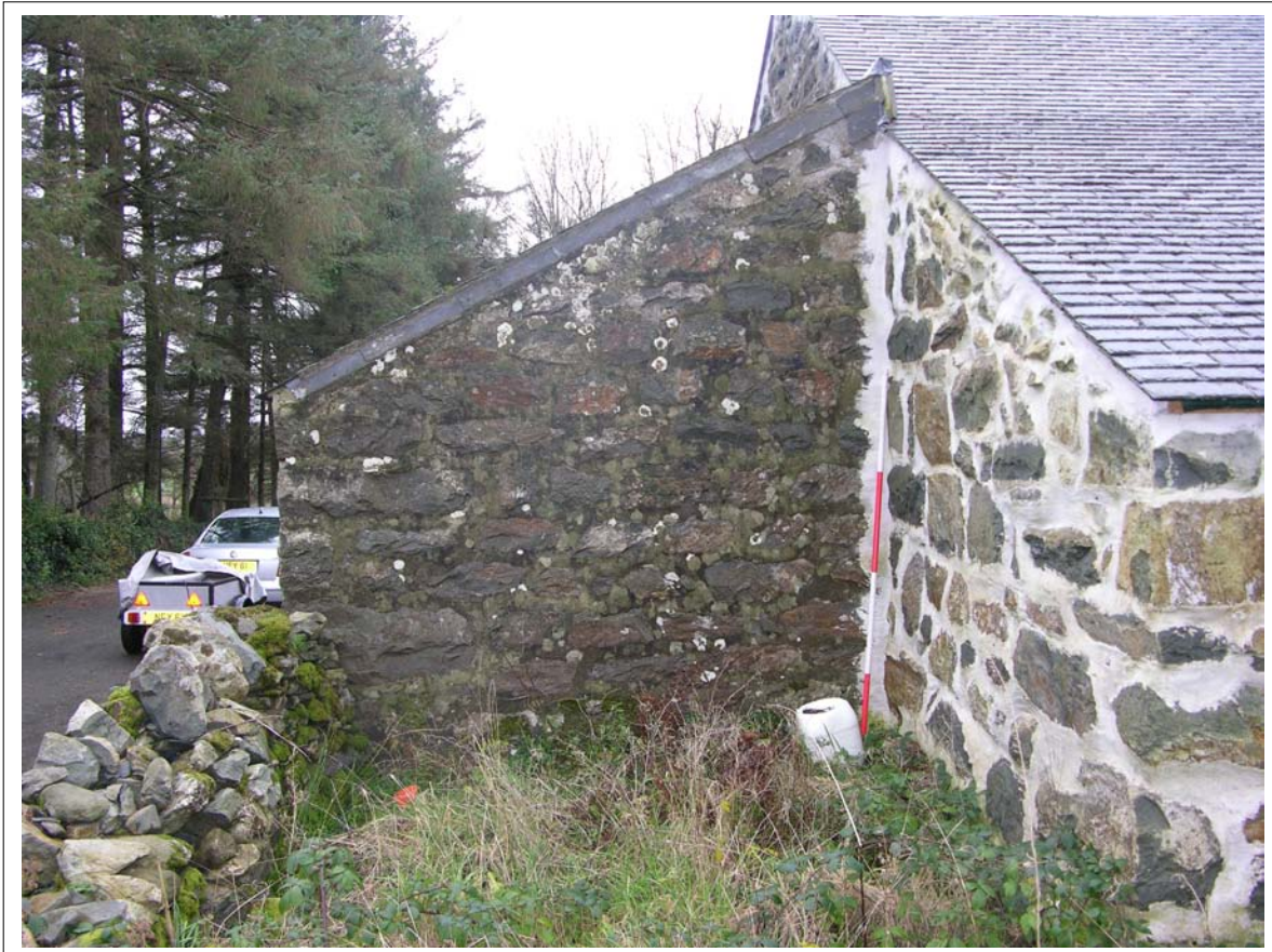
Plate 19: View of butt joint between both additional structures, Scale 1x2m
