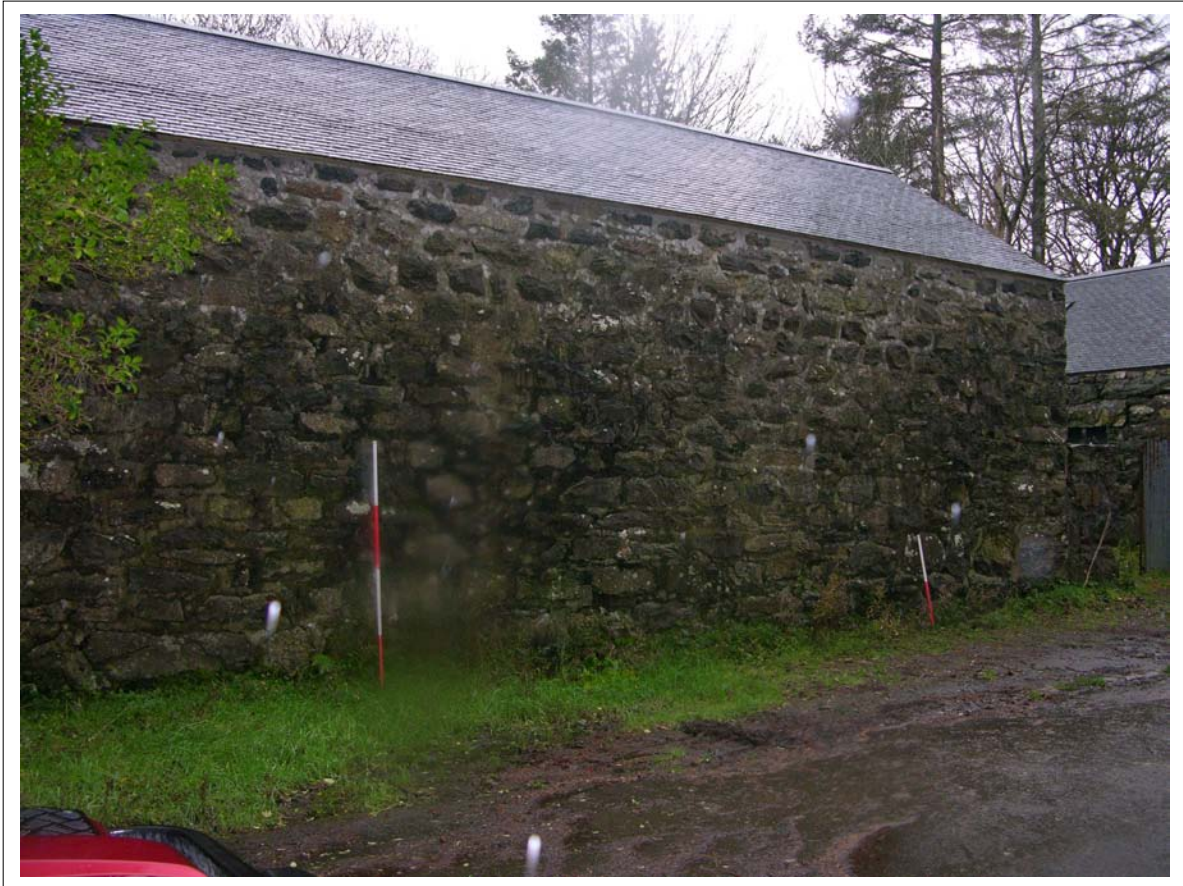
Plate 36: External view of Building two, Scales 1x2m & 1x1m
