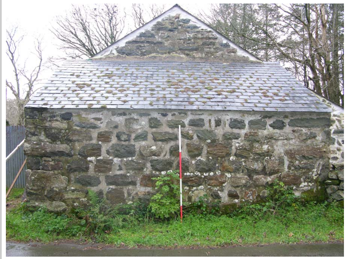
Plate 18: External view of further additional structure, Scale 1x2m
