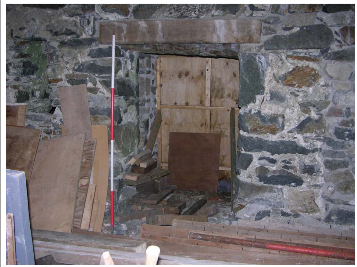
Plate 6: View of internal doorway through to additional structure, Scale 1x2m
