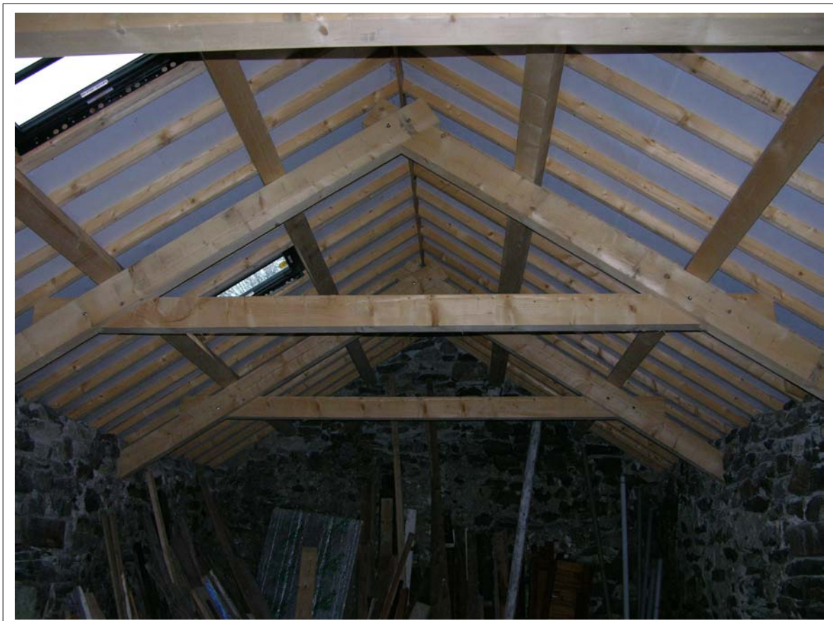
Plate 9: View of relatively new roof from within Building one
