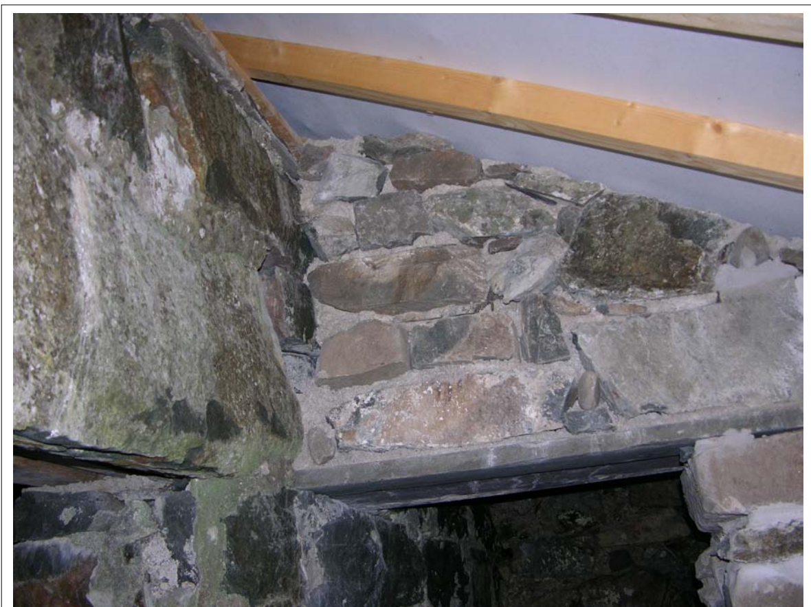
Plate 13: View of butt joint between Building one and additional structure
