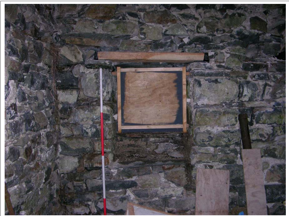
Plate 33: View of blocked window within Building two, Scale 1x2m
