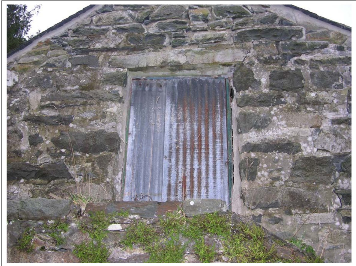
Plate 26: View of doorway at top of external stairs, Building two
