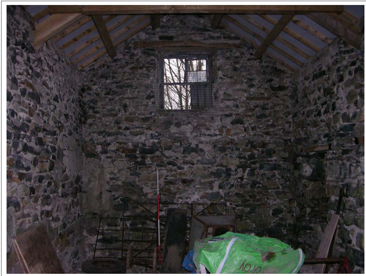
Plate 28: Internal view of Building two, Scale 1x2m
