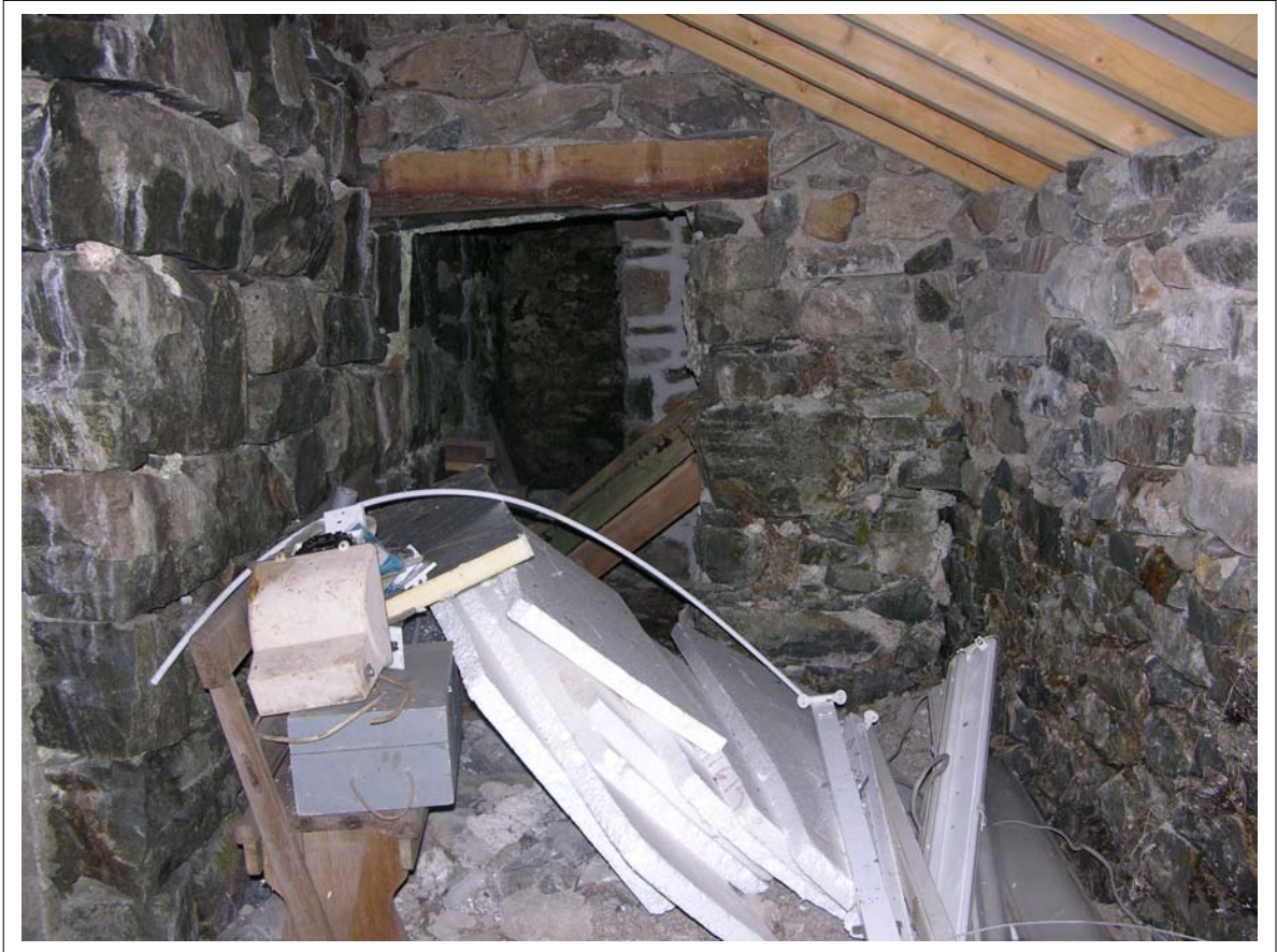
Plate 14: Internal view along additional structure, Building one
