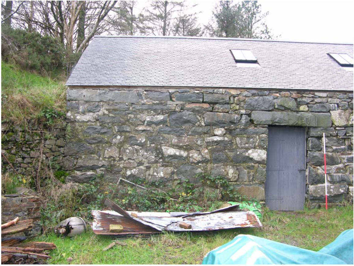
Plate 16: External view of Building one showing where the structure butts against the motte, Scale 1x2m
