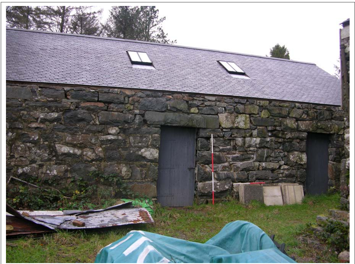
Plate 15: External view of main entrance into Building one, Scales 1x2m & 1x1m
