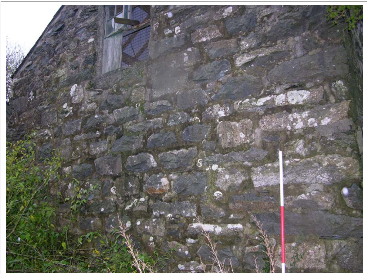
Plate 37: External view of end wall of Building two
