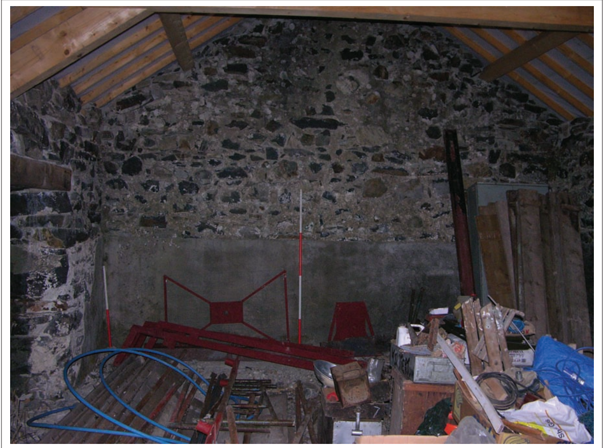
Plate 4: Internal view of Building one, Scale 1x1m & 1x2m
