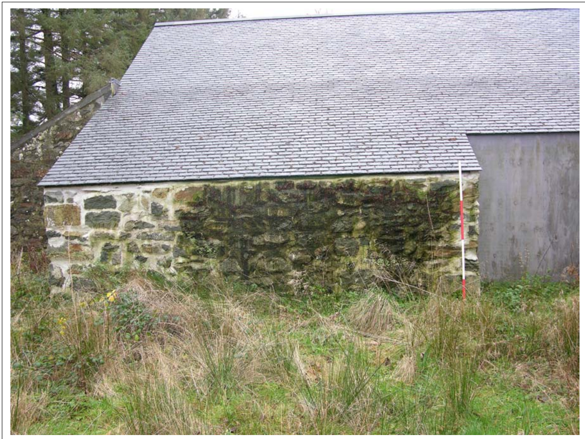
Plate 20: External view of rear of additional structure, Building one, Scale 1x2m
