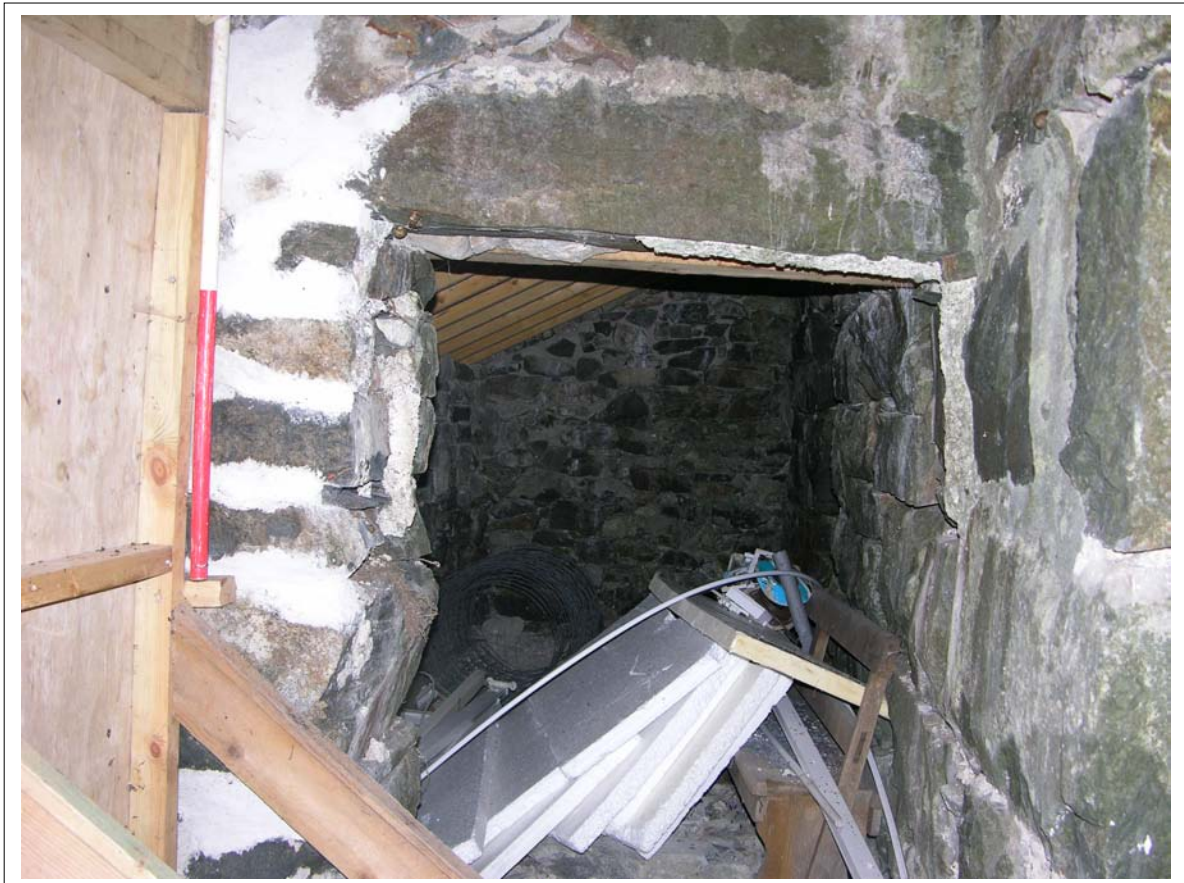
Plate 11: View along added structure in Building one, Scale 1x1m
