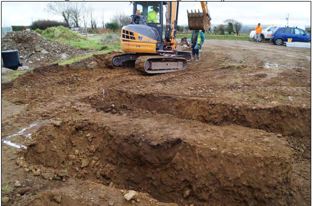
Plate10: HMN2015_110, HMN2015_003, in section after excavation of wall foundations, looking south southeast
