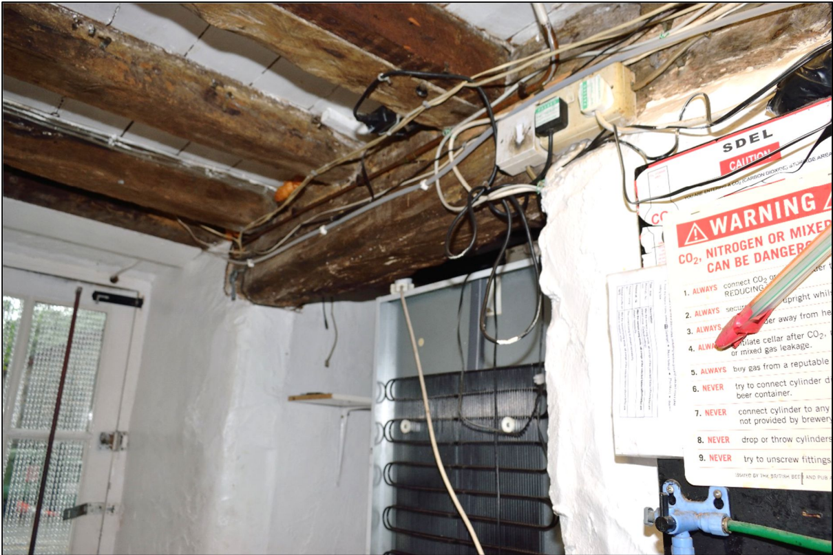
Plate 31: Beam and joists on the eastern side of the passageway
