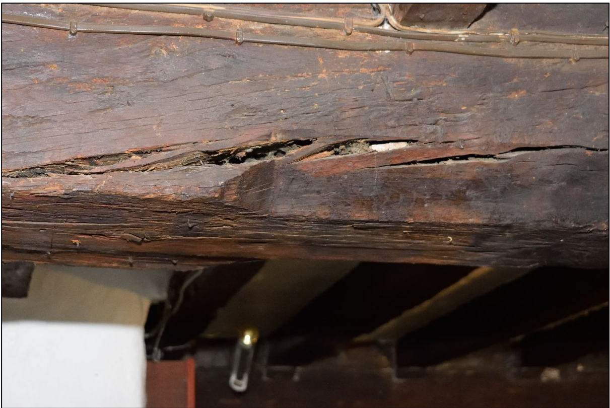
Plate 24: Chamfer and run-out stop on the eastern ceiling beam
