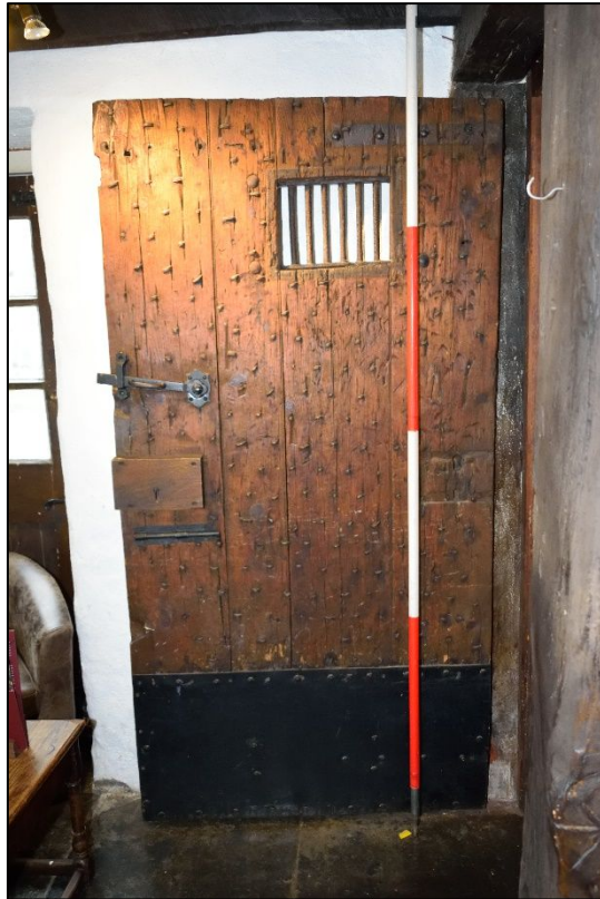
Plate 29: Door at the base of the staircase
