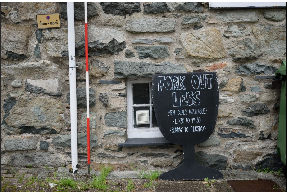
Plate 8: Ground floor window in the southern elevation
