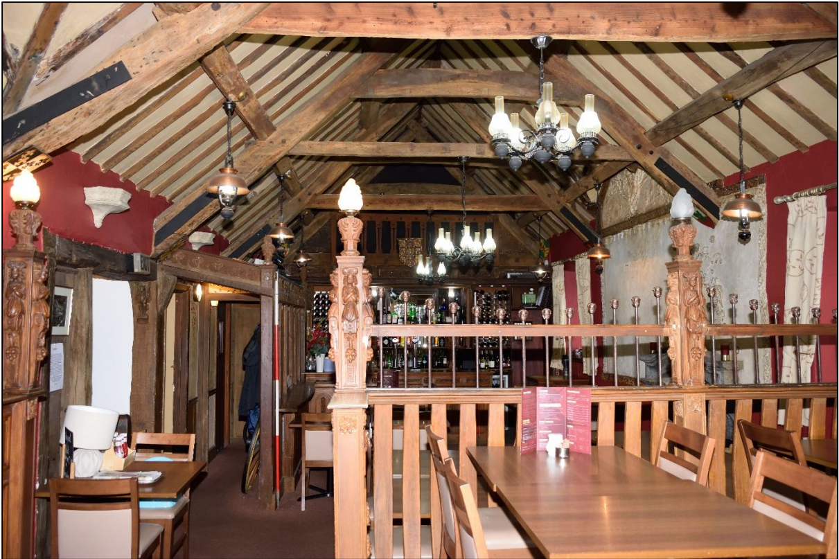
Plate 33: First-floor restaurant, looking west
