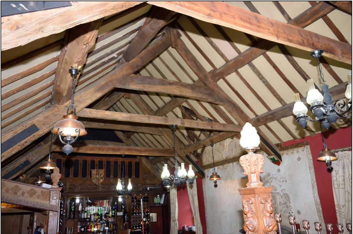
Plate 37: Truss 2, looking west
