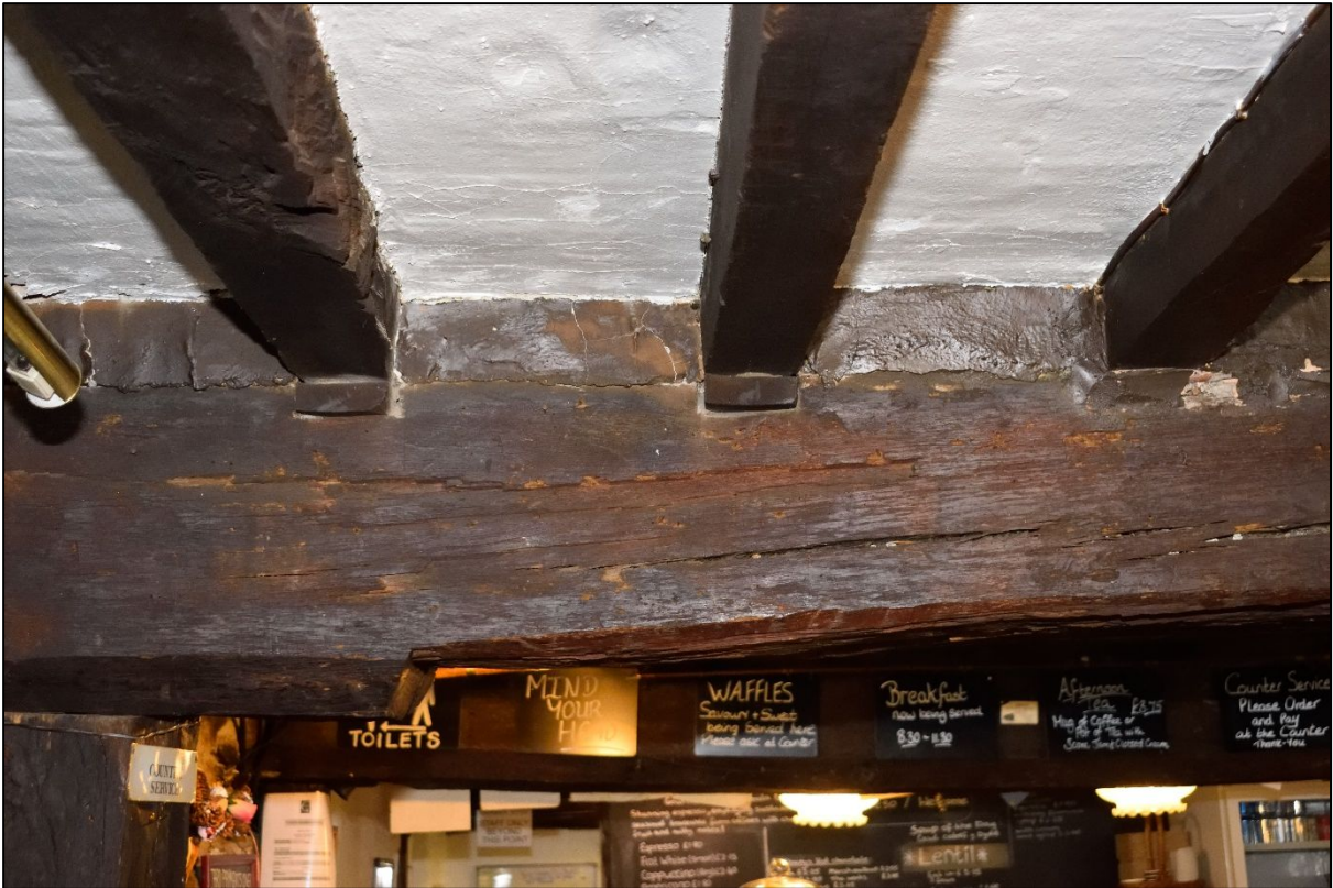
Plate 25: Cogged joists
