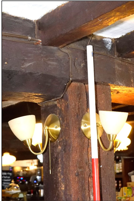
Plate 23: Chamfer on one of the ceiling beams
