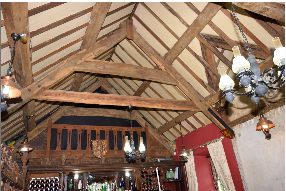
Plate 38: Truss 3, looking west
