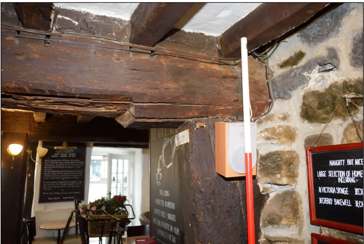
Plate 22: Chamfer on one of the ceiling beams
