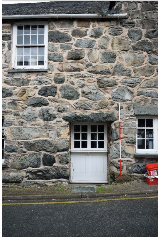
Plate 17: Partially blocked doorway and window above
