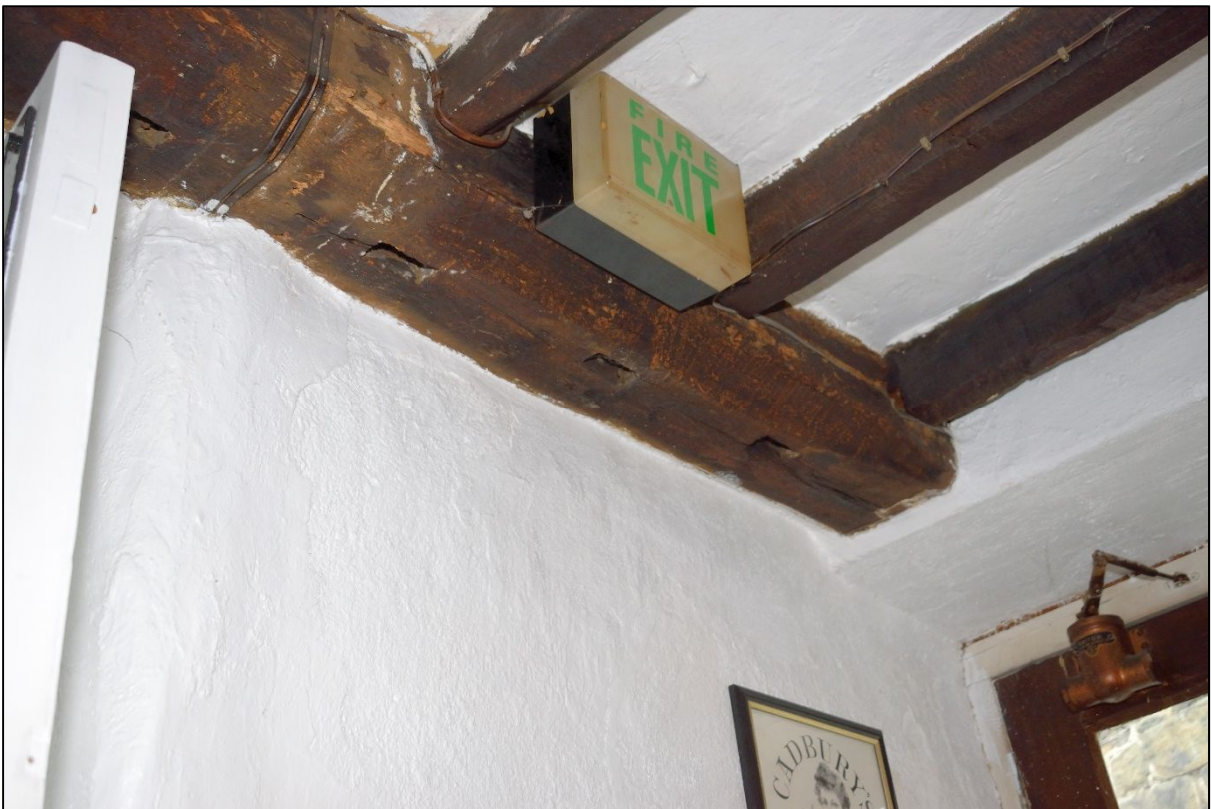
Plate 26: Re-used timber in south eastern corner of the tearoom
