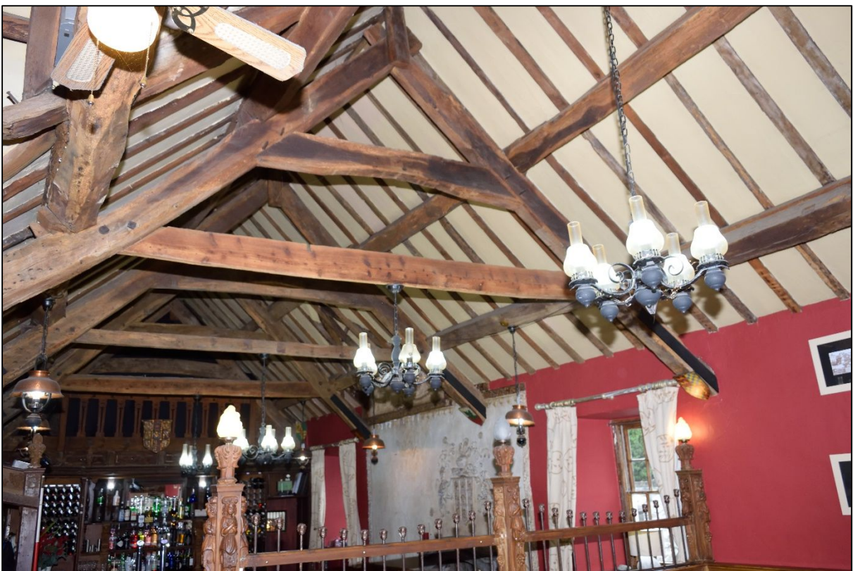
Plate 36: Truss 1, looking west
