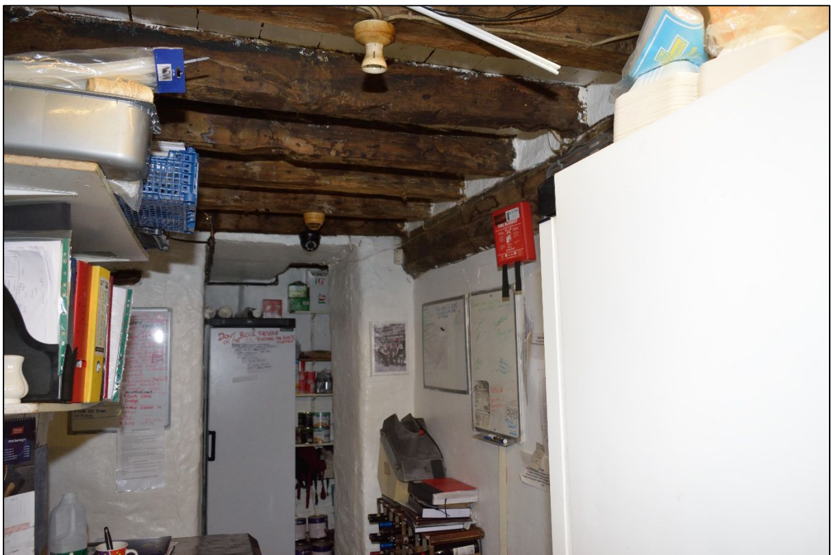
Plate 30: Passageway, looking south
