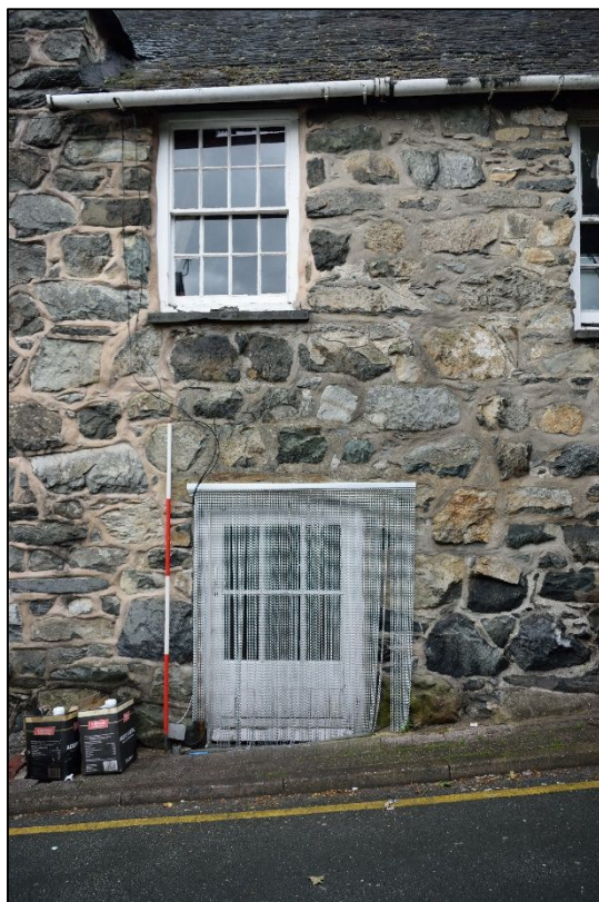
Plate 16: Door and window above in the northern elevation
