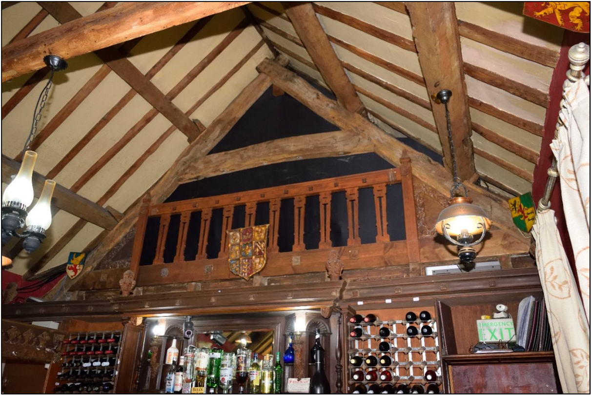
Plate 39: Truss 4, looking south west
