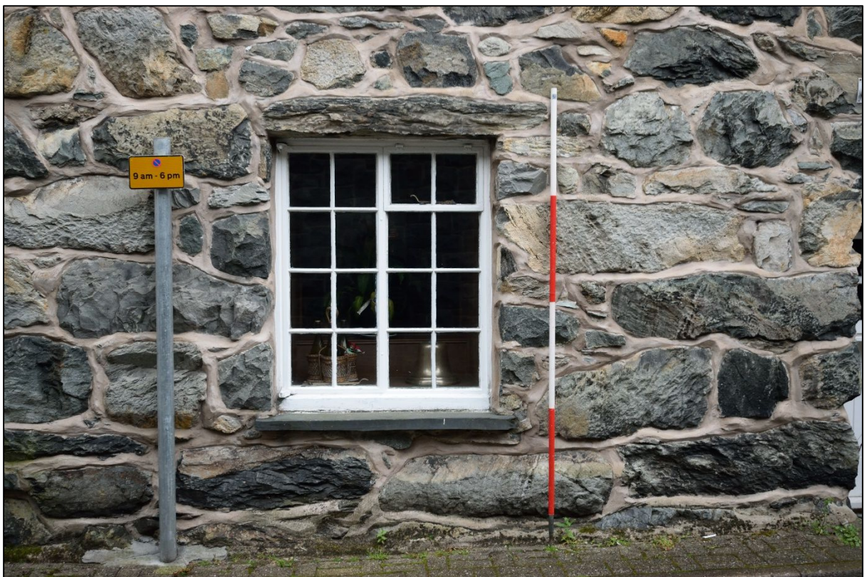
Plate 18: Eastern window in the northern elevation
