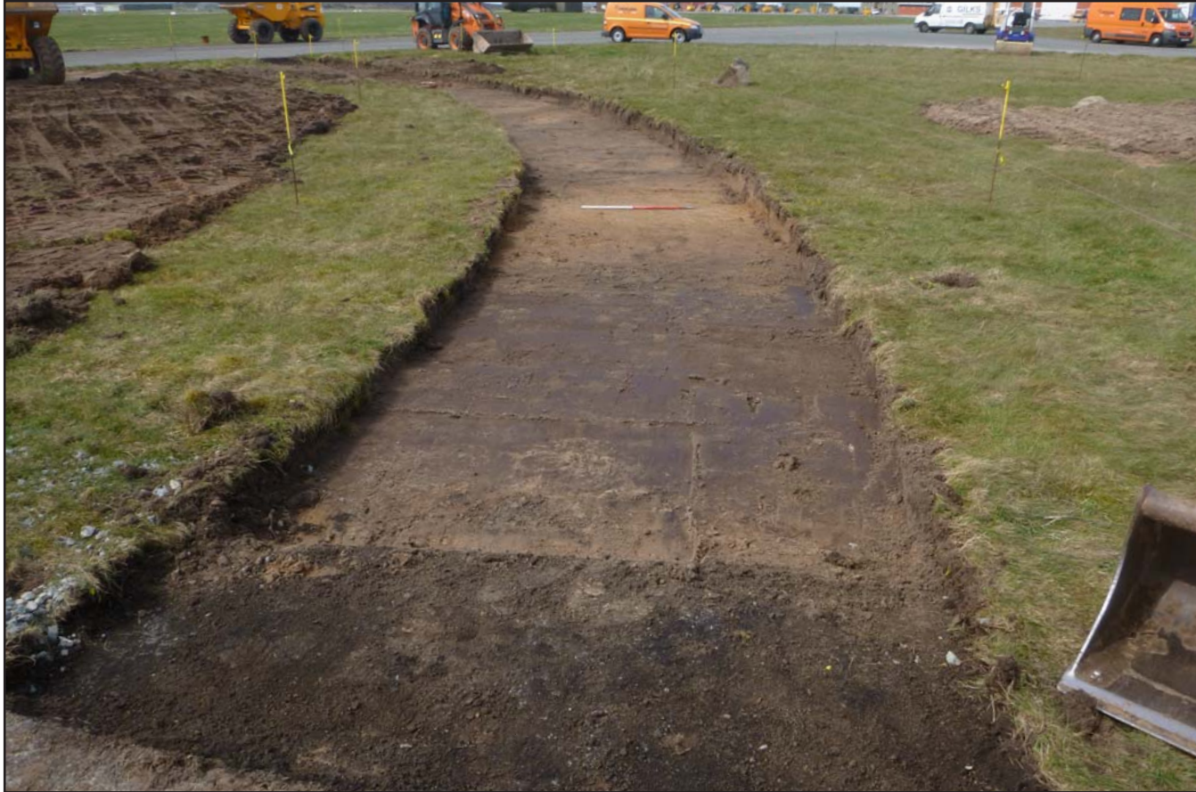
Plate 21: CCB strip excavation (north eastern quadrant) - from the southwest - 1m scale
