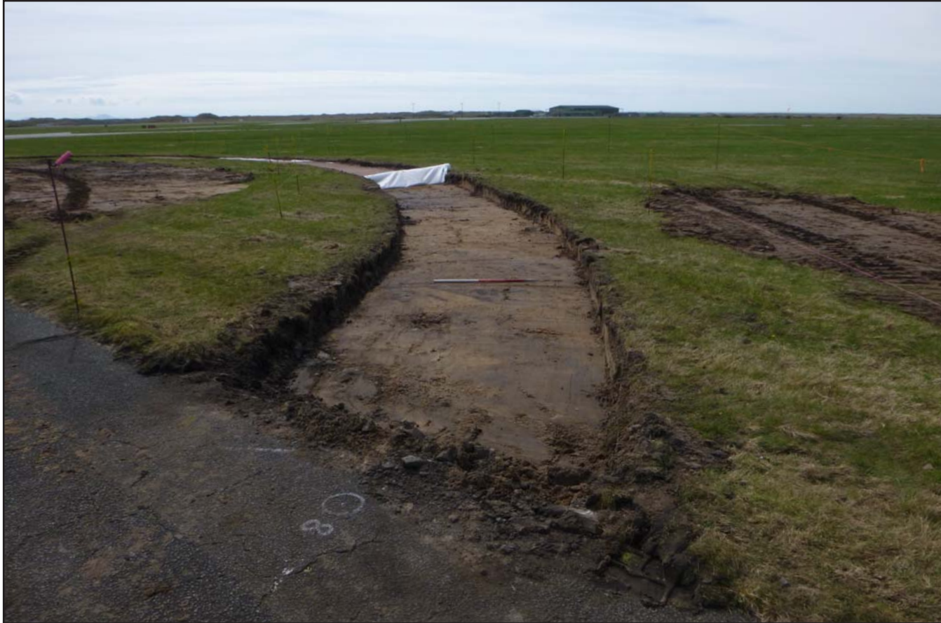
Plate 19: CCB strip excavation (north western quadrant) - from the northeast - 1m scale
