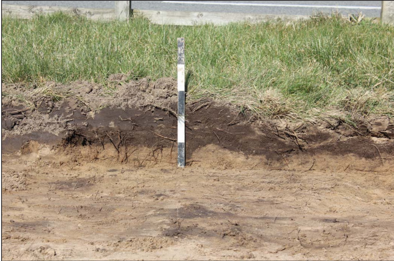
Plate 34: Section of perimeter road (at 100.0m) - from the south - 0.50m scale
