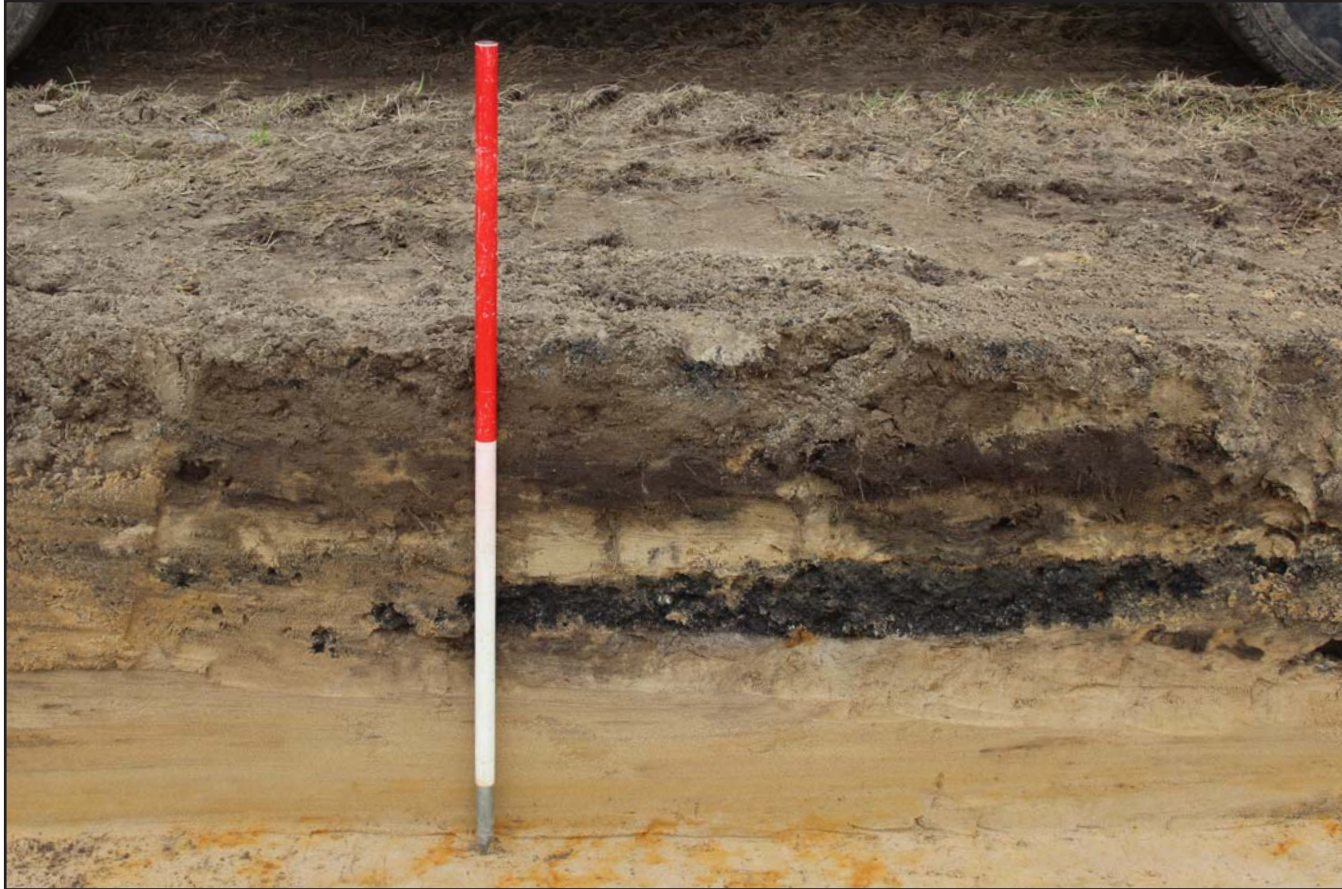
Plate 37: Section of perimeter road (at 550.0m) - from the northeast - 1m scale
