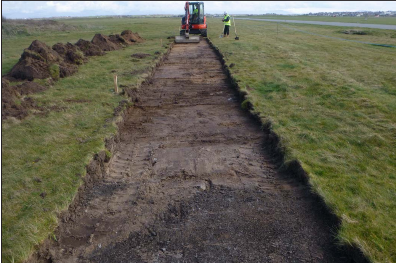
Plate 02: Area of previous dense vegetation 50.0m-70.0m - from the northwest - no scale
