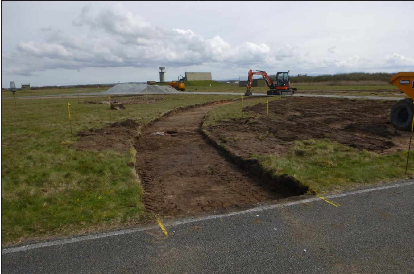
Plate 20: CCB strip excavation (north eastern quadrant) - from the northwest - no scale
