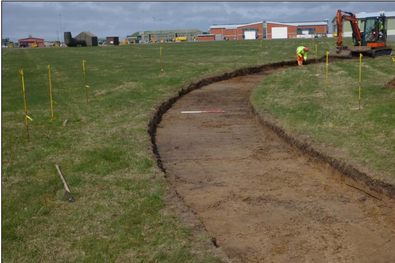
Plate 18: CCB strip excavation (south western quadrant) - from the south - 1m scale
