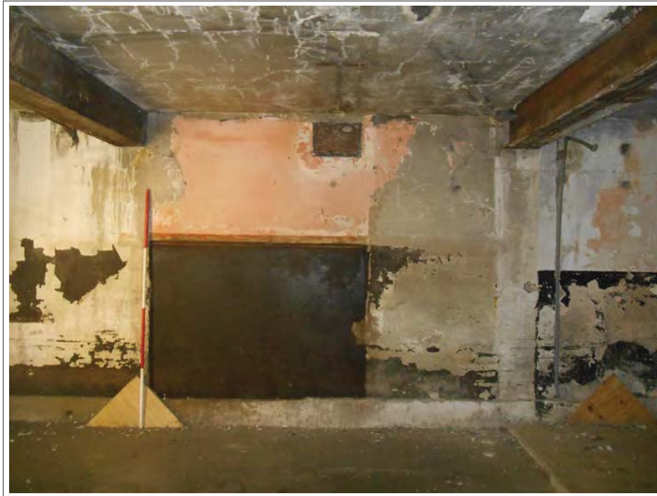
Plate 140. West facing wall with dado rail.
