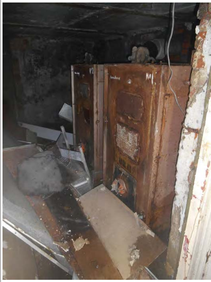
Plate 114. Meter room, looking SSW.
