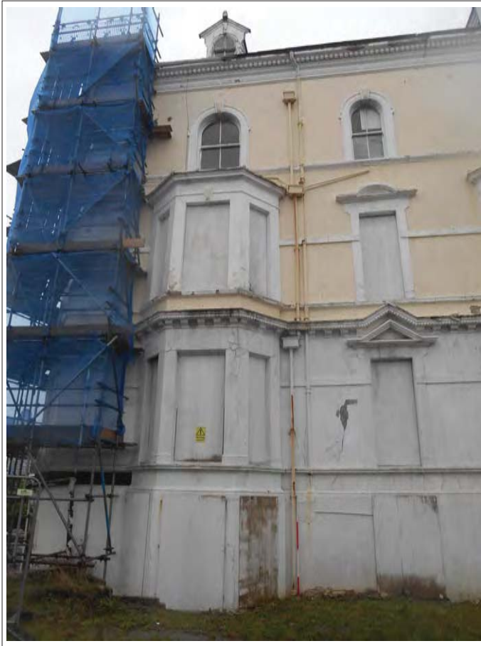
Plate 9. View of eastern elevation, looking NW.
