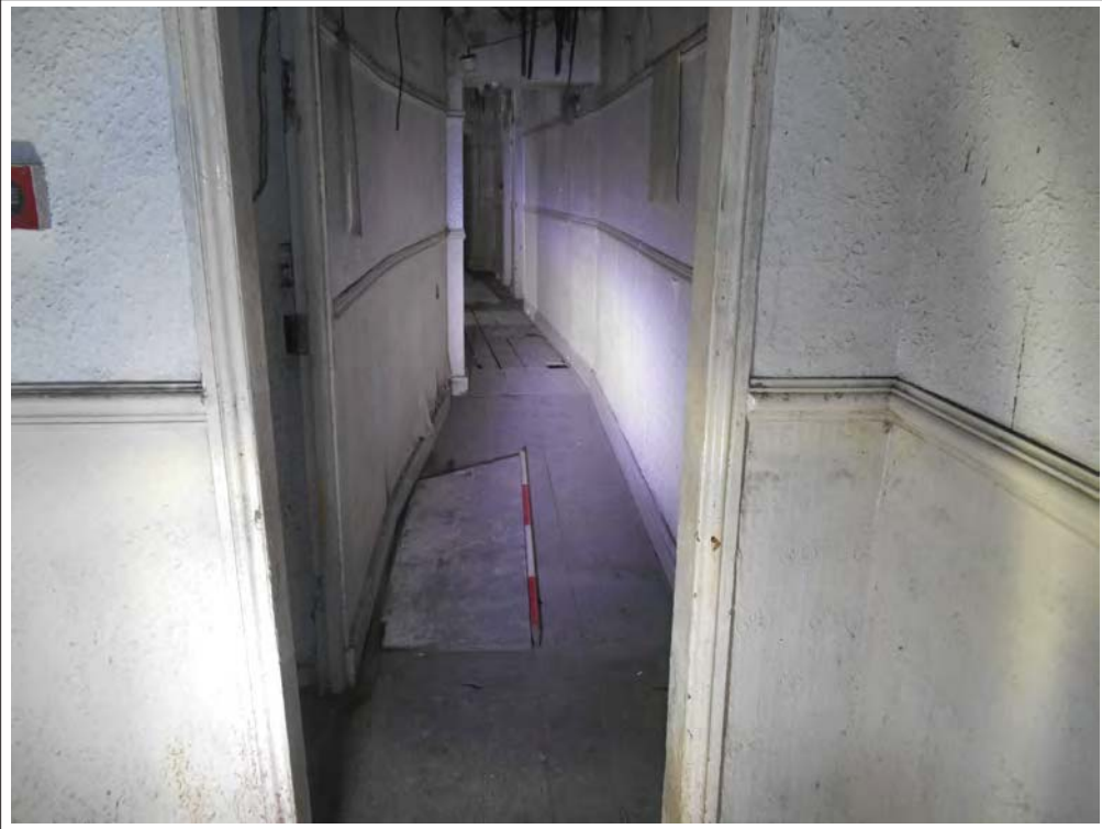
Plate 101. View of corridor looking E.
