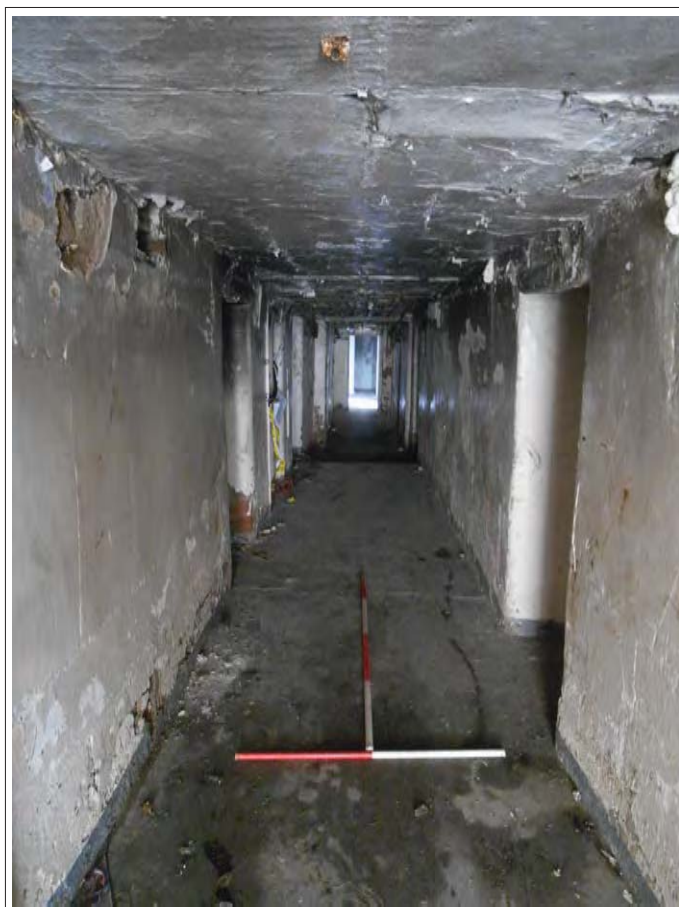
Plate 108. View of basement corridor, looking W.
