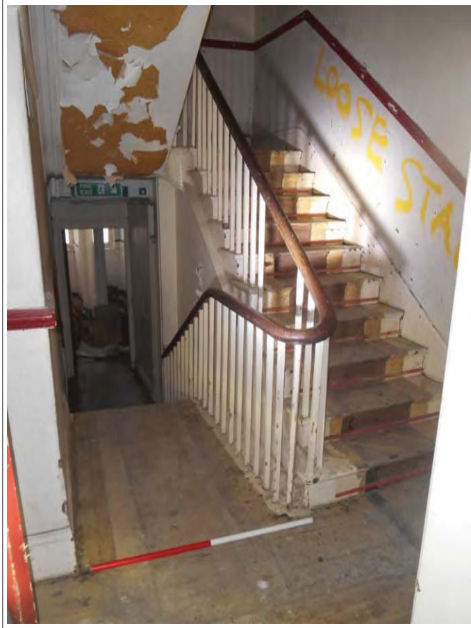
Plate 59. View of staircase, looking E.
