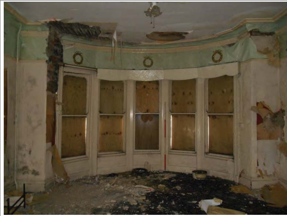
Plate 49. Canted five-light window, looking N.
