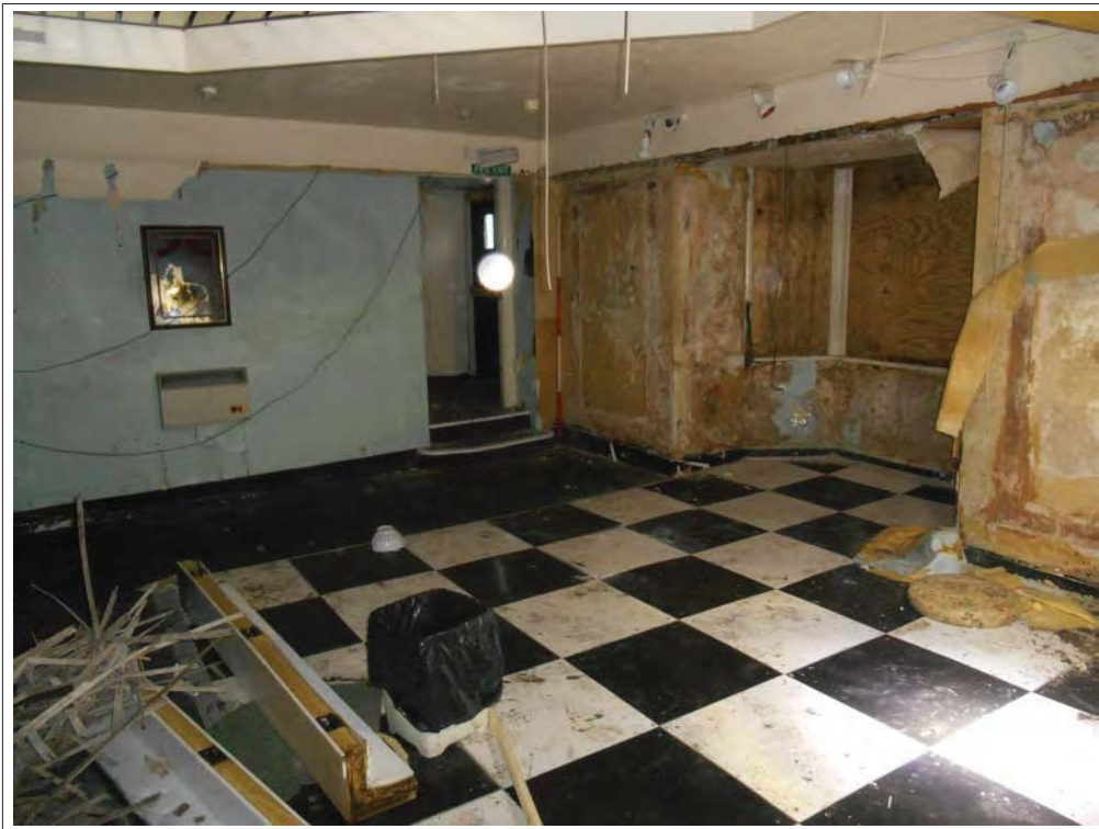
Plate 123. Bar area, looking E.
