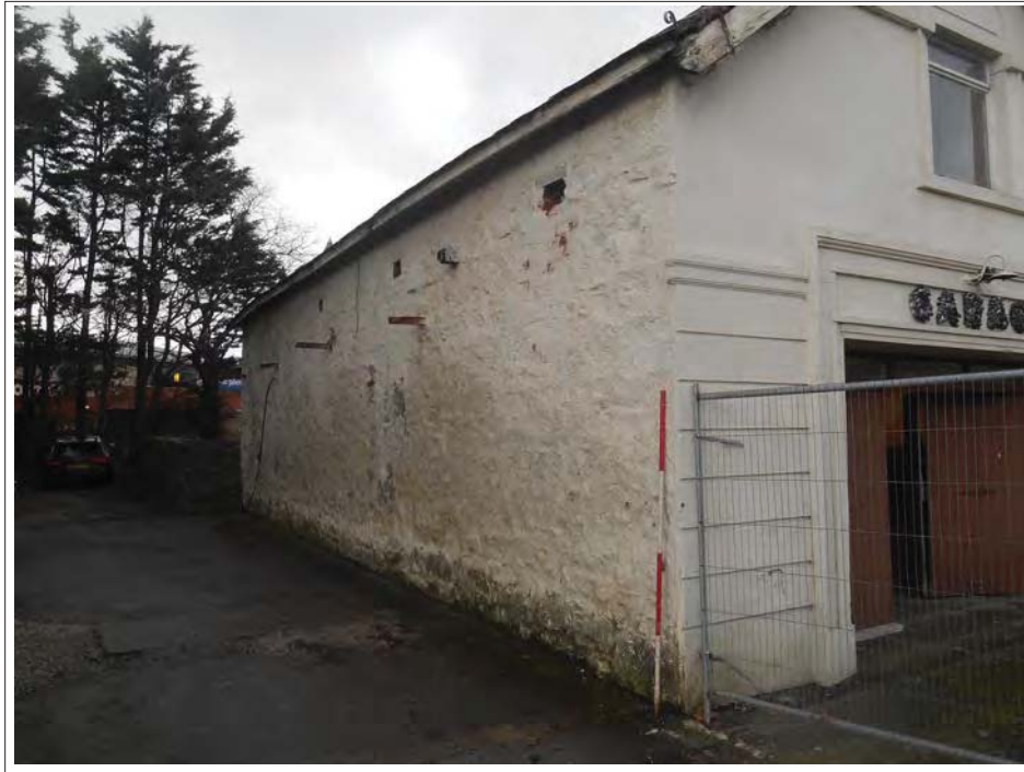
Plate 148. Oblique view of west facing exterior wall with corbels.
