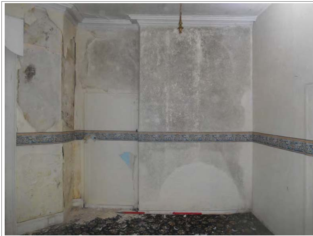
Plate 44. Blocked door predating current wall decoration, looking E.
