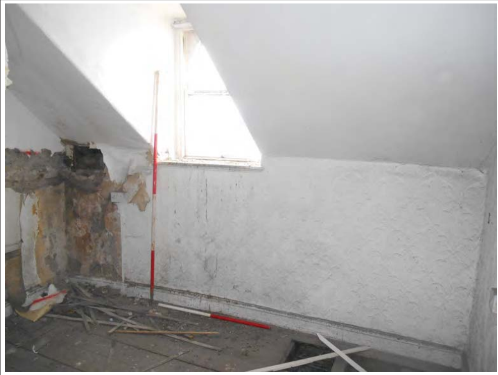
Plate 105. View of attic window, looking W.
