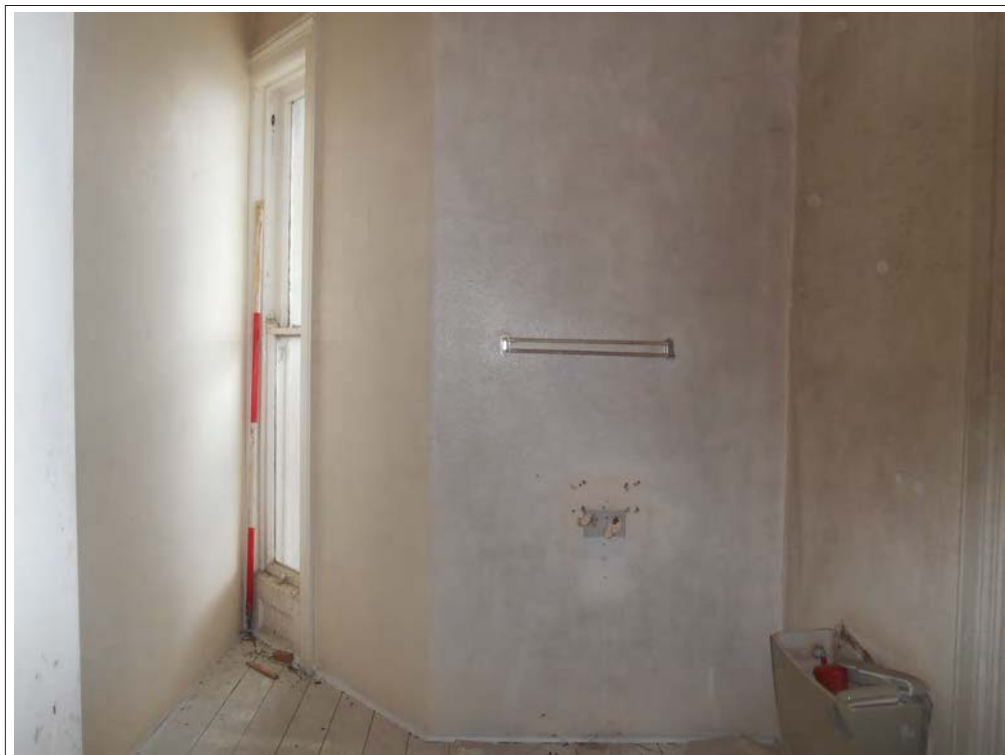
Plate 74. View of Room 7. Ensuite bathroom. Door blocked, looking NE.
