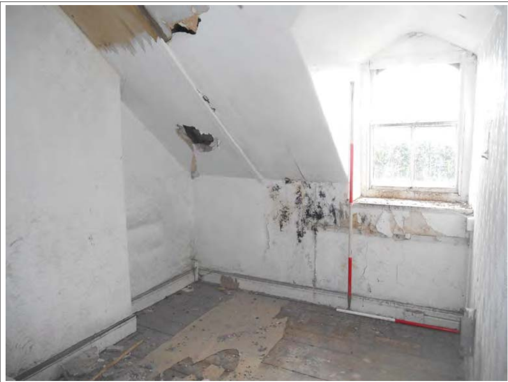
Plate 106. View of attic window, looking W.
