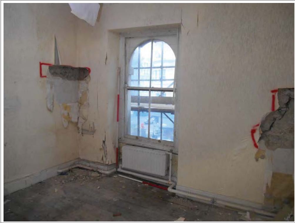
Plate 75. View of Room 11 with rounded head sash window, looking N.
