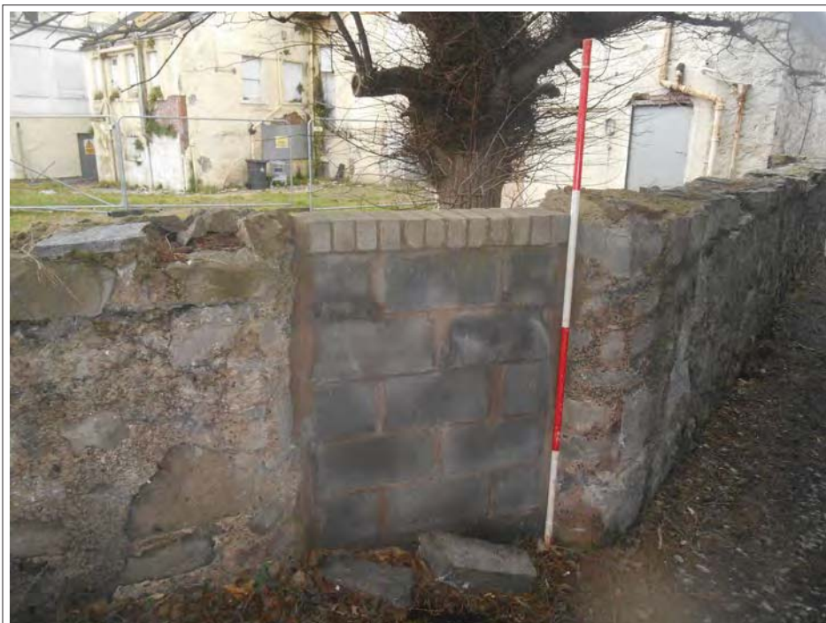
Plate 172. Modern alteration of circuit wall. Scale 2m
