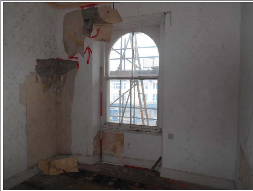
Plate 83. View of Room 2, with round-headed sash window and multiple layers of wall paper, looking SSW
