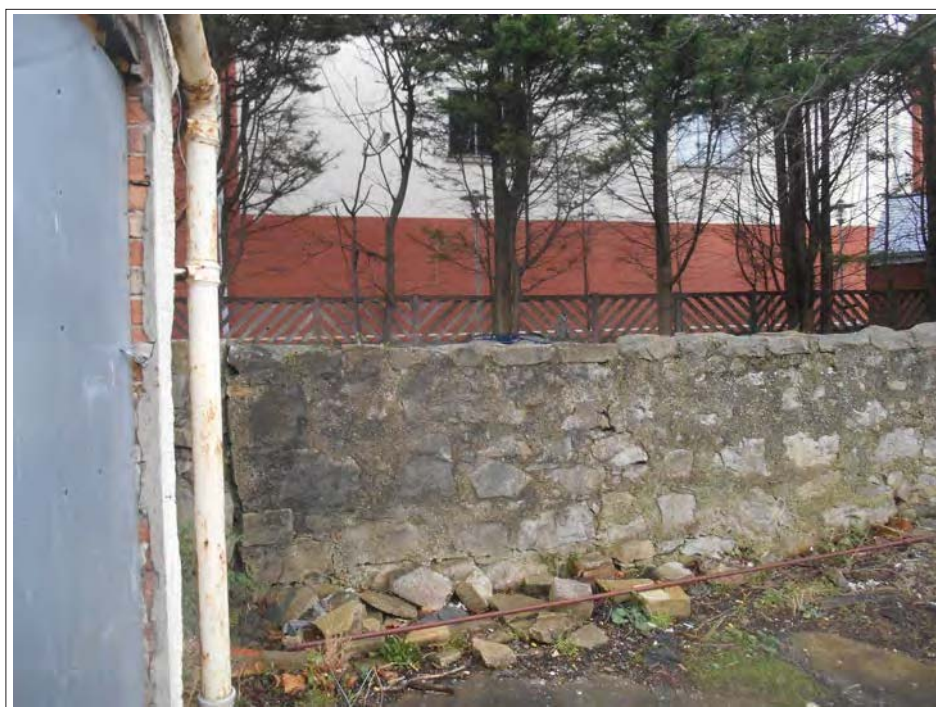
Plate 173. Circuit wall viewed from back entrance.
