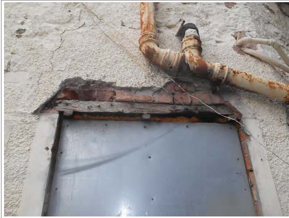
Plate 158. Detail of wooden lintel.
