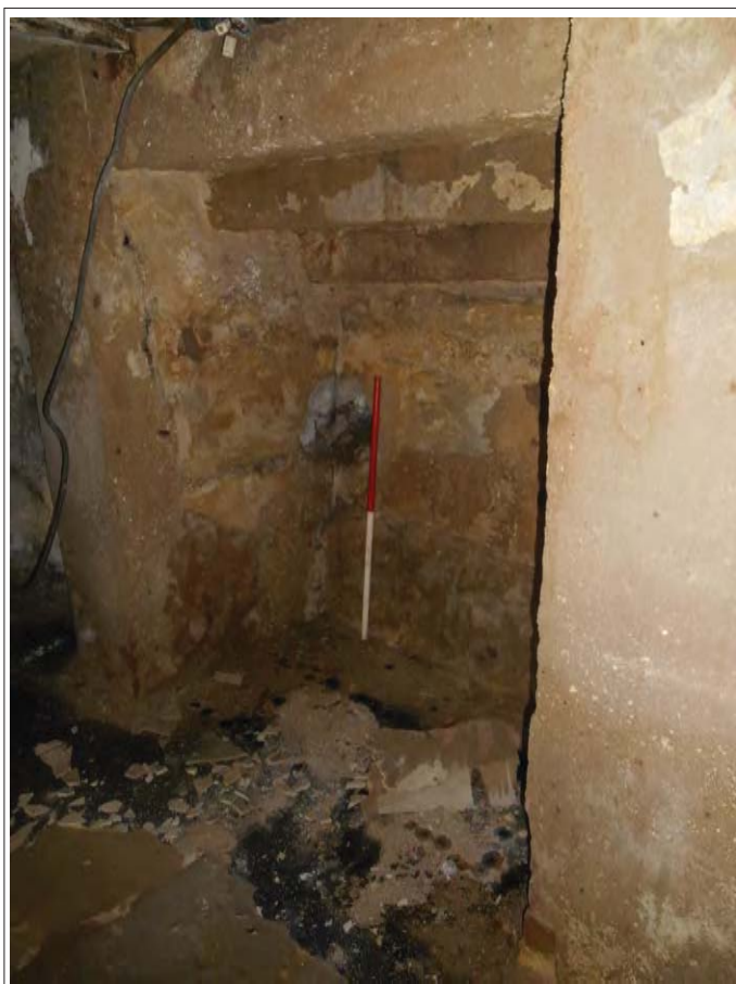
Plate 125. Original construction materials, looking NNE.
