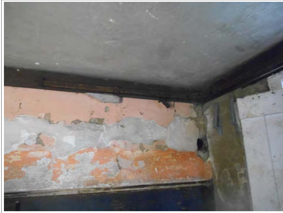
Plate 132. Detail of door track/slide - no longer in use
