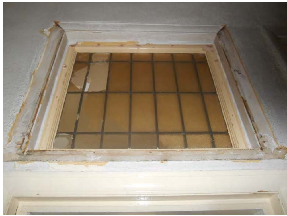
Plate 67. Light box above door. Room 9, looking E .
