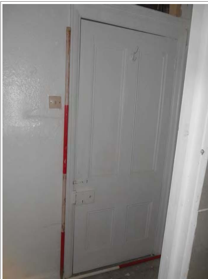
Plate 66. Original door frame. Room 9, looking SW.
