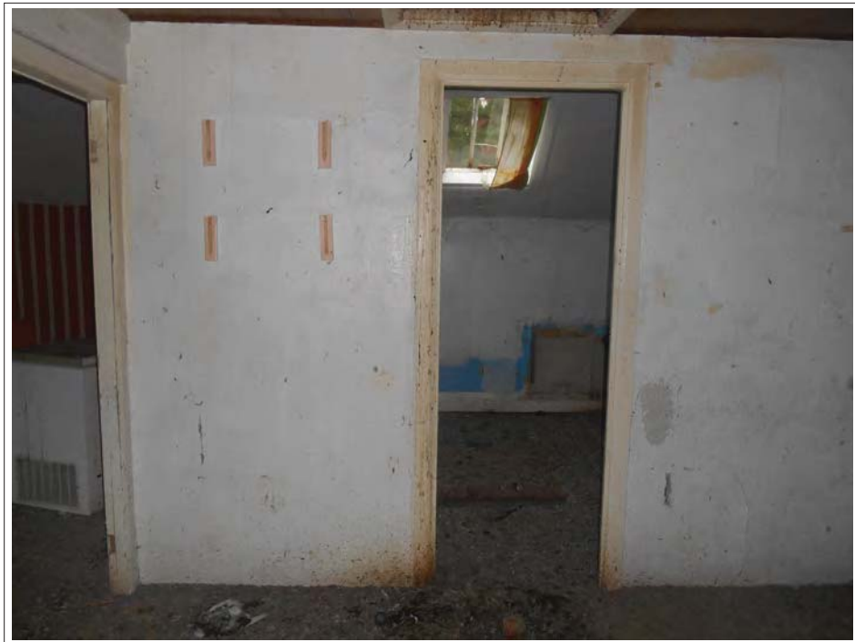
Plate 161. First floor, looking west.
