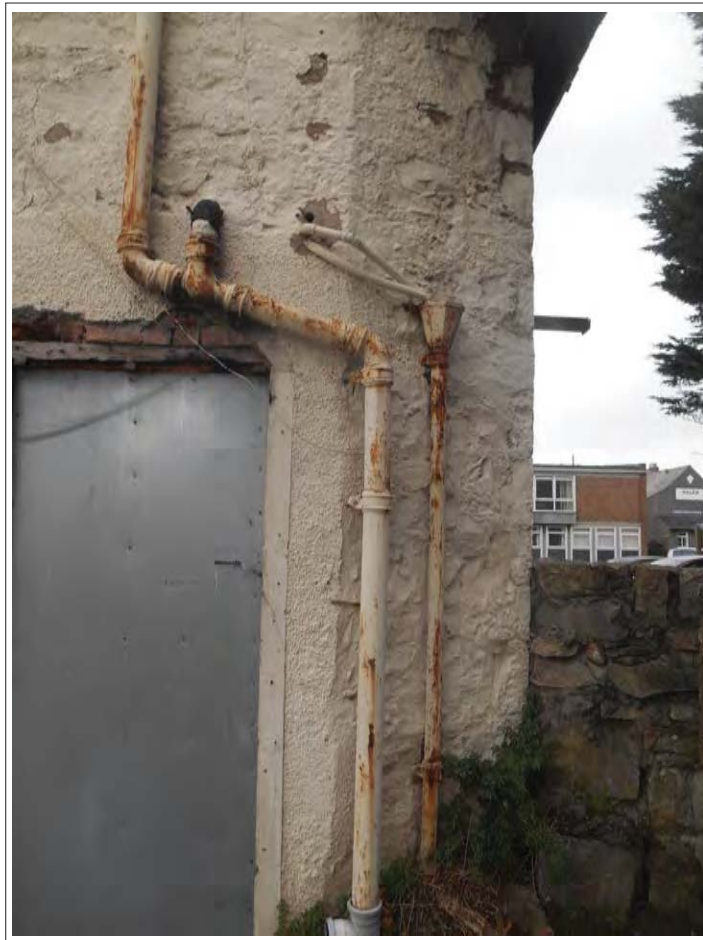
Plate 156. View of cast iron guttering.
