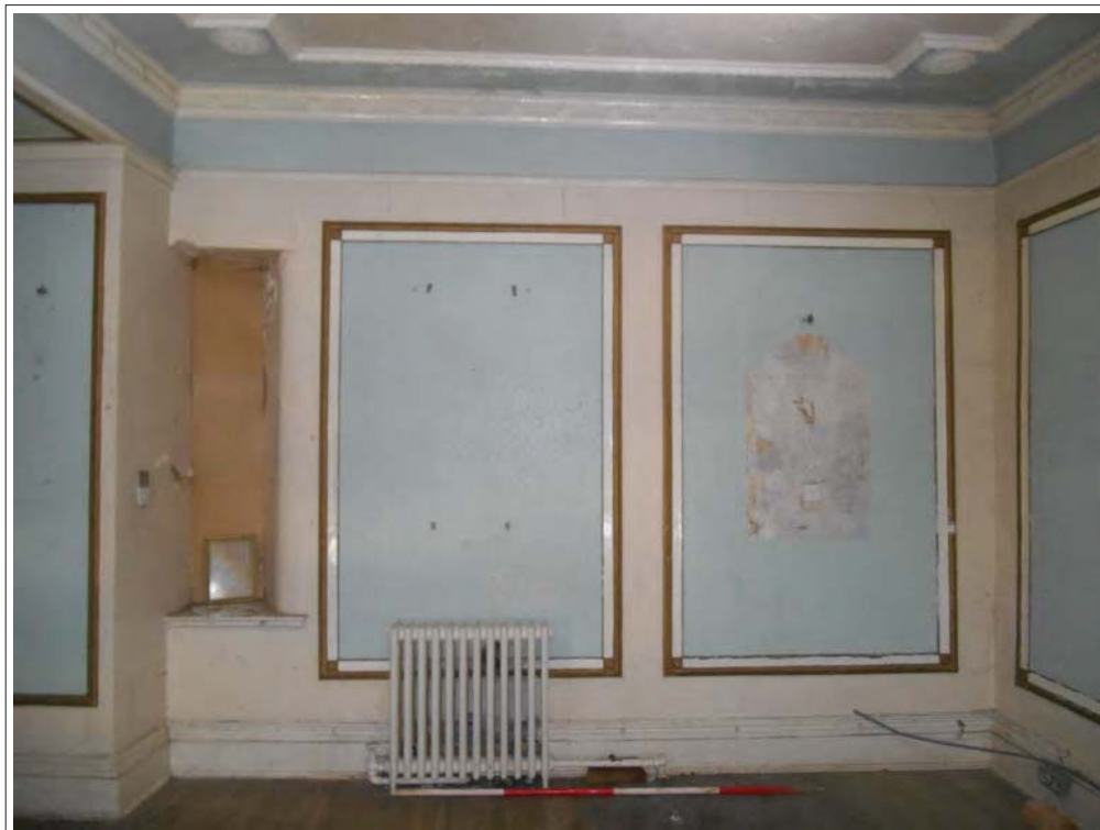
Plate 30. Detail of blocked window using projected wall, looking SW.
