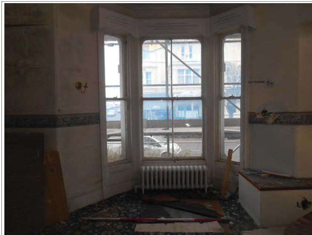
Plate 40. Canted three-light window, looking N.
