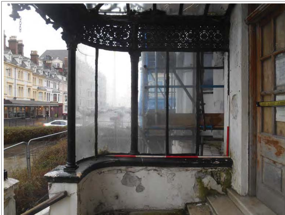
Plate 6. Detail of entrance porch, looking N.
