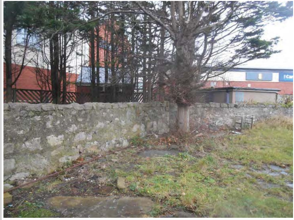
Plate 174. Detail of circuit wall viewed from back entrance.
