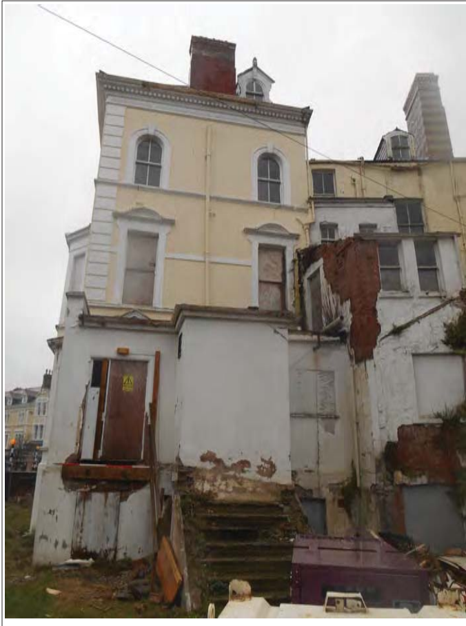
Plate 11. View of extension 1, looking NW.
