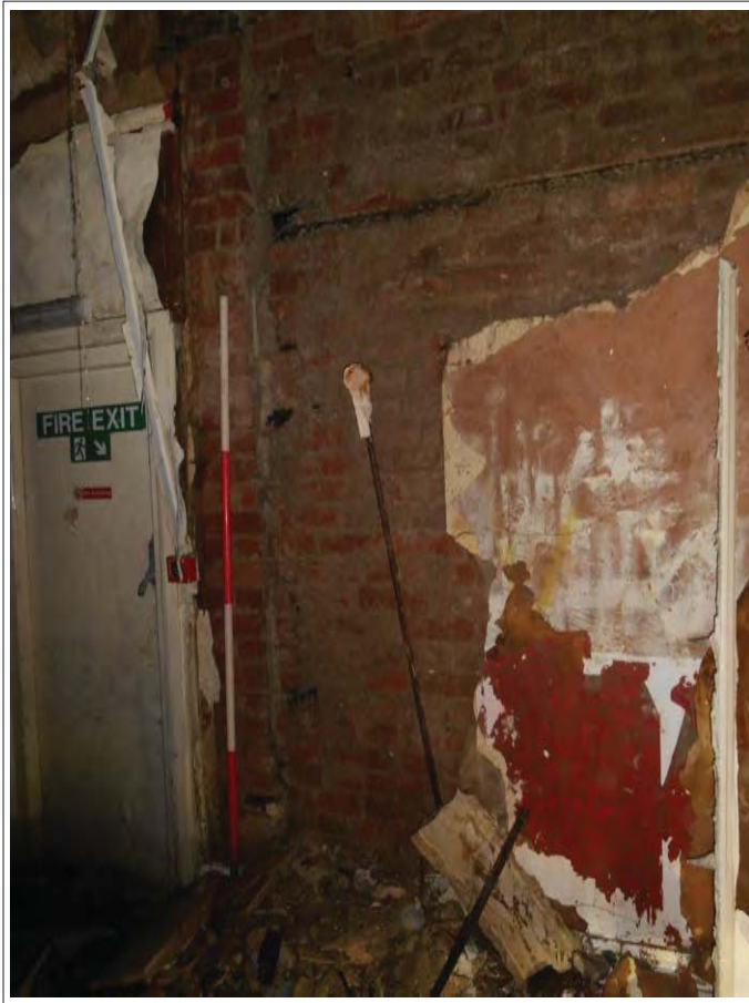
Plate 51. Original brickwork, looking S.
