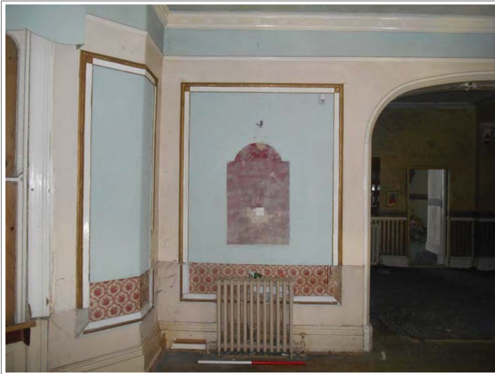
Plate 35. Reception wall showing different layers of decoration, looking NNW.
