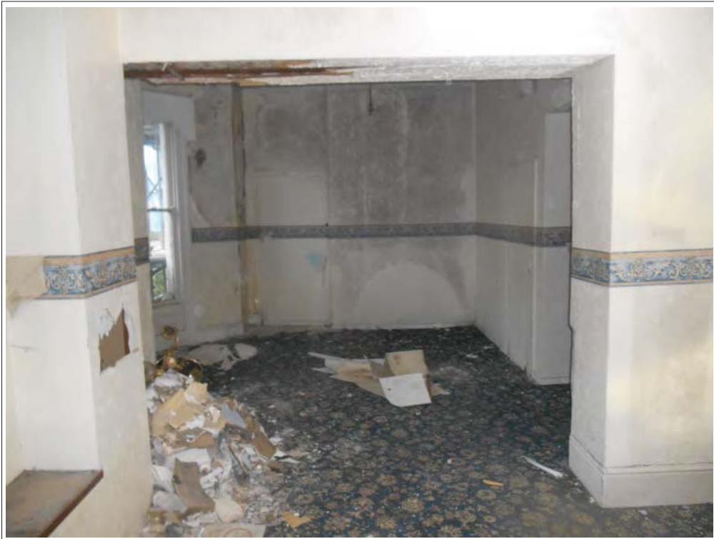
Plate 39. Blocked door predating current wall decoration, looking E.
