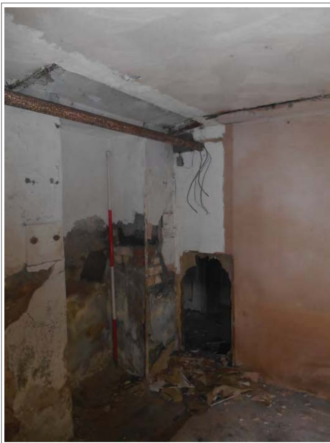
Plate 112. View of wall addition, looking NE.
