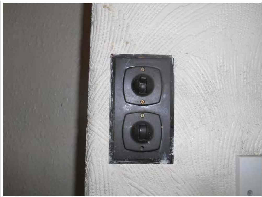
Plate 94. Detail of electrical fitting from Room 6, looking S.
