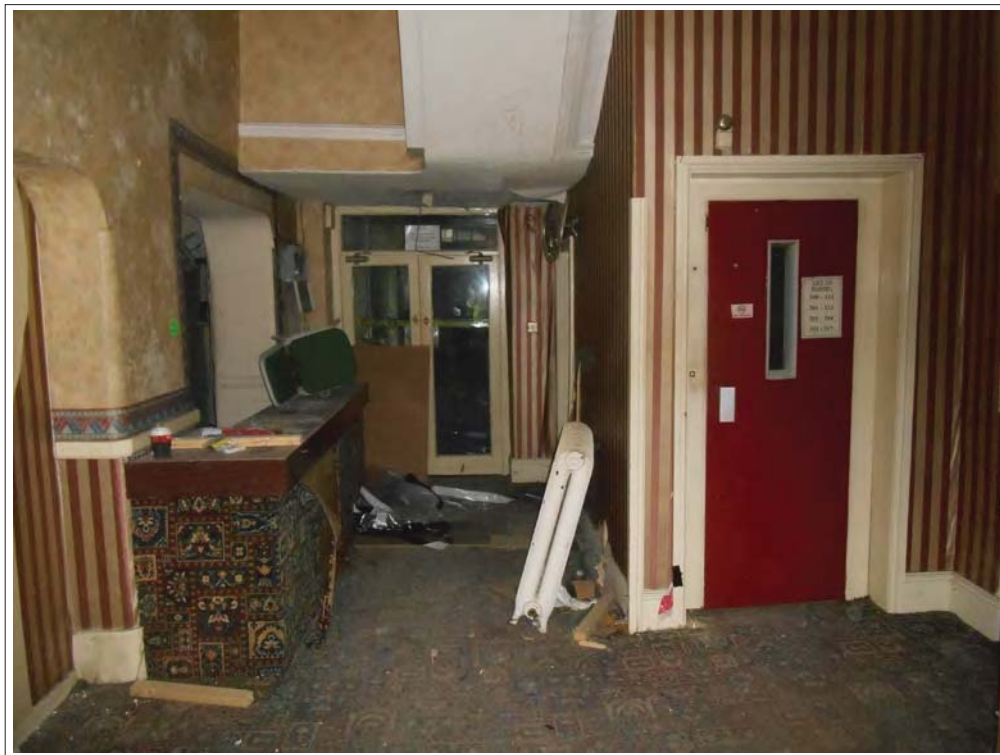
Plate 36. Reception area, looking NNW.
