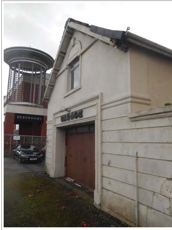
Plate 130. View of entrance. Looking southeast.
