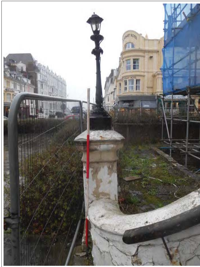
Plate 4. Detail of entrance lantern, looking N.
