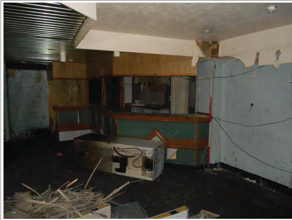
Plate 122. Bar area, looking E.
