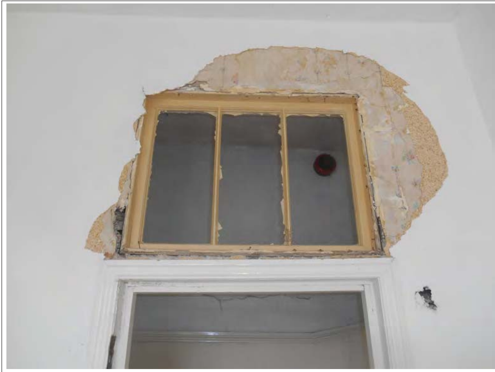
Plate 85. Detail of light box, Room 10, looking W.
