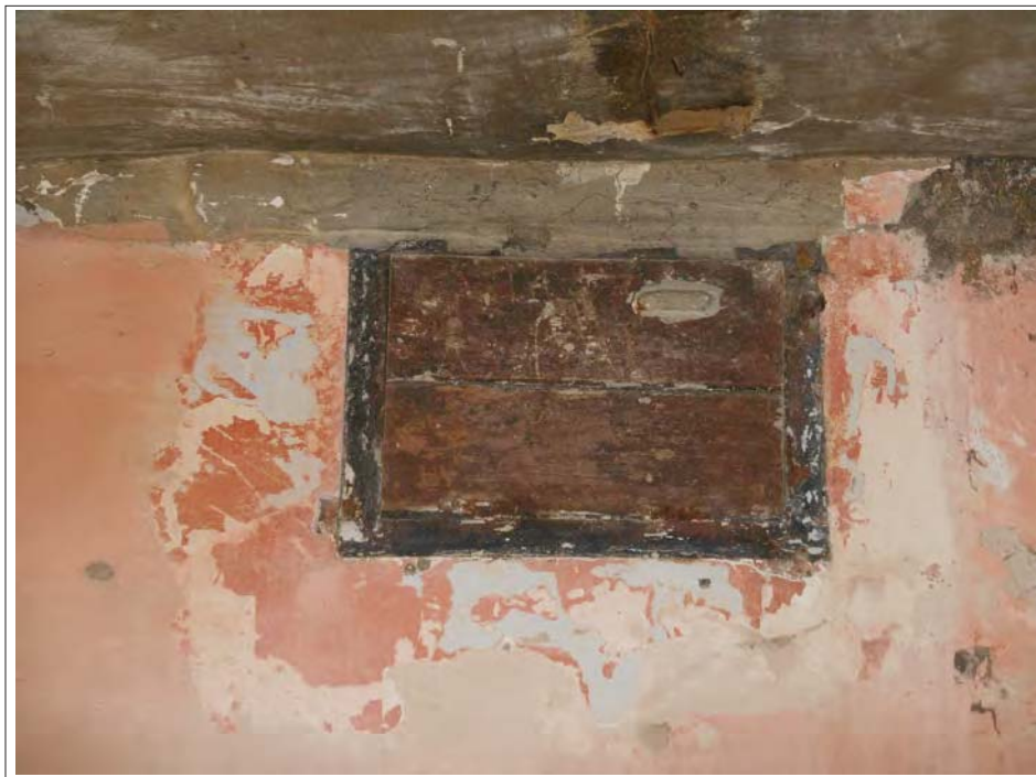
Plate 141. Possible vent, west facing wall.
