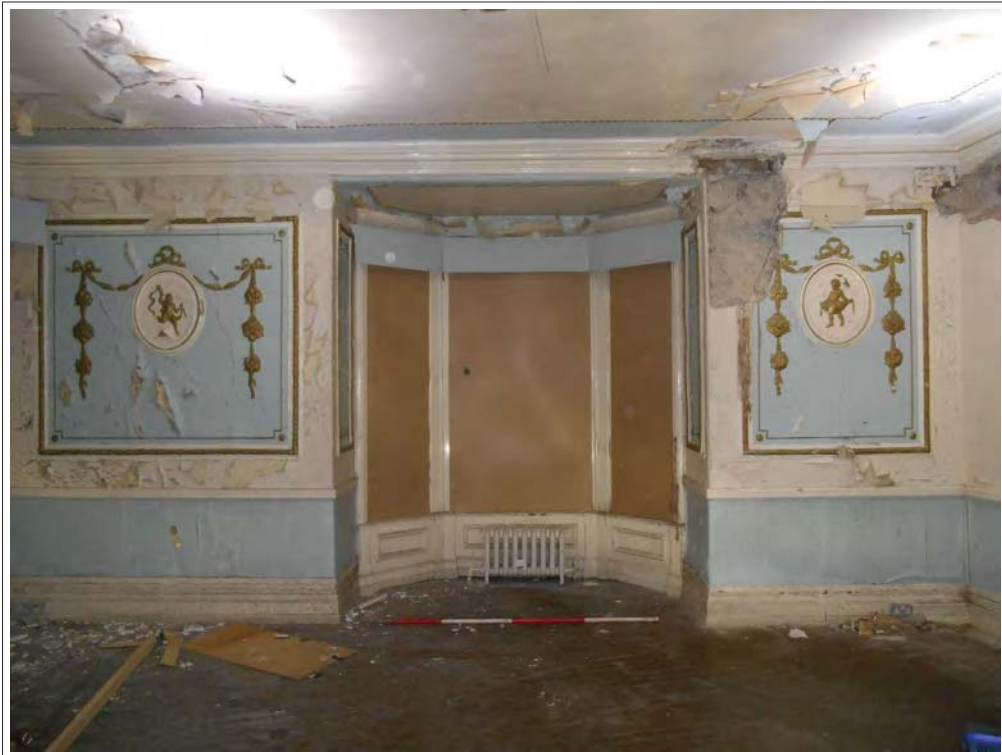
Plate 27. Storeyed canted three-light windows from ballroom, looking WSW.
