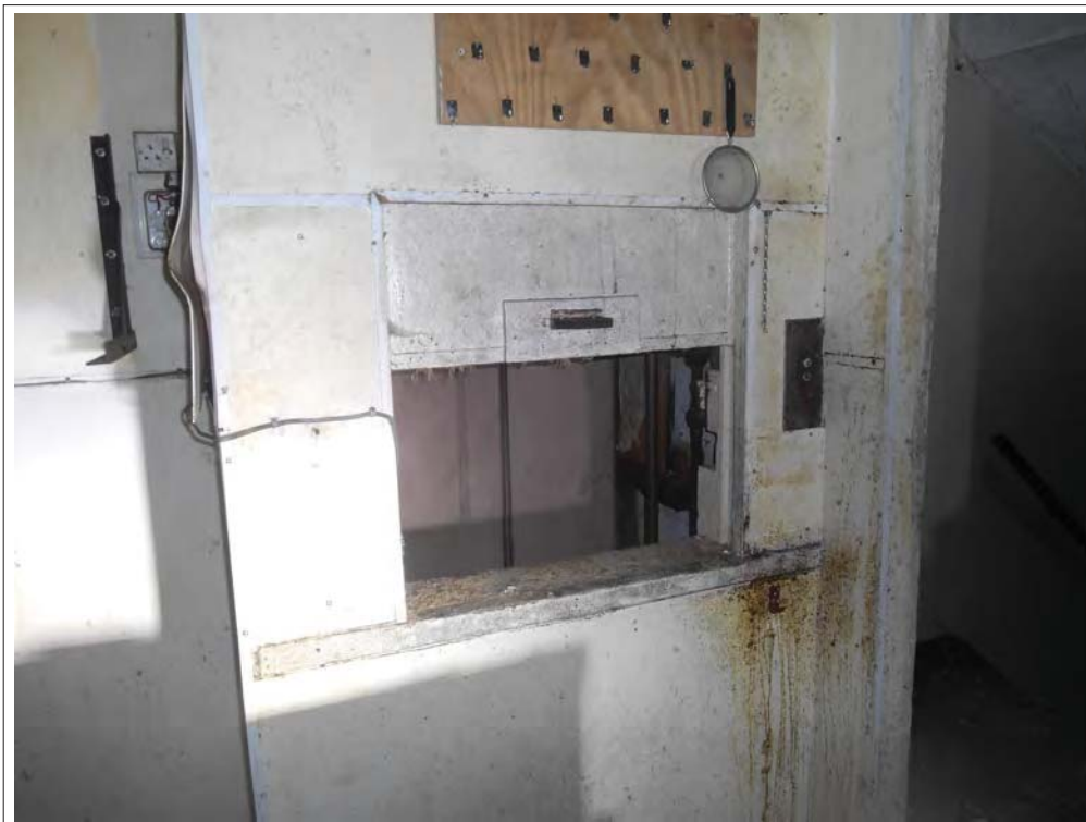
Plate 22. Detail of kitchen 1, looking W.
