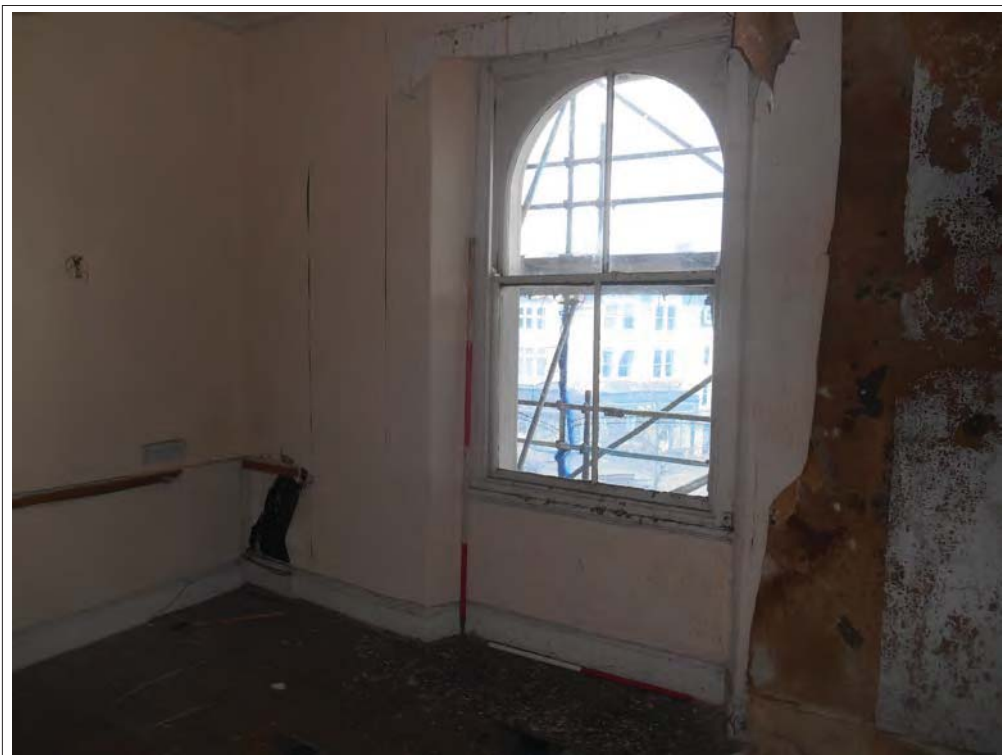
Plate 84. View of Room 3, with round-headed sash window and multiple layers of wall paper, looking SW.
