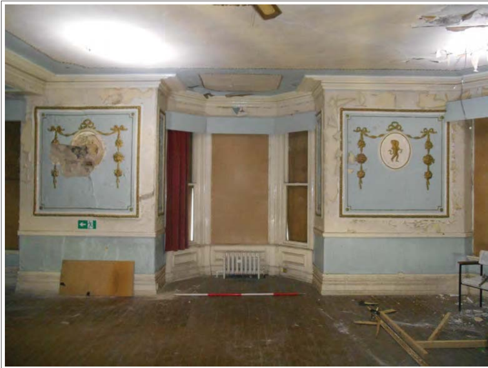
Plate 25. Canted three-light window from ballroom, looking SE.
