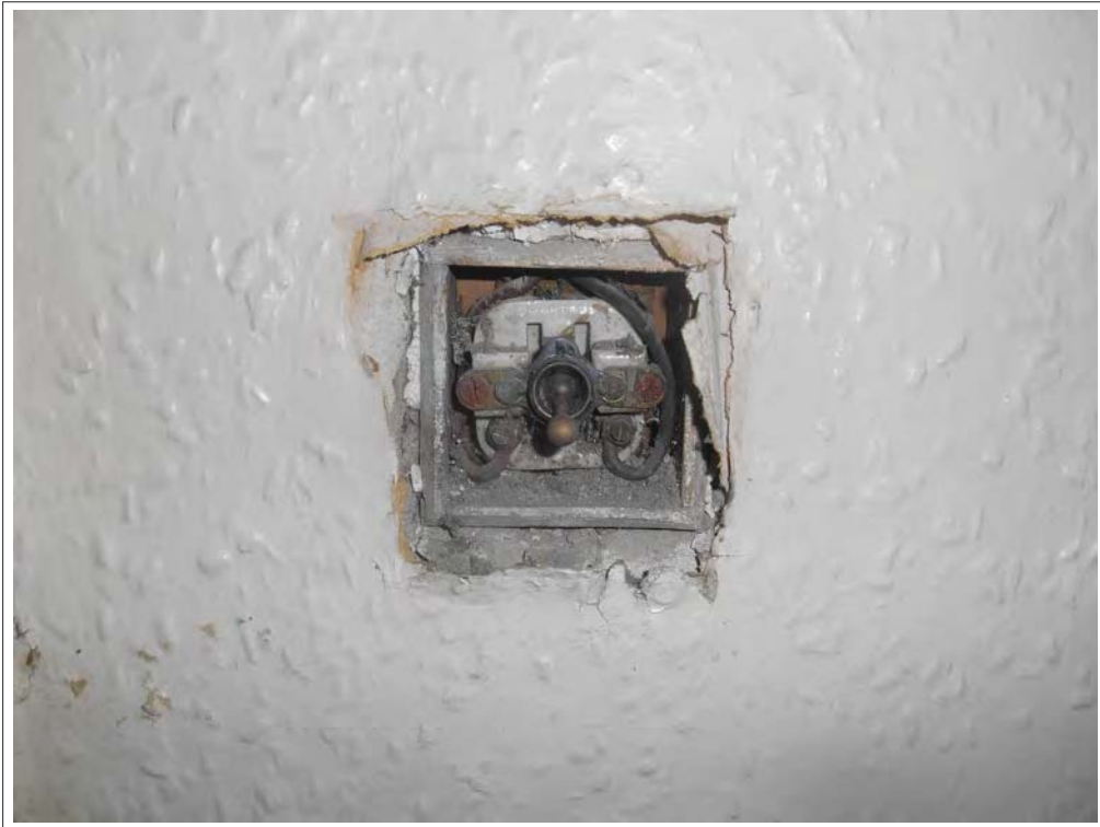
Plate 95. Detail of electrical fitting from Room 6, looking S.
