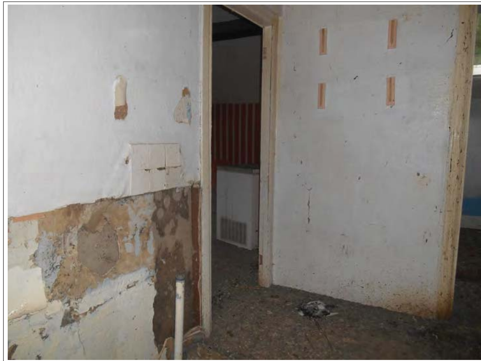
Plate 163. First floor, looking north.
