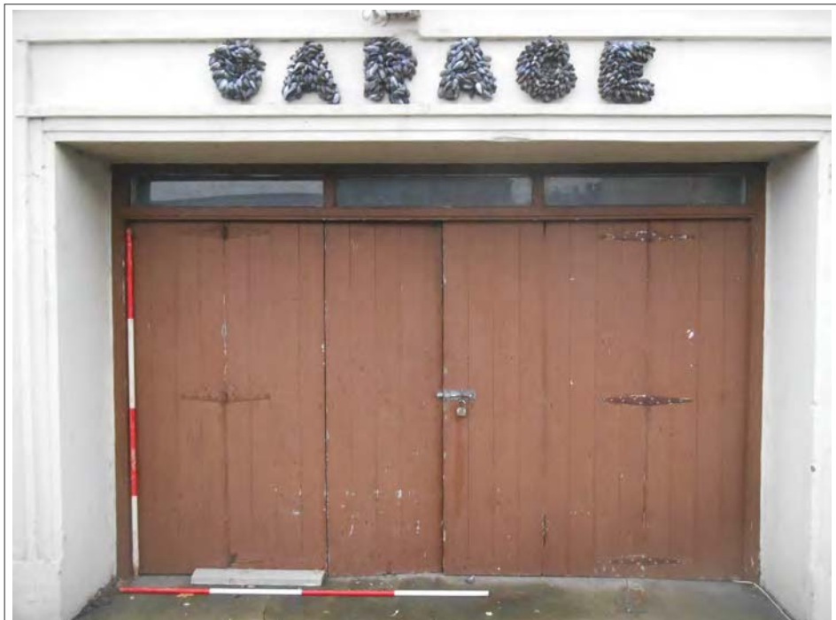
Plate 129. Main garage entrance. Looking south.
