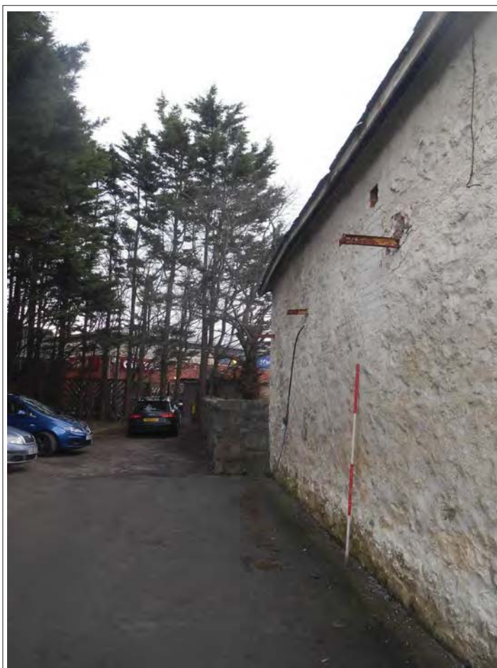
Plate 150. View showing relationship between garage and circuit wall.
