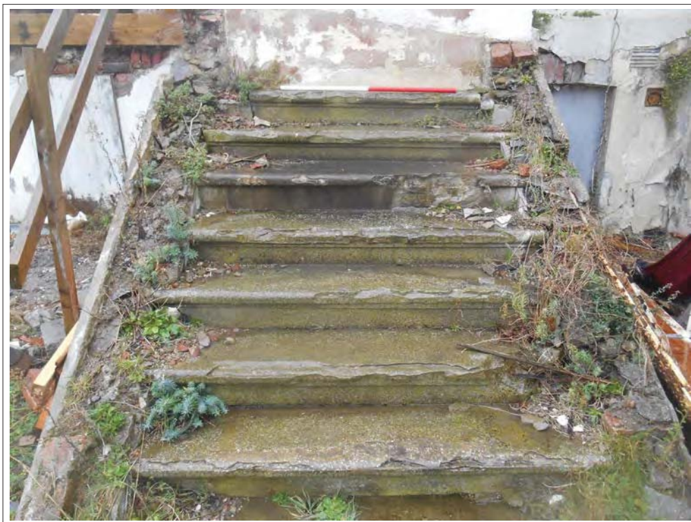
Plate 12. Detail of staircase leading to extension 1, looking W.
