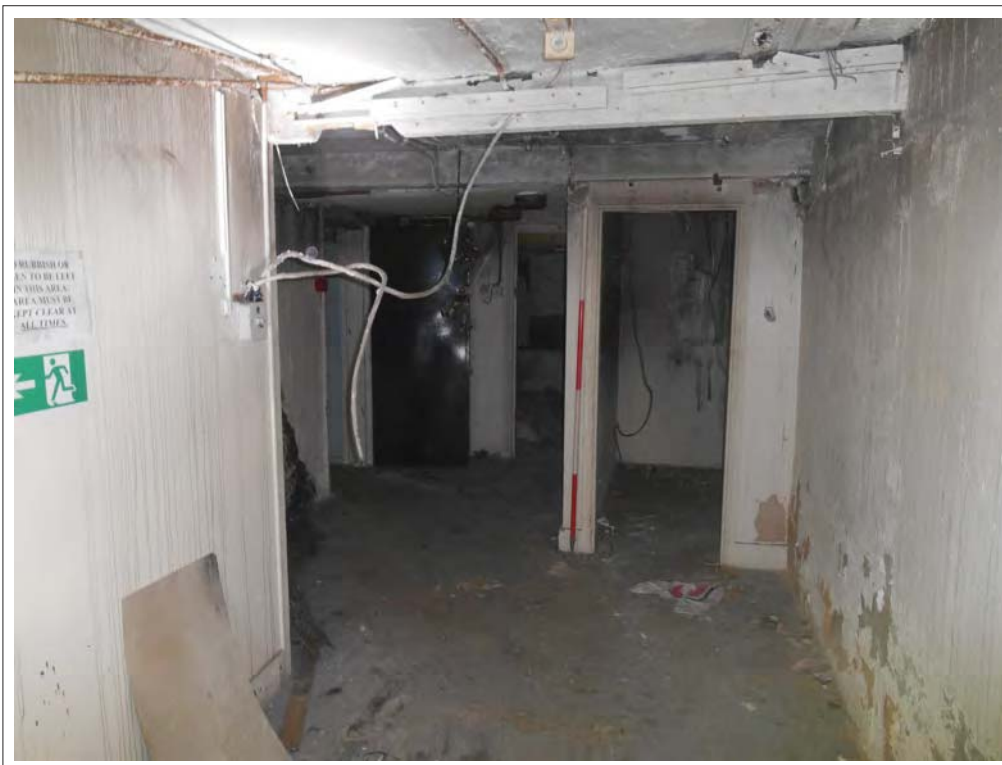
Plate 124. Toilet facilities, looking NW.
