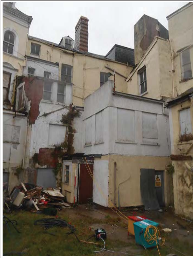
Plate 13. View of extension 2, looking NW.
