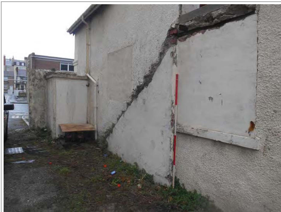
Plate 168. Outbuilding attached to garage behind facade wall. West facing wall.
