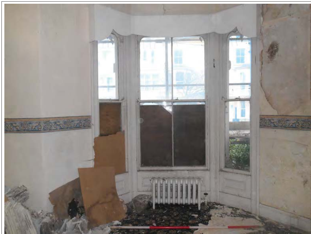
Plate 42. Canted three-light window. Looking N.
