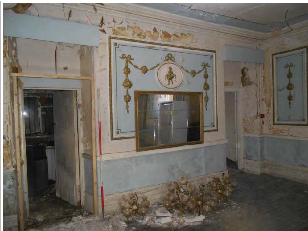
Plate 18. View of altered wall. Fireplace replaced for panelled wall. Looking E.
