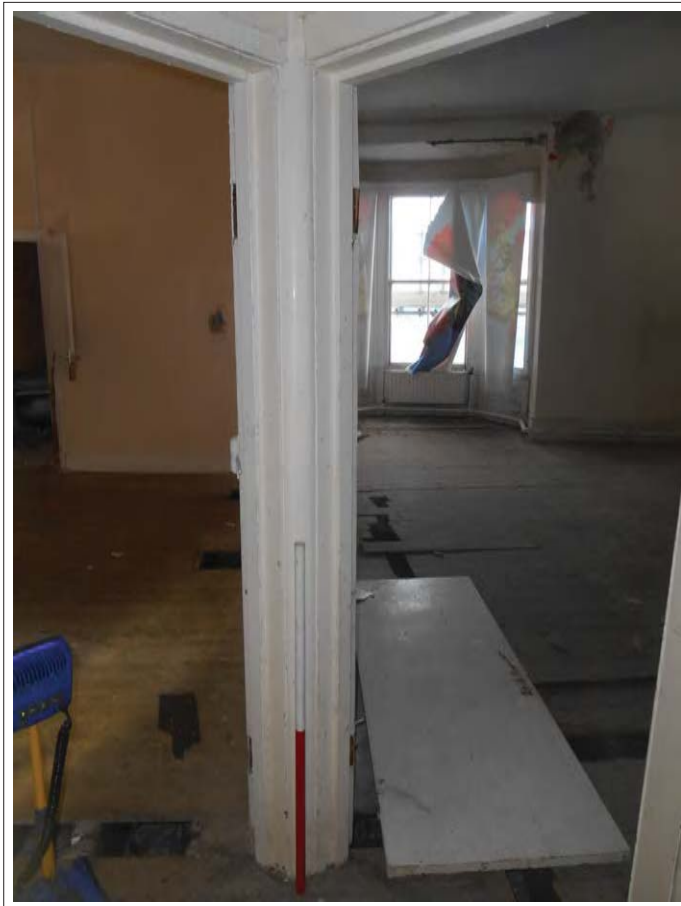
Plate 53. Dividing wall between Room 1 and 2, looking ESE.
