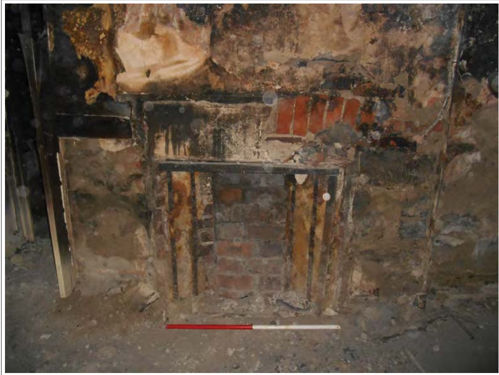
Plate 126. Original fireplace, looking SSW.
