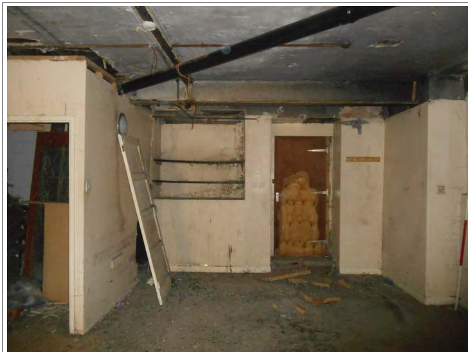
Plate 137. North facing wall. Inset blocked window transformed into shelving.
