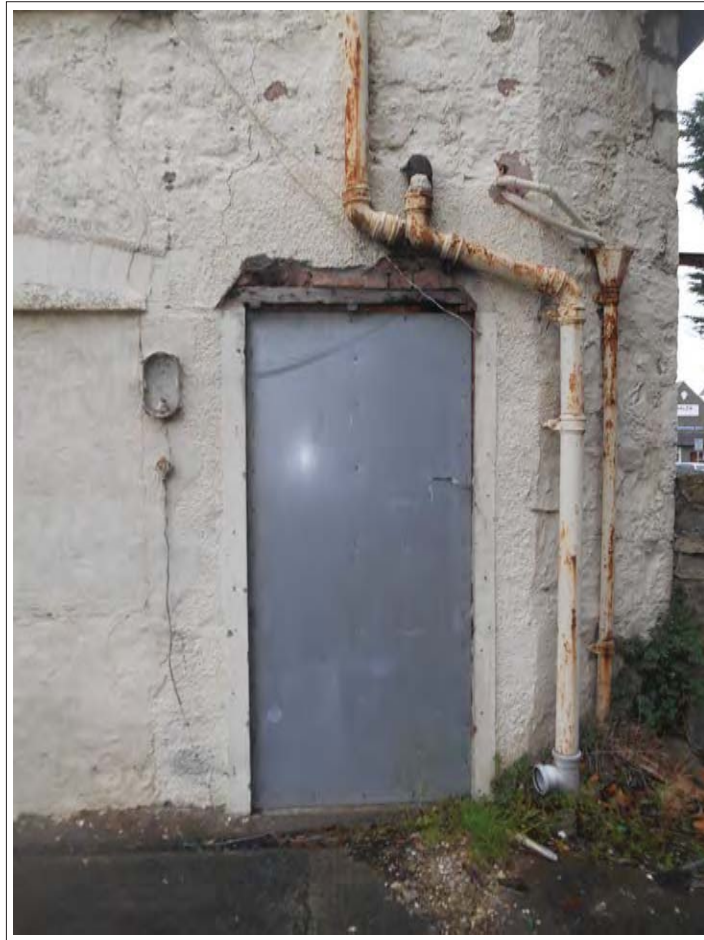
Plate 154. Detail of door associated to internal studded wall room.
