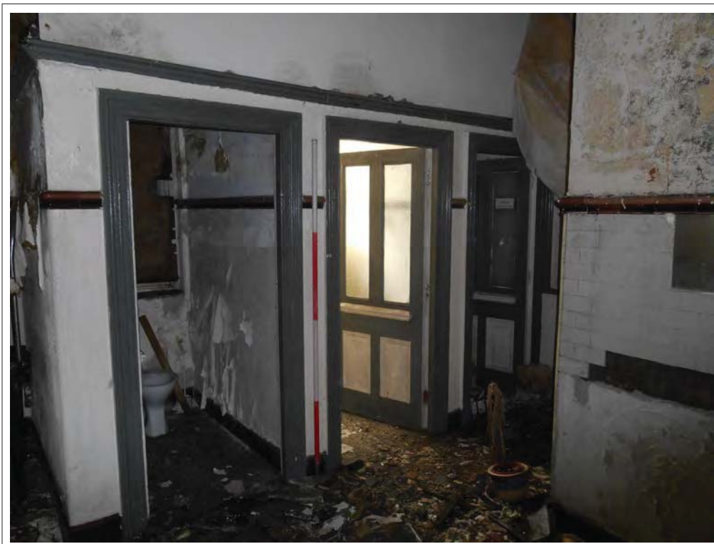
Plate 52. View of toilet facilities, looking SE.
