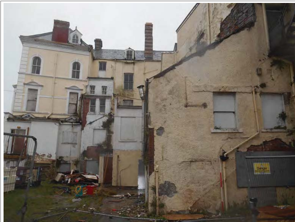
Plate 16. View of side and rear elevations, looking SW.
