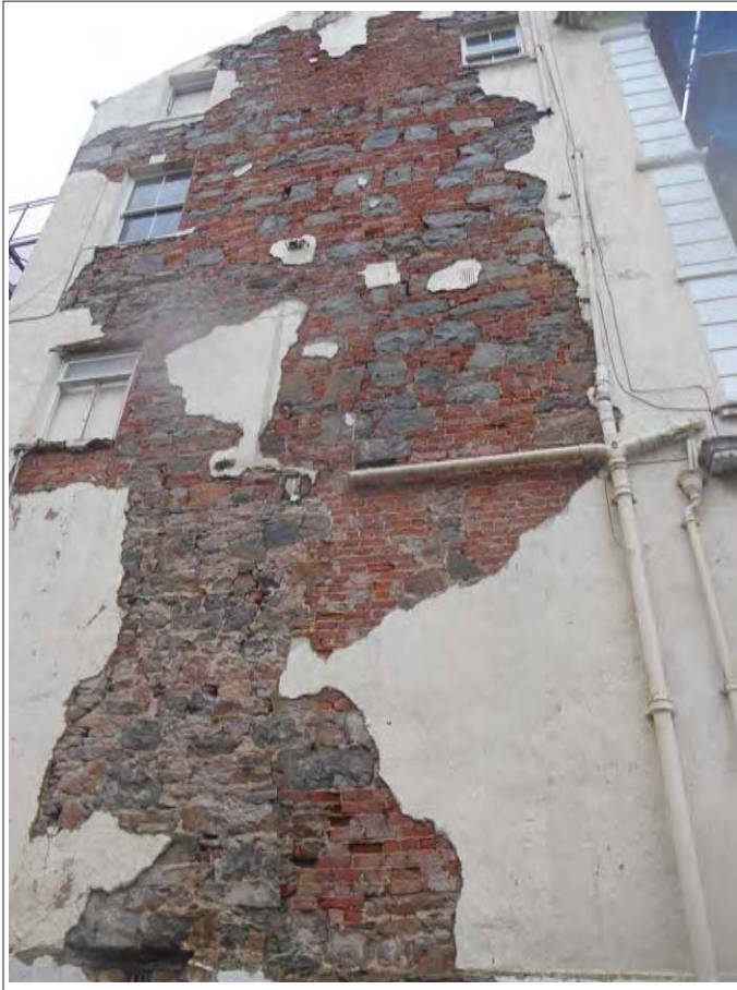
Plate 17. Detail of wall construction and alterations, looking W.
