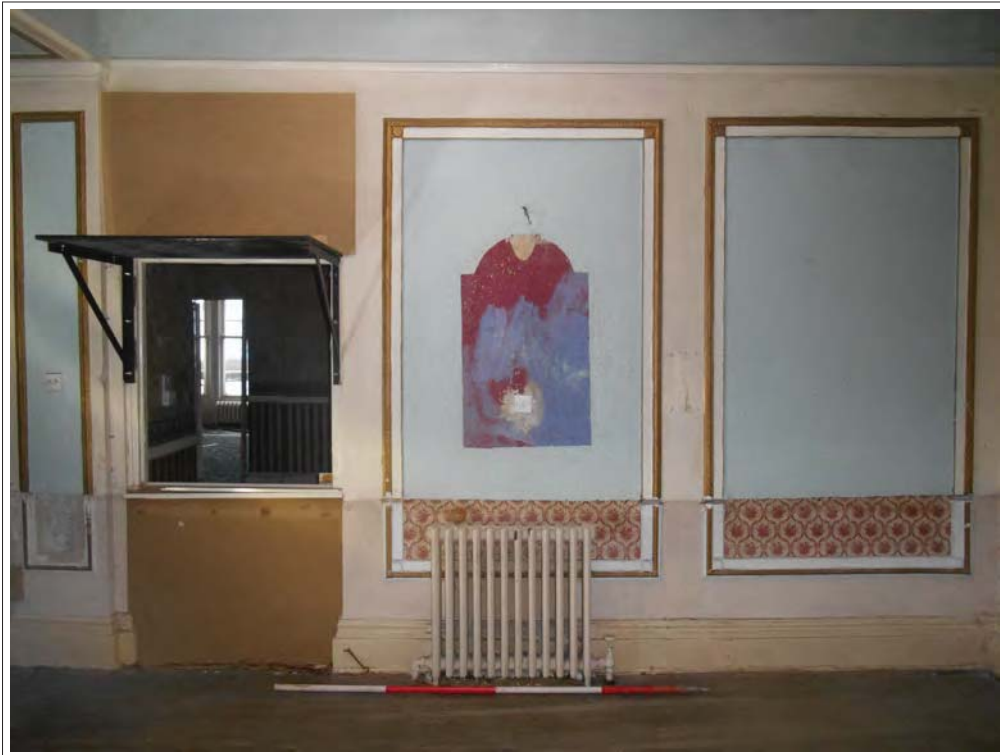
Plate 37. View of blocked door, reception area, looking E.
