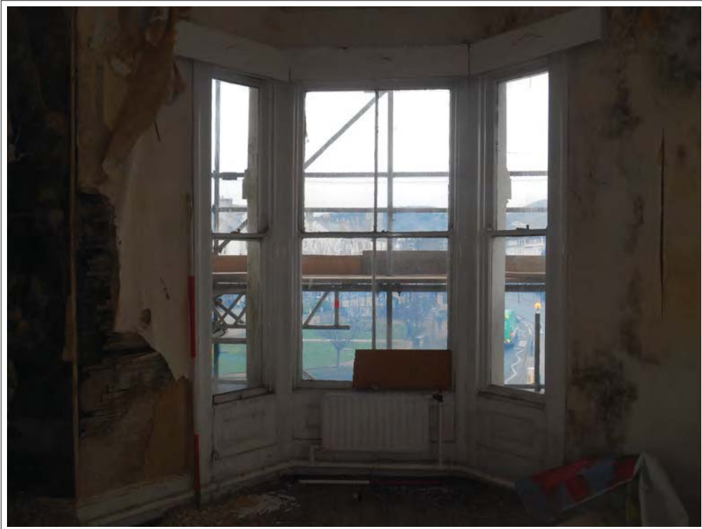
Plate 71. View of Room 7 with storeyed canted three-light window, looking W.
