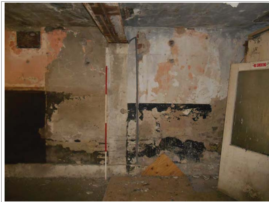
Plate 139. West facing wall.
