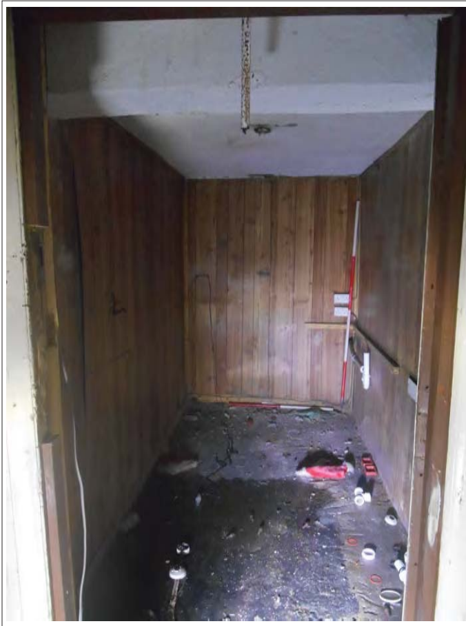
Plate 109. View of room addition, looking ESE.
