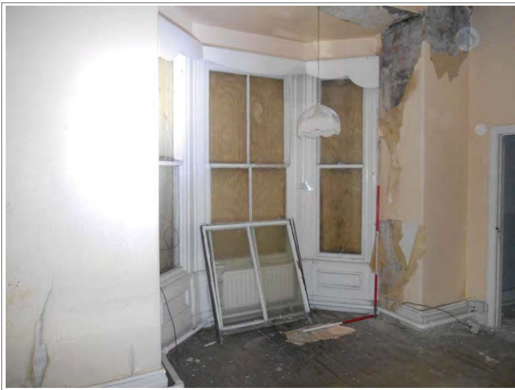
Plate 54. View of Room 1 with canted three-light window, looking SSW.
