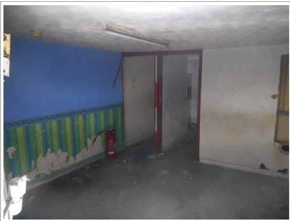
Plate 111. Toilet facilities, looking N.
