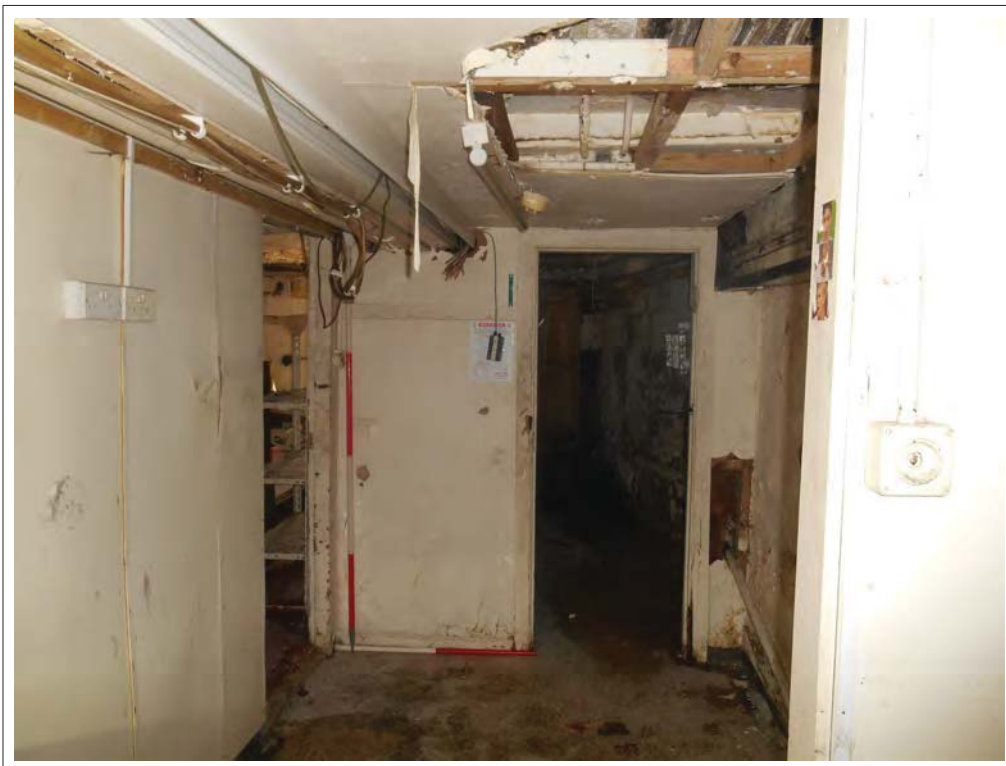
Plate 119. From kitchen, view to cellar. Looking S.
