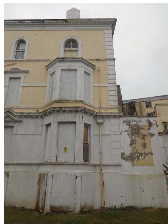
Plate 10. View of eastern elevation, looking NW.
