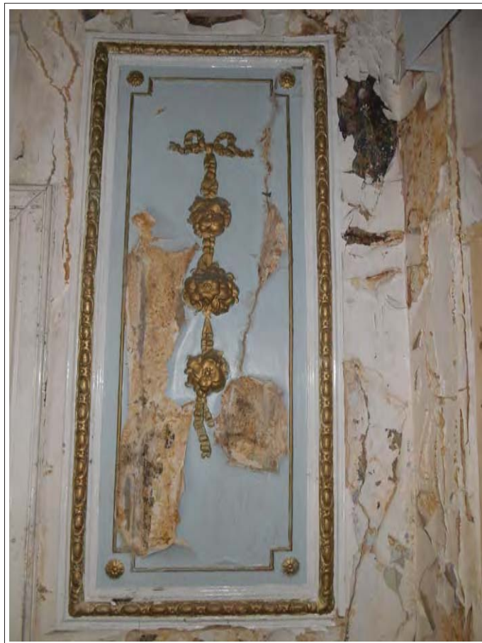
Plate 20. Detail of decorated panel adjacent to blocked door, looking S.
