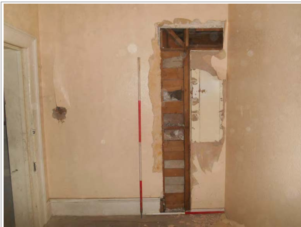
Plate 70. View of Room 8. Storeyed canted three-light window blocked by wall addition. Looking N.
