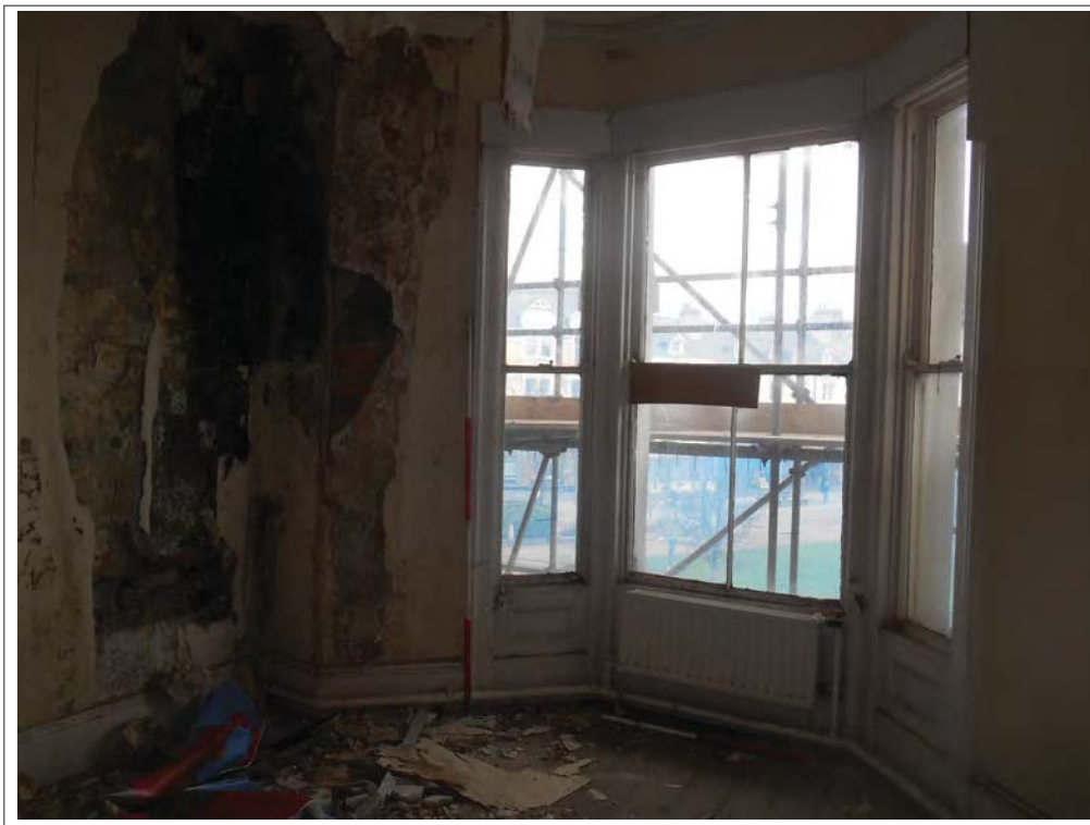
Plate 62. View of Room 5, with storeyed canted three-light window, looking W.
