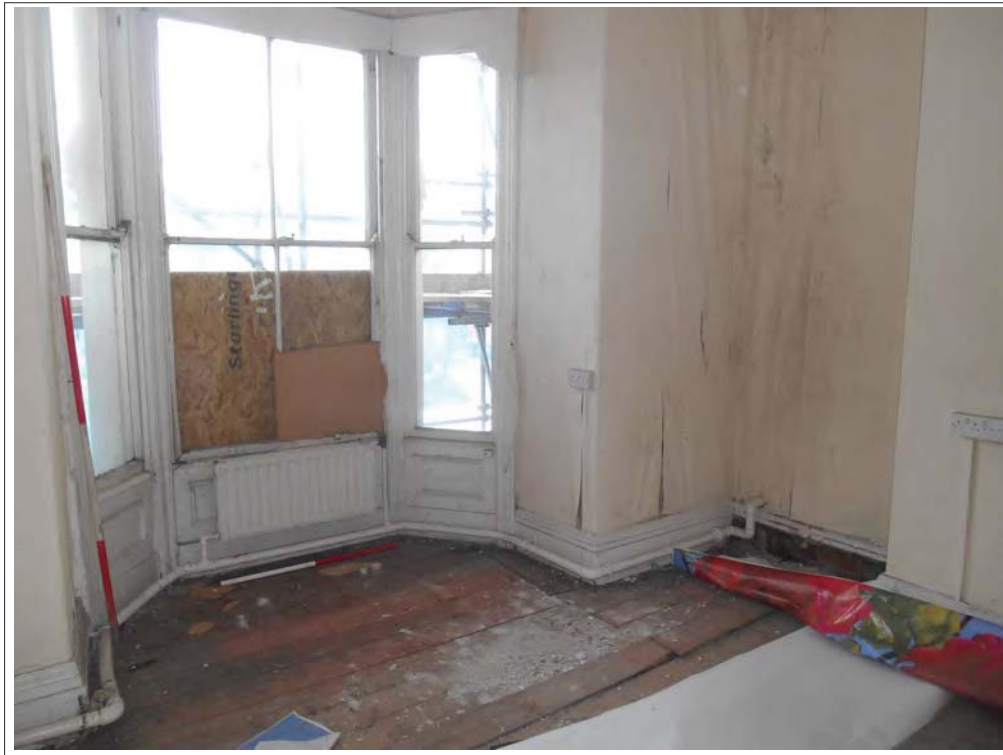
Plate 61. View of Room 4, with storeyed canted three-light window, looking W.
