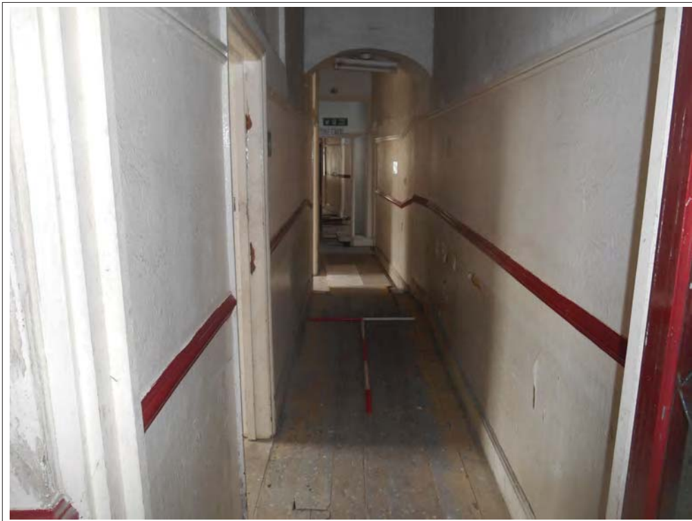
Plate 88. View of corridor, looking S.
