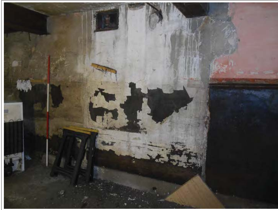
Plate 142. West facing wall.
