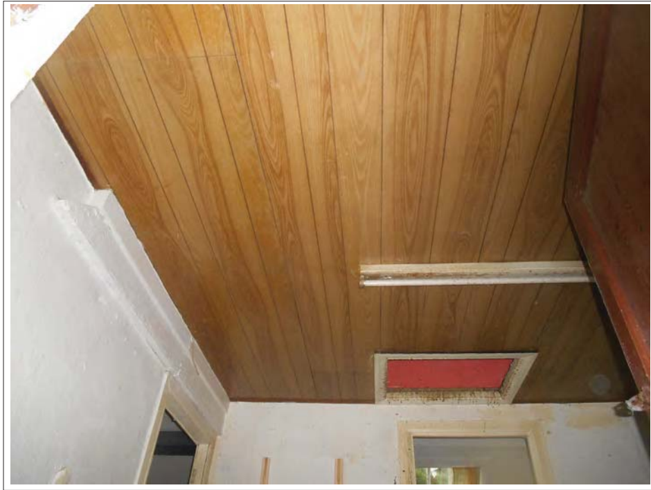
Plate 164. First floor sealing.
