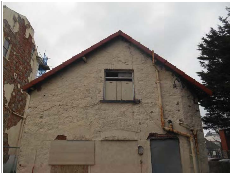
Plate 155. Detail of first floor window.
