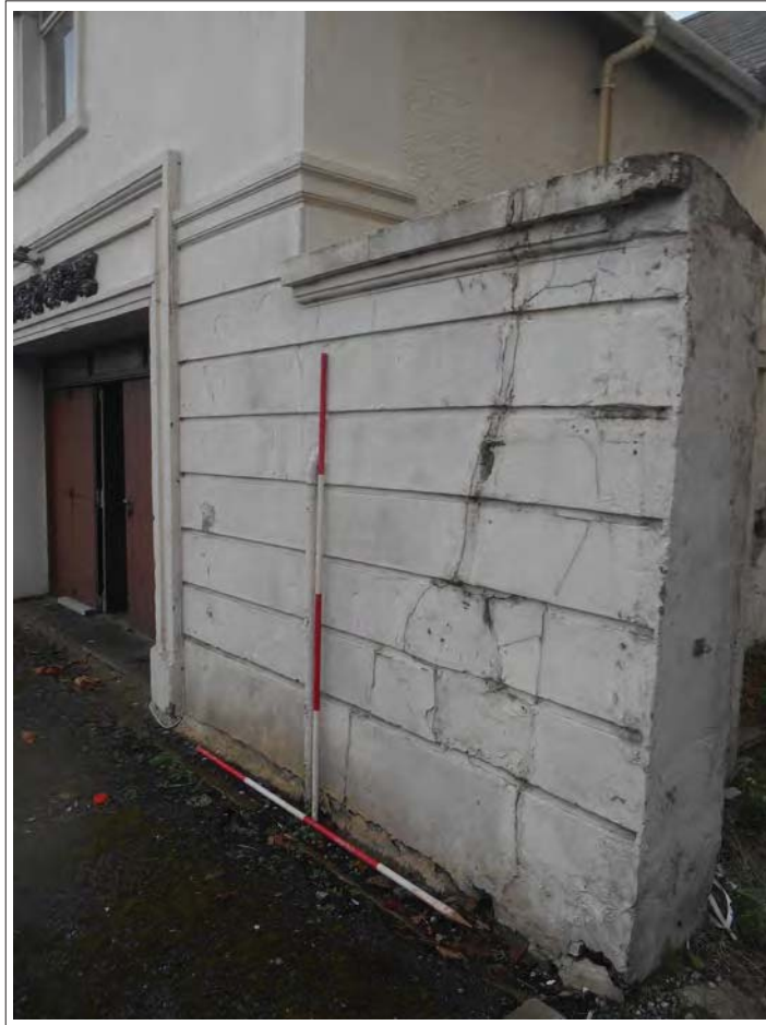
Plate 128. View of western wall of facade. Looking south.
