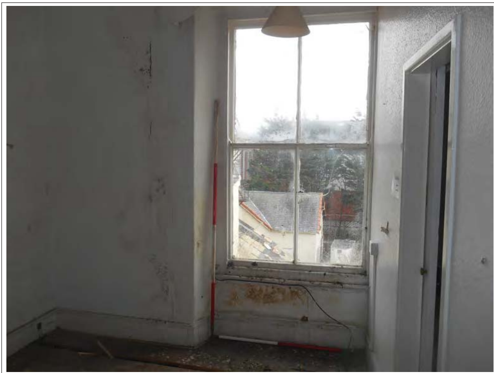
Plate 86. View of Room 10 with centre bar window, looking E.
