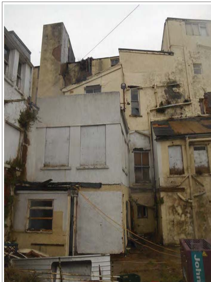
Plate 14. View of extension 2 and 3, looking N.
