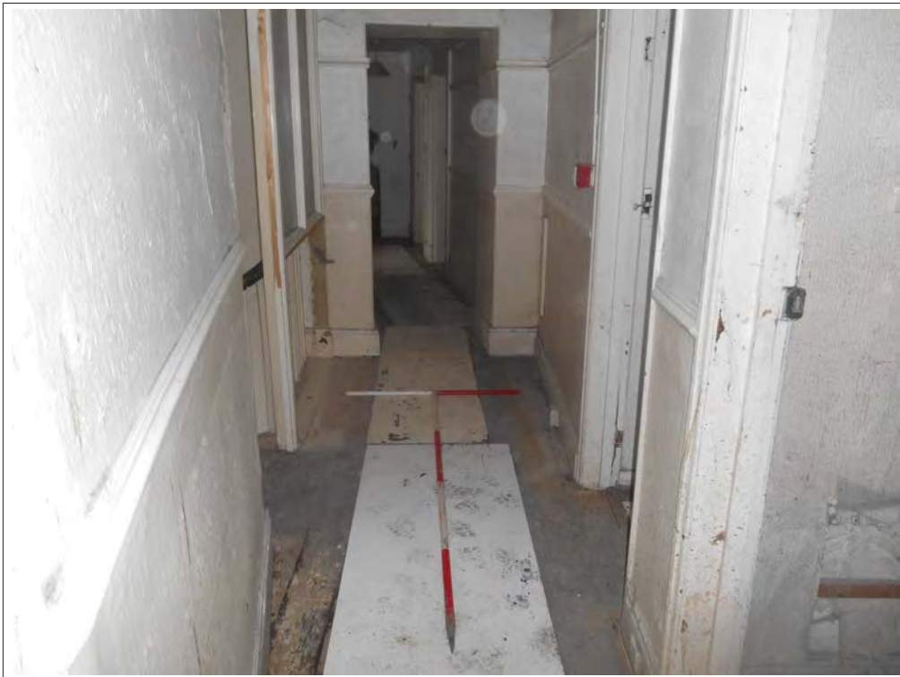
Plate 104. View of corridor, looking S.
