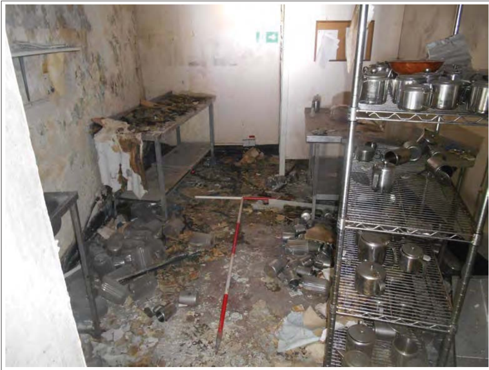
Plate 23. View of kitchen 2, looking N.
