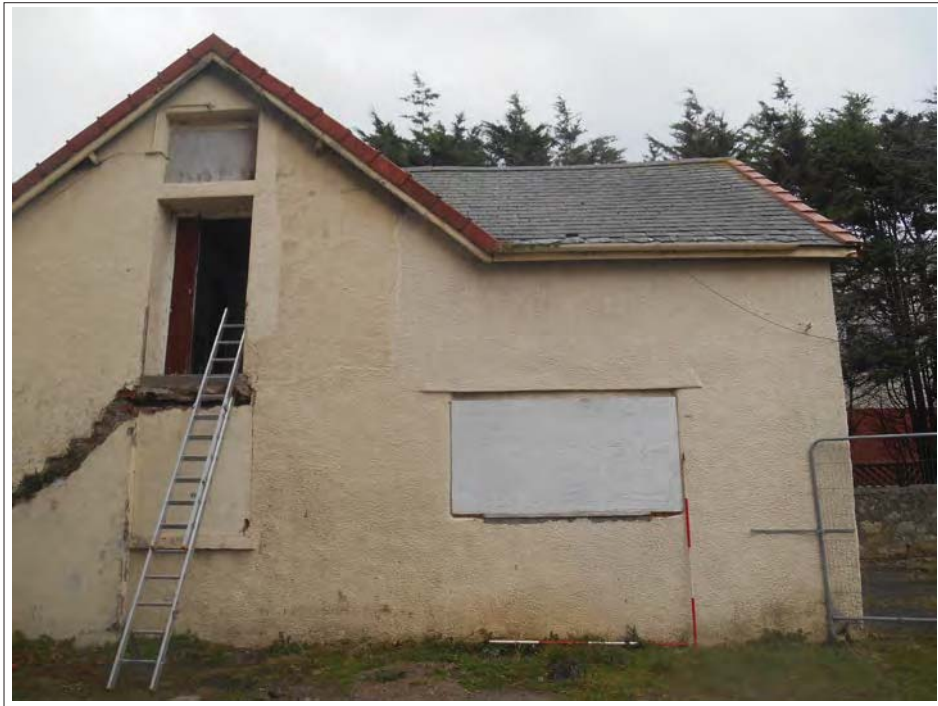
Plate 160. View of east facing wall.
