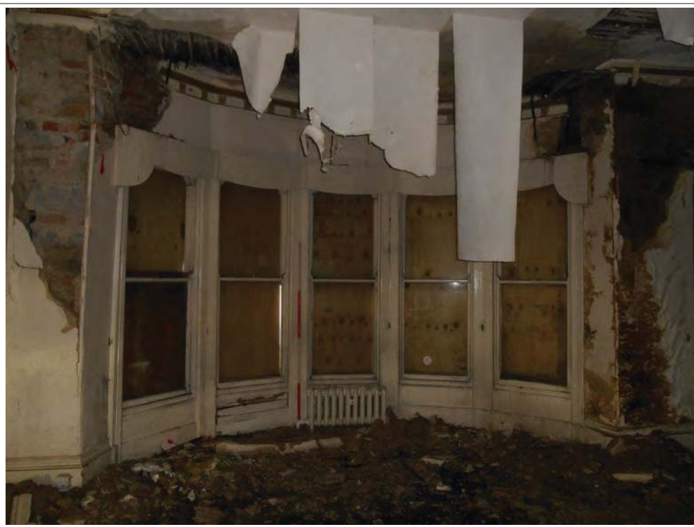
Plate 46. Canted five-light window, looking N.
