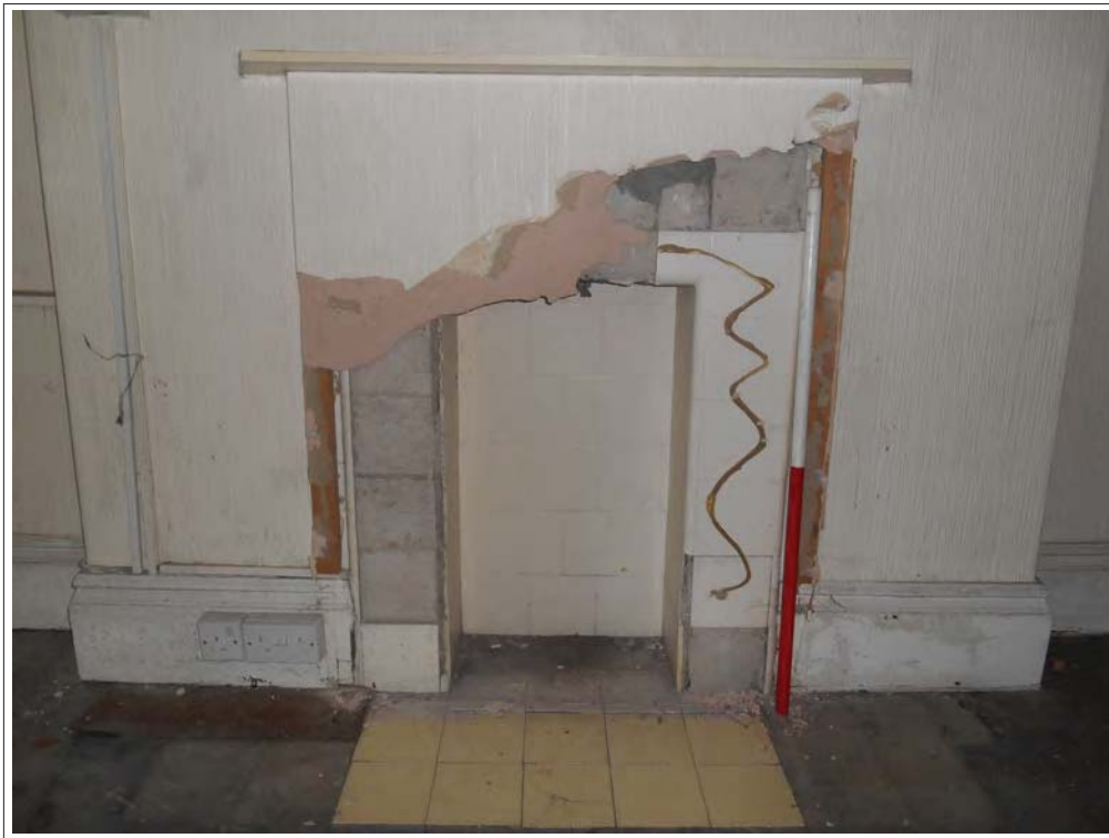
Plate 56. Location of original fireplace. Room 2, looking N.
