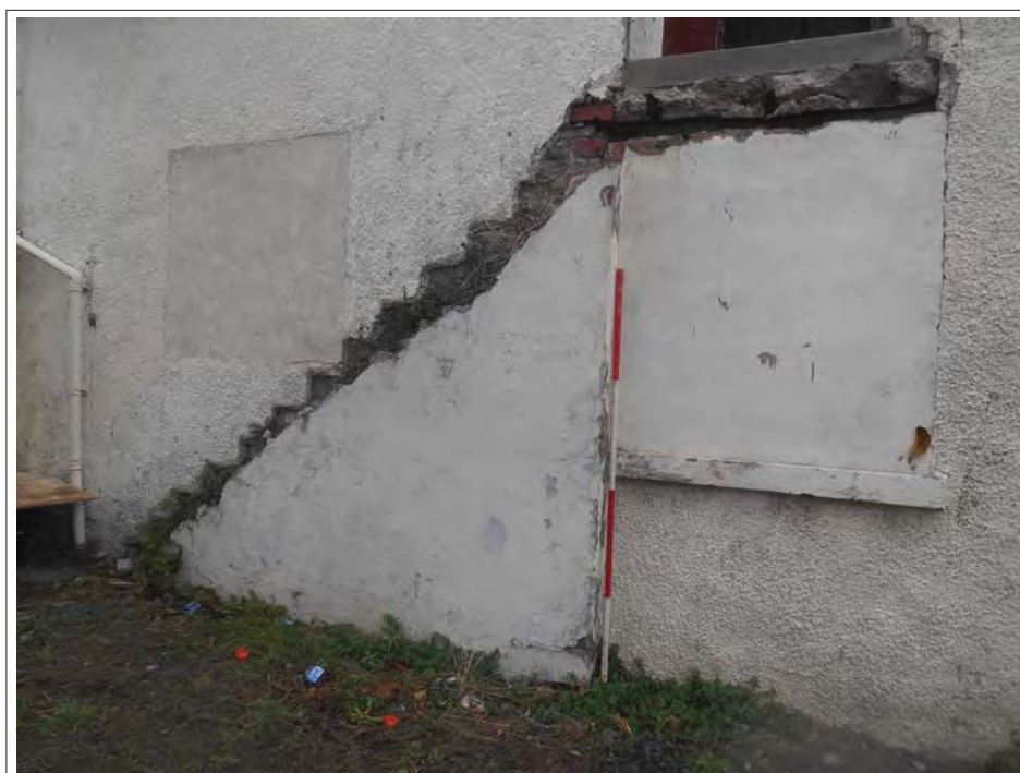
Plate 167. Detail of exterior stair case and doorway/window. Scale 2m
