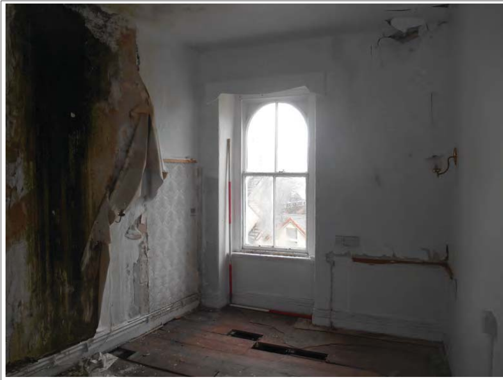
Plate 79. View of Room 12, with round-headed sash window and multiple layers of wall paper, looking NE.
