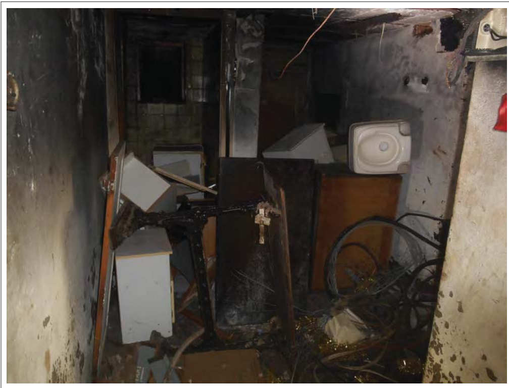
Plate 115. Storage room, looking S.
