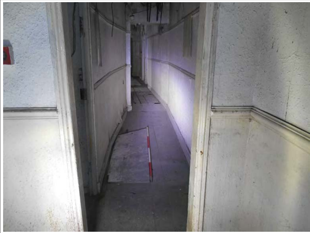
Plate 103. View of corridor, looking S.
