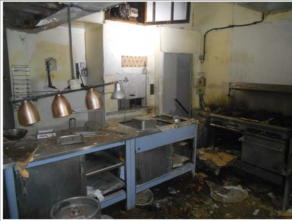
Plate 21. View of kitchen 1, looking N.
