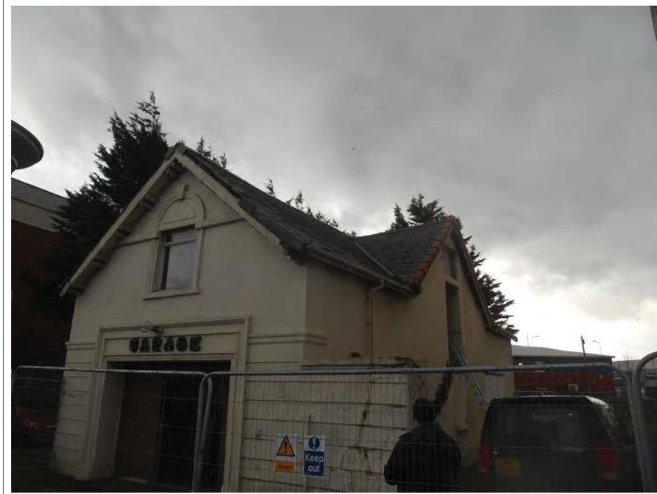
Plate 146. View of garage facade.
