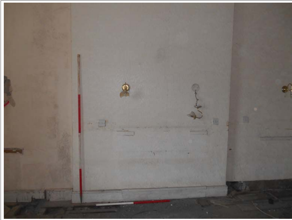
Plate 93. Location of original fireplace Room 7, looking E.
