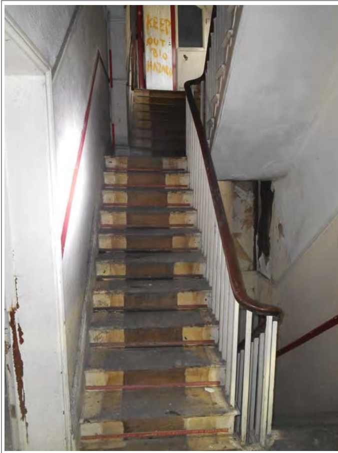
Plate 91. View of staircase, looking E
