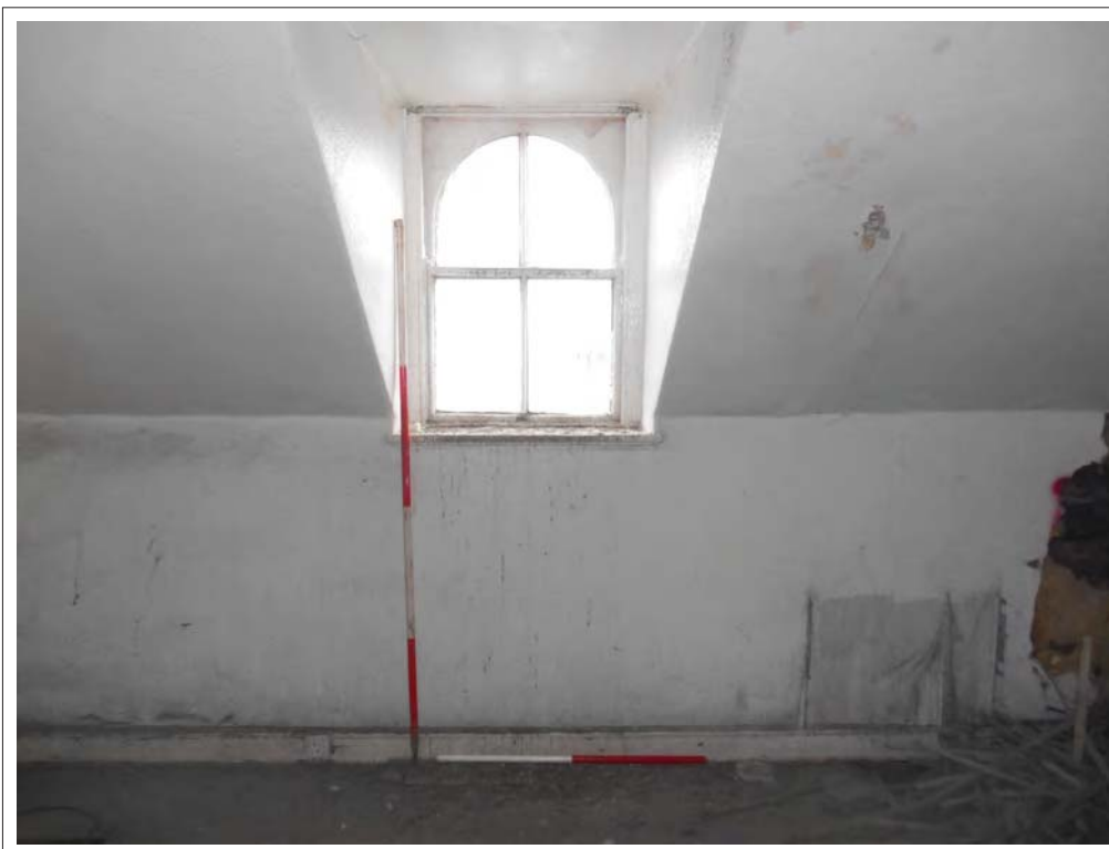
Plate 107. View of attic window, looking E.
