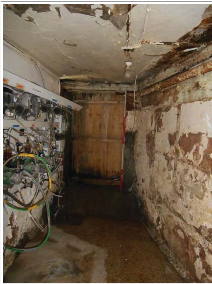
Plate 120. View to cellar, looking E.
