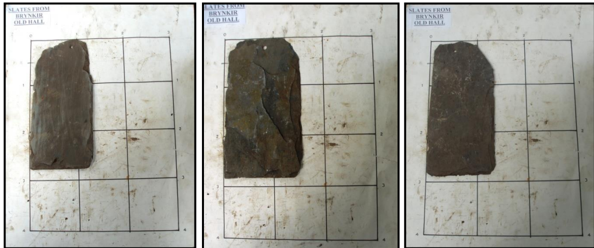
Brynkir slate from the left hand side of the roof
