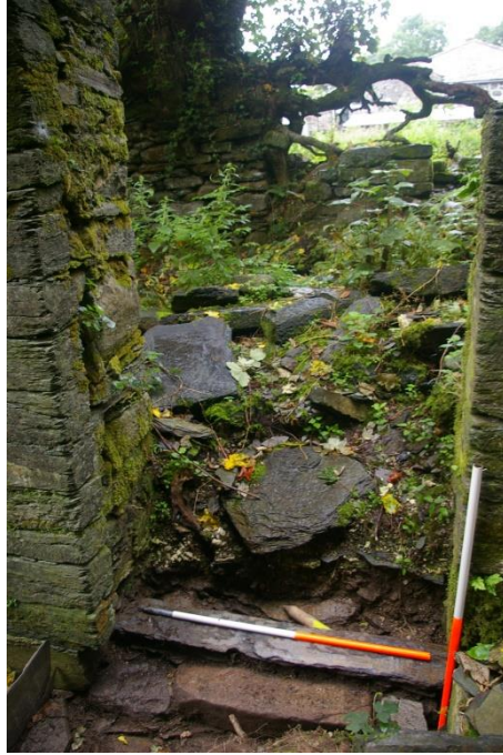
Figure 19: Trench I. The Doorway of the 17 th Century hall, showing the slate threshold (where the ranging pole is resting) sitting on top of the earlier dolerite threshold stone. Notice the squared mudstone “Renaissance” wall in front of the earlier uneven wall. Photo: S.Doherty.
