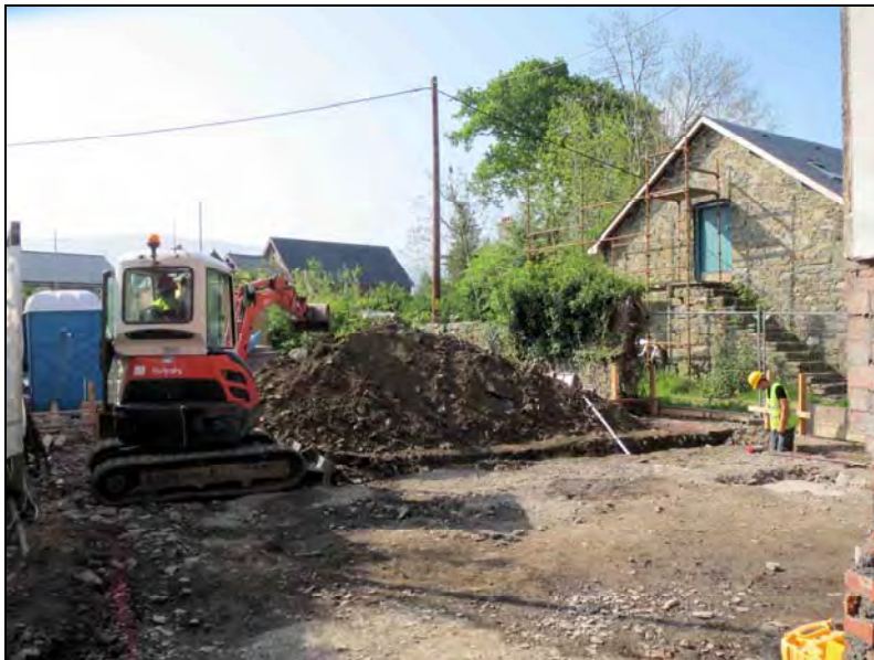
Plate 2. Working shot of the excavation. Looking south.
