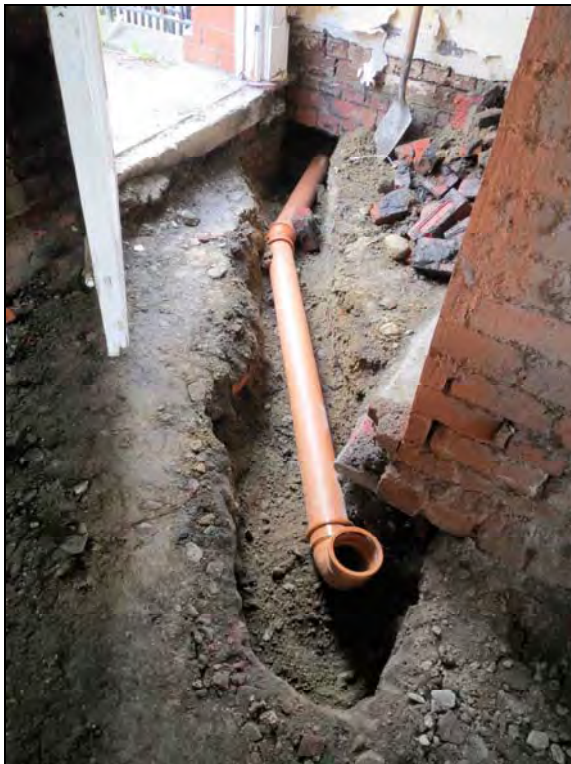
Plate 22. Excavation for new soil pipes, extending to East Street. Looking north-northeast.
