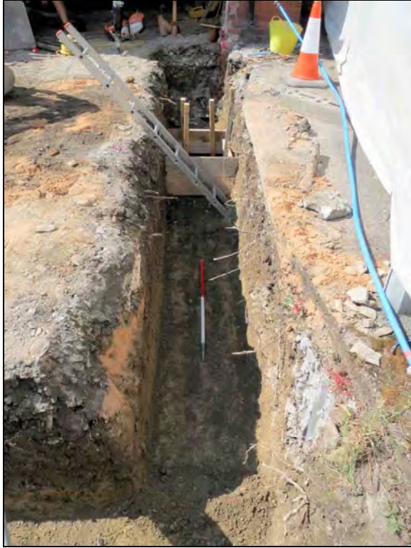
Plate 19. The northeast foundation trench. Scale: 1m. Looking northwest.
