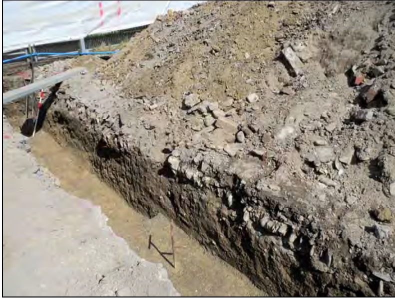
Plate 17. Oblique view of northwest-facing section along the southeast footing, showing buried cobbled surface. Looking east-northeast.
