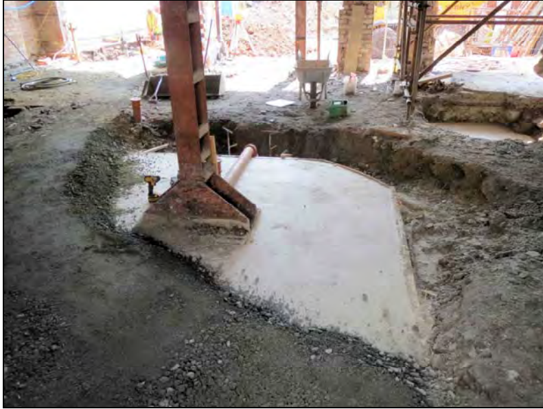
Plate 21. General shot of foundation bases within the building. Looking southeast.
