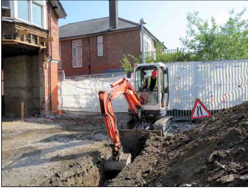
Plate 3. Working shot of the excavation. Looking northeast.
