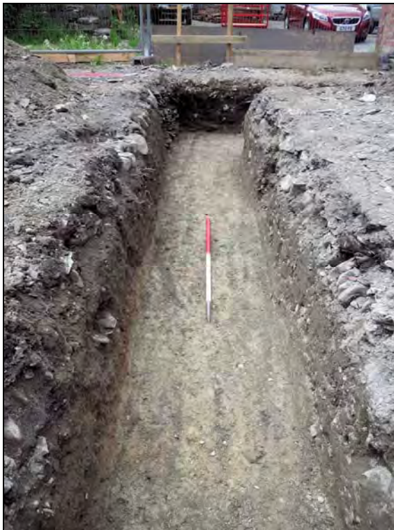
Plate 8. The southeast foundation trench. Scale: 1m. Looking southwest.
