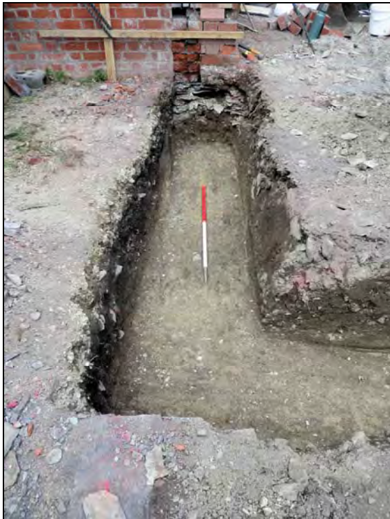
Plate 4. The southwest foundation trench. Scale: 1m. Looking northwest.
