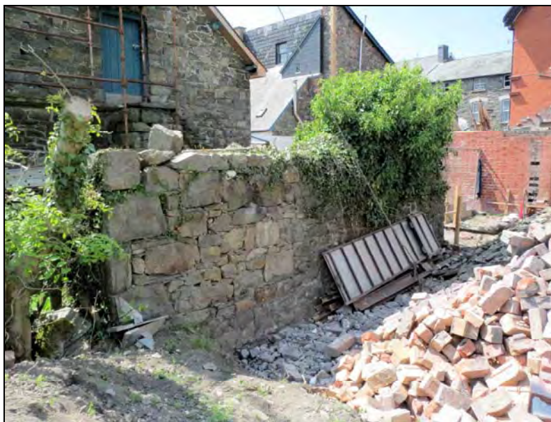
Plate 12. Detail of the stone boundary wall. Looking west.
