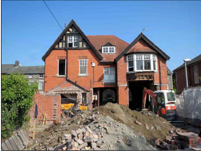
Plate 1. General view of the excavation area. Looking northwest.
