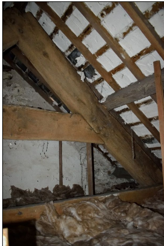
Plate 14: Western principle rafter of one of the trusses
