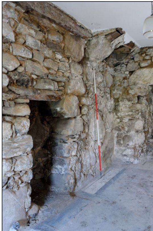
Plate 12: Possible supports for a staircase in the Parlour
