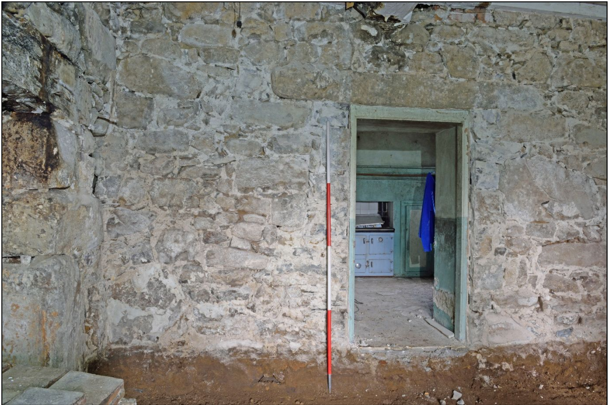
Plate 3: Blocked window in the western wall of the Hall
