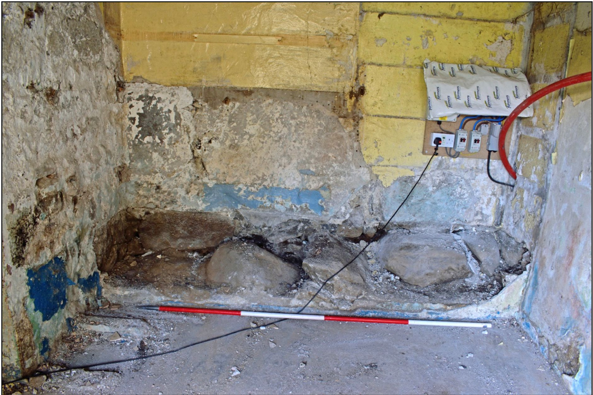
Plate 19: Foundation exposed in the Utility Room.
