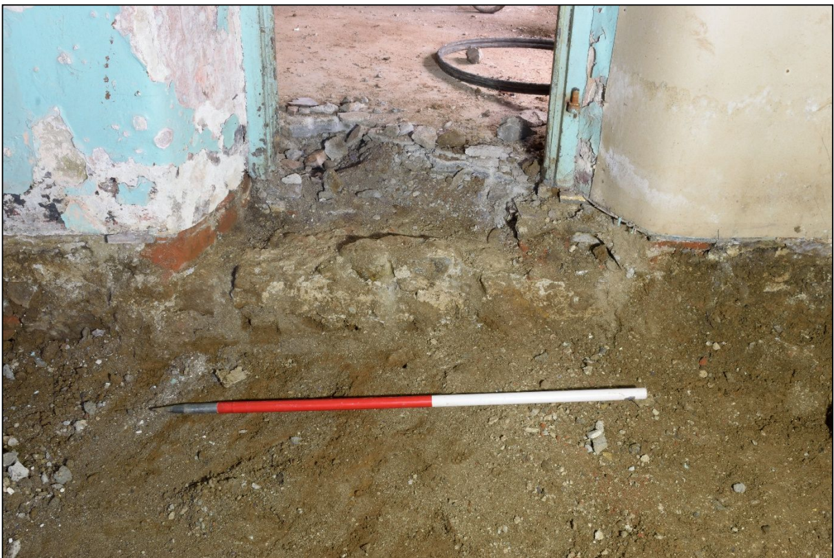
Plate 20: Concrete floors in the Utility Room (from the Kitchen)
