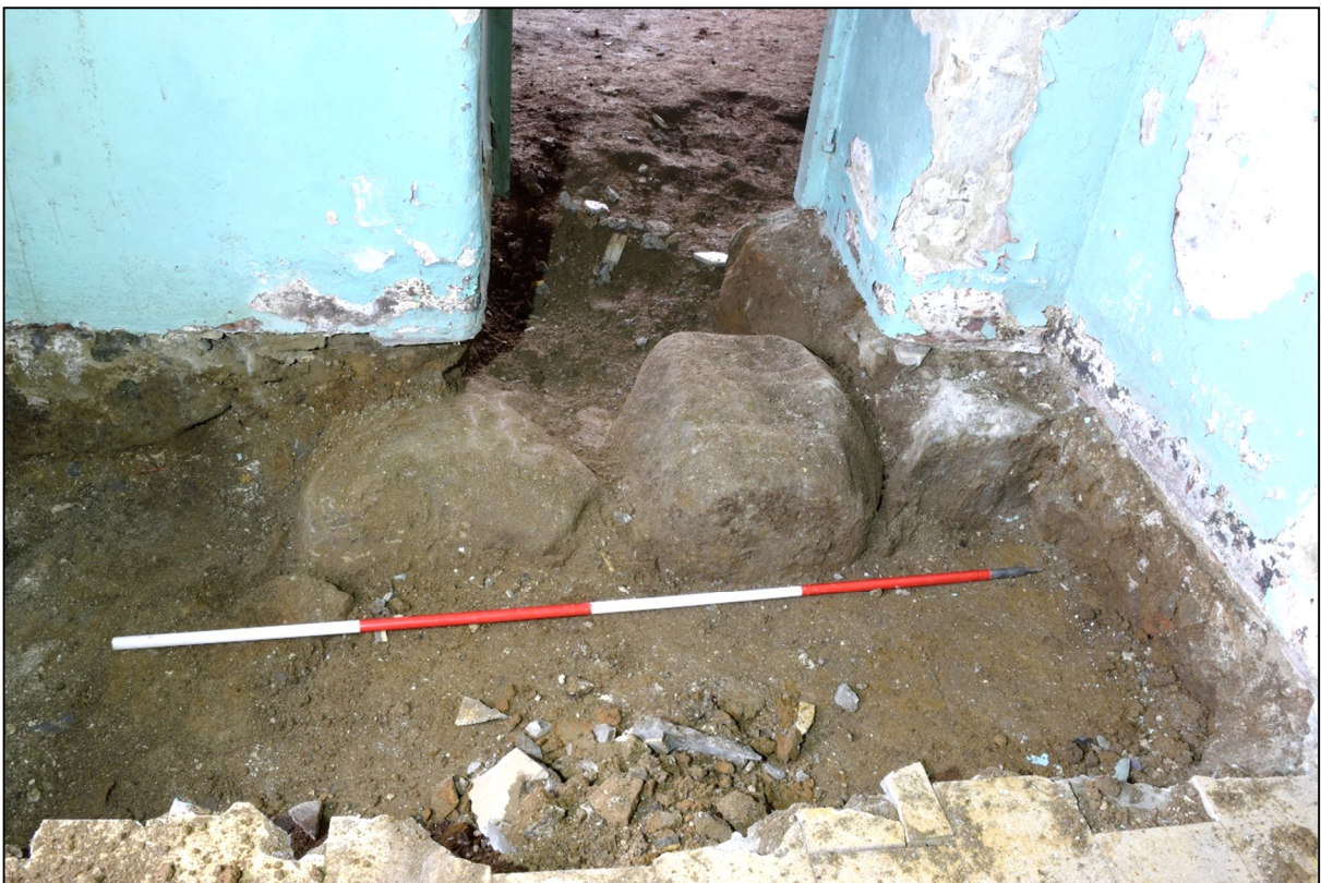
Plate 18: Foundations of the rear wall of the property
