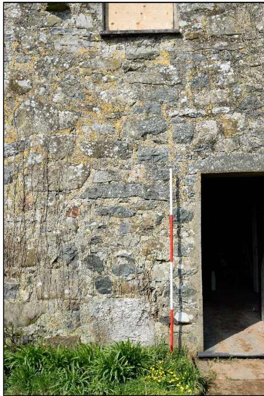
Plate 2: External appearance of blocked door
