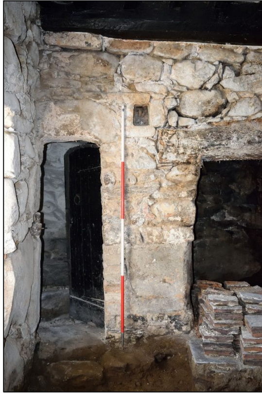
Plate 5: Socket in wall between the fireplace and the intra-mural stairs in the Hall
