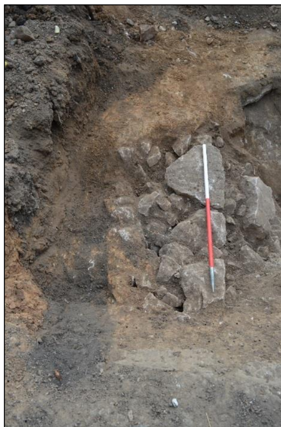
Photo 5. Plan view of the dry limestone wall (07), the wall trench cut (06) into the orange subsoil and the rubble fill (08). CPAT Photo 4078-0032
