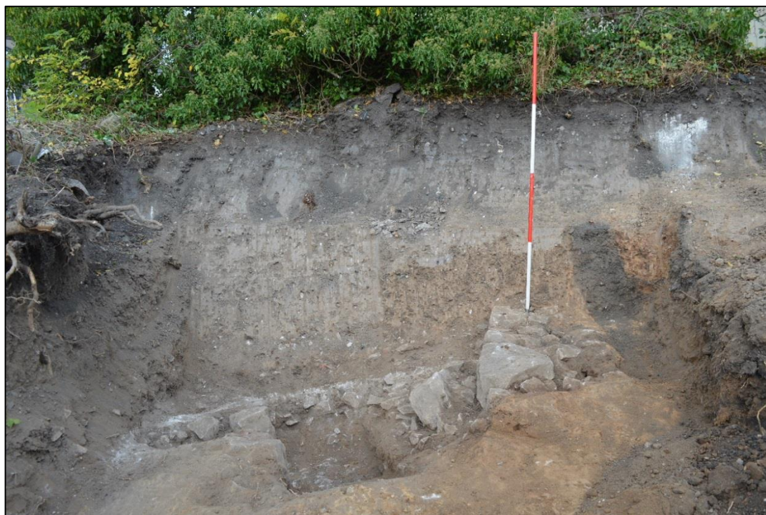
Photo 4. The dry-stone wall (07) beneath the garden soils. Note also the cut of linear (15) to the right of the wall. CPAT Photo 4078-0028
