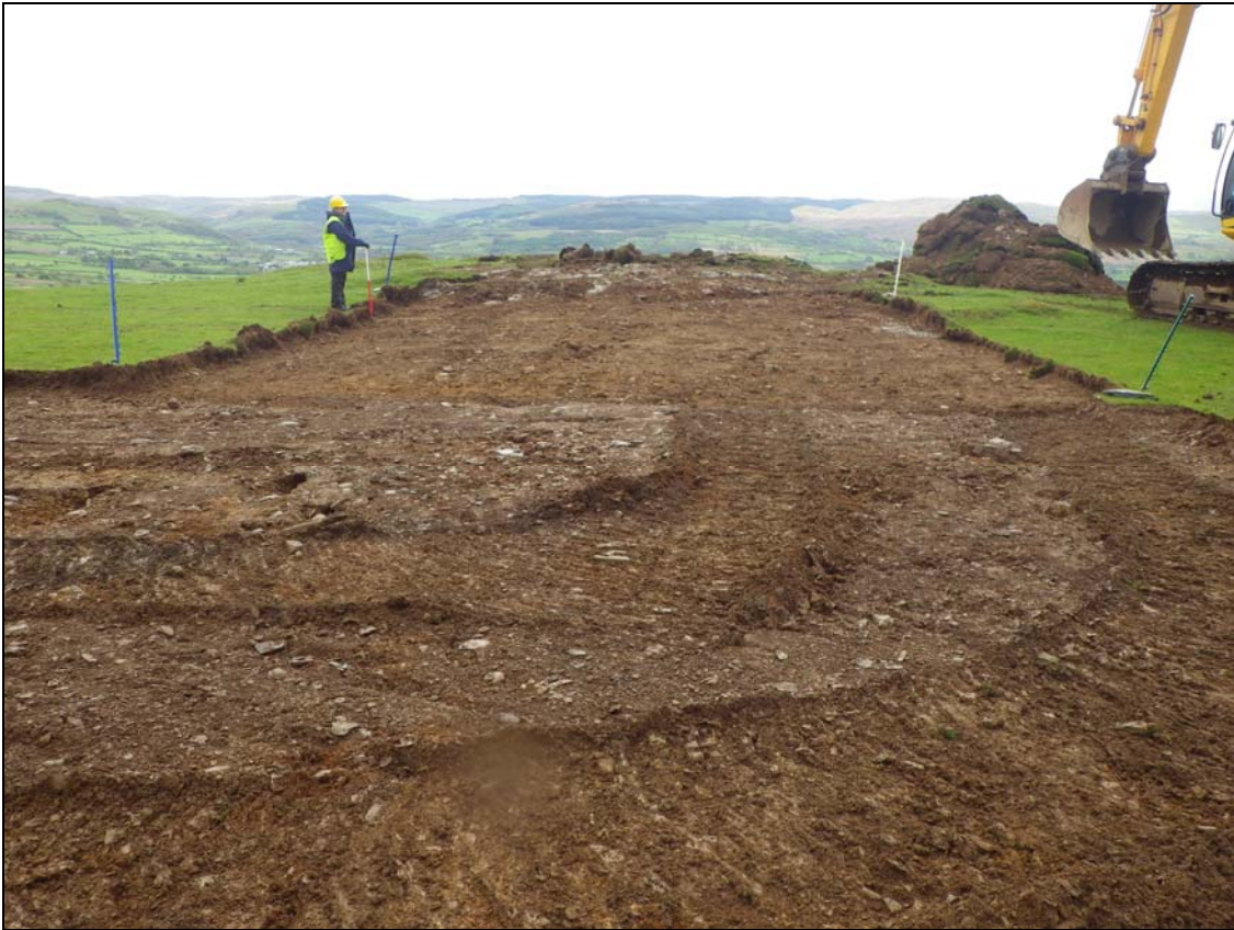
Plate 1: PGU2015_101, After the topsoil, 001, removed from the hardstanding area, looking southwest.
