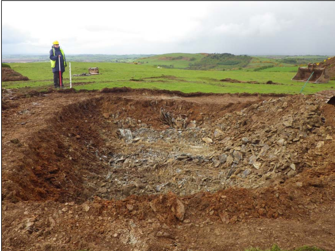
Plate 3: PGU2015_103, the area of the turbine foundation, looking southwest. The natural rock can be seen in the far section, showing how it has been folded and has an uneven interface with subsoil above.
