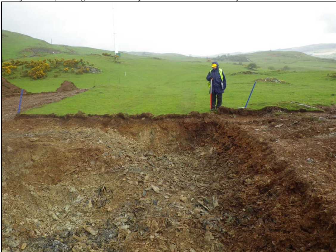
Plate 4: PGU2015_104, the area of the turbine foundation, looking northeast. Again the uneven natural rock surface can be seen in the far section, here it gives a deeper depth of mixed subsoil. This is a natural feature and not created by human interaction
