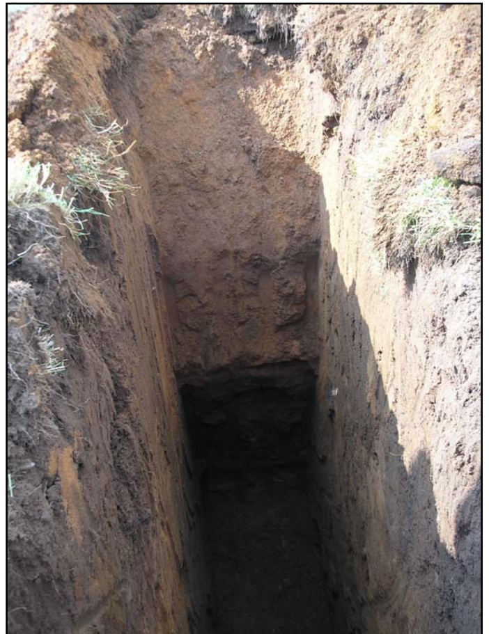
Plate 2 Longitudinal view into TP 6
