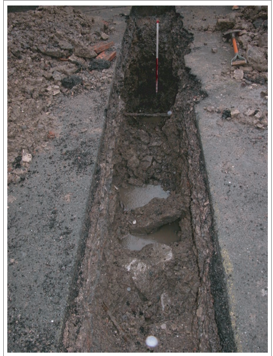
Plate 4: View of Trench TT06, looking north-west. Scale 1 x 1 m.
