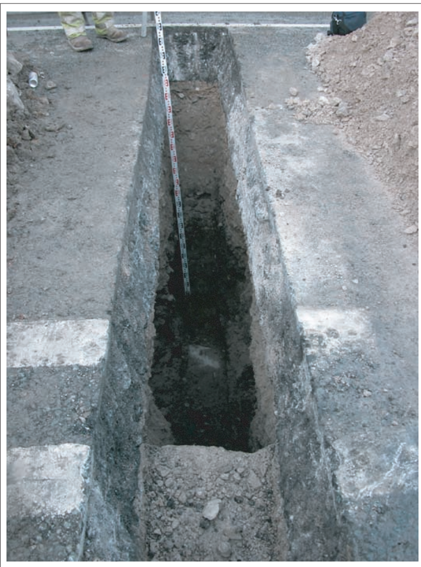
Plate 11: View of trench TT10, looking north-west. Scale 2 m.
