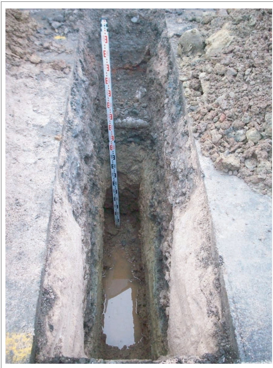
Plate 9: View of extended trench TT09, looking south. Scale 2 m.
