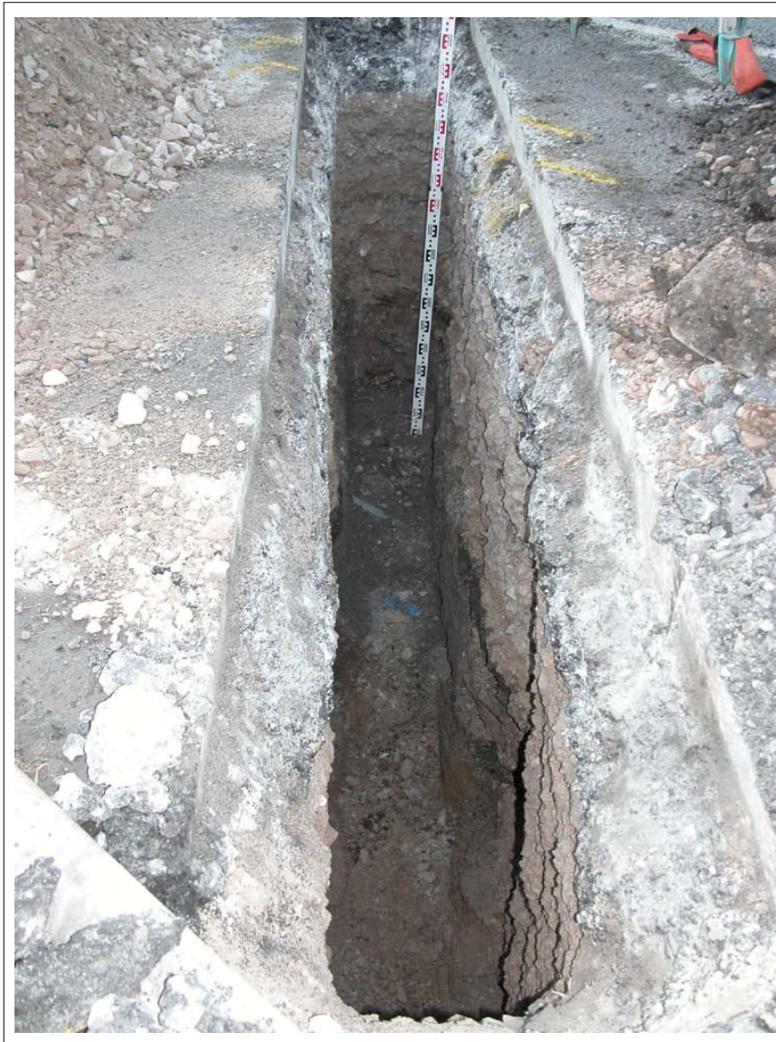
Plate 13: View of trench TT12, looking north-west. Scale 2 m.
