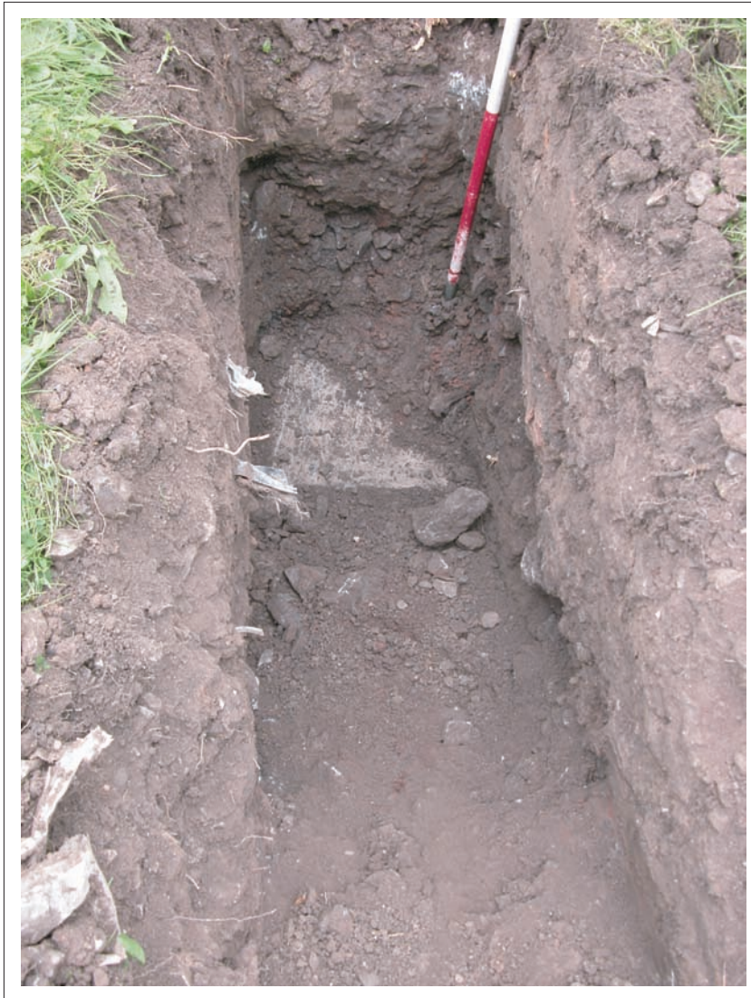
Plate 1: Example view of a trial trench to locate culvert, looking east, scale 1 x 1m.
