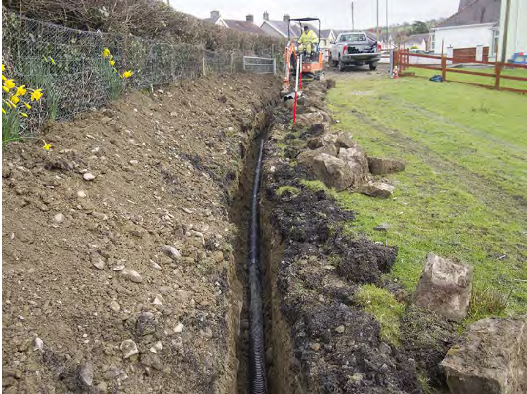
Photo 1: Looking southeast along the cable trench excavations in the easternmost field. The modern road lies to the left of the hedge. Note the large stone from deposit 103. 1m scale.
