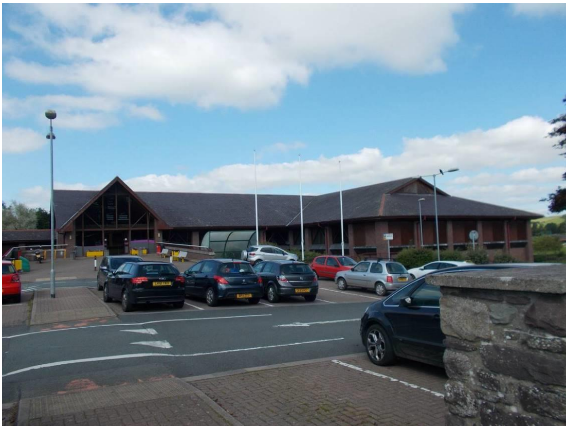
Photo 18: Brecon Leisure Centre building a short distance NE of site.
