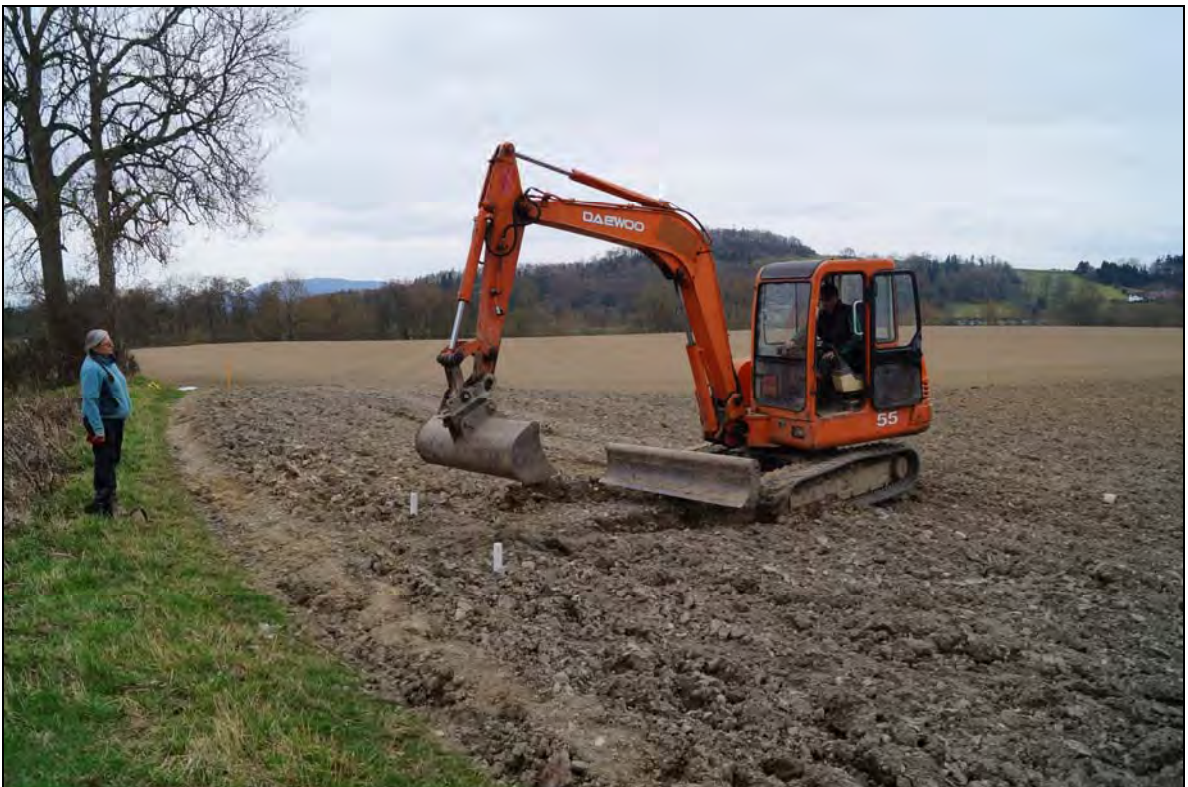
Plate 4: CCH2016_104. Beginning excavation of Trench 1, looking southeast
