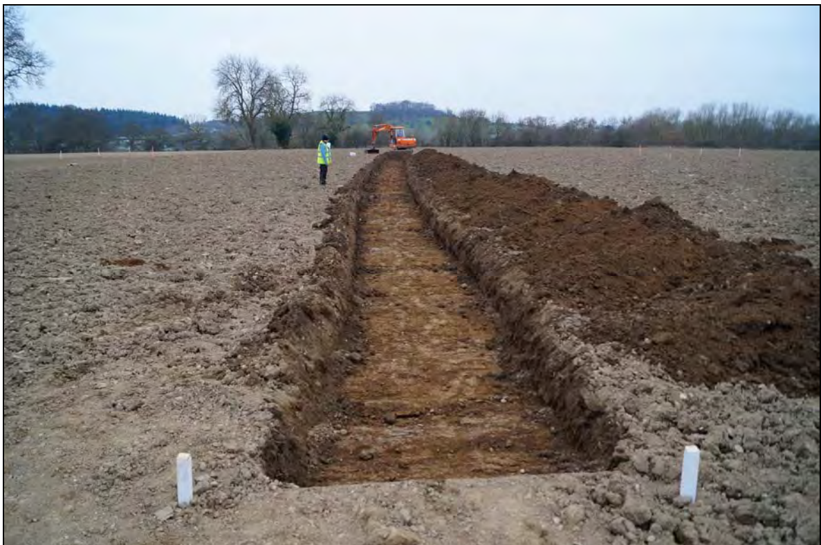
Plate 10: CCH2016_110. Excavated Trench 3, looking southwest.
