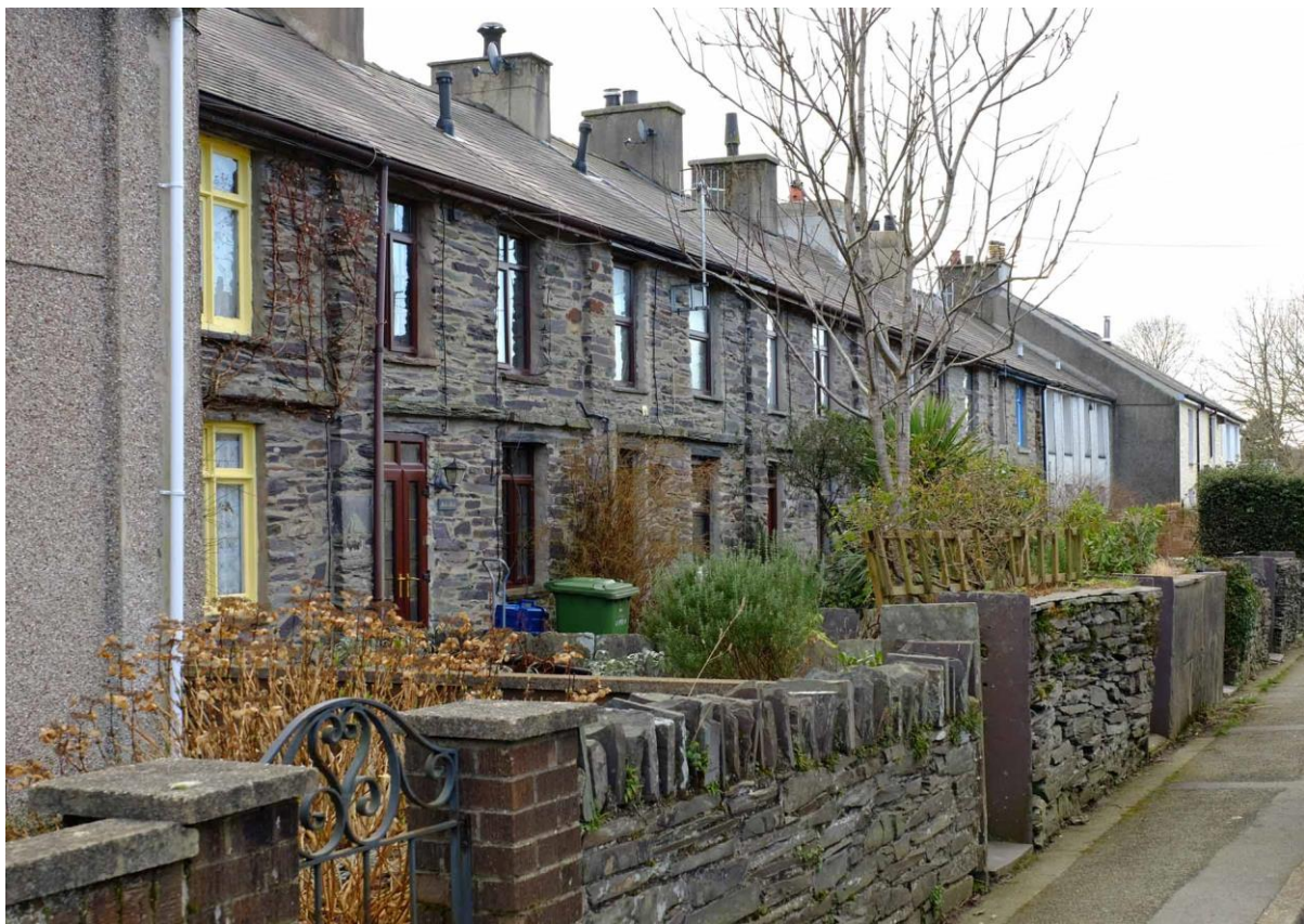
Fig 22 Tai Penyrsedd, Nantlle, with slate garden walls and gate piers of sawn slabs. Note that the houses are articulated with pilaster strips and string course.
