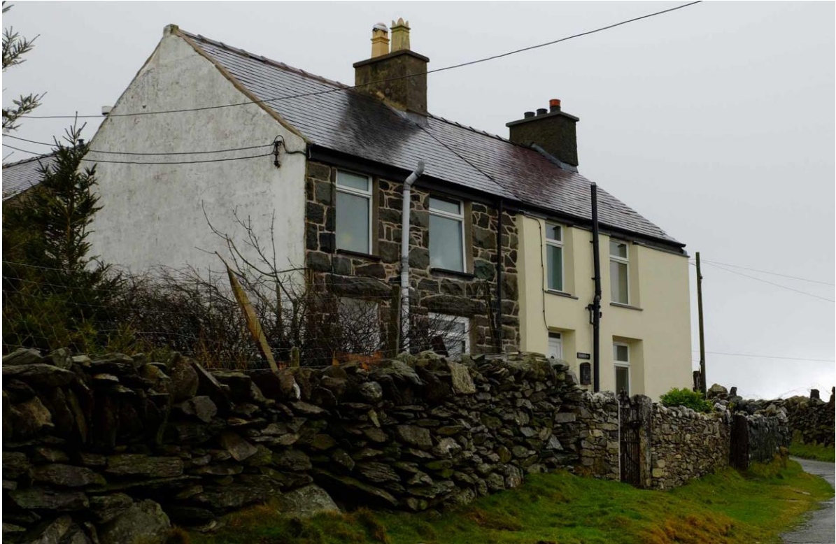
Fig 12 Two-storey houses in Cilgwyn
