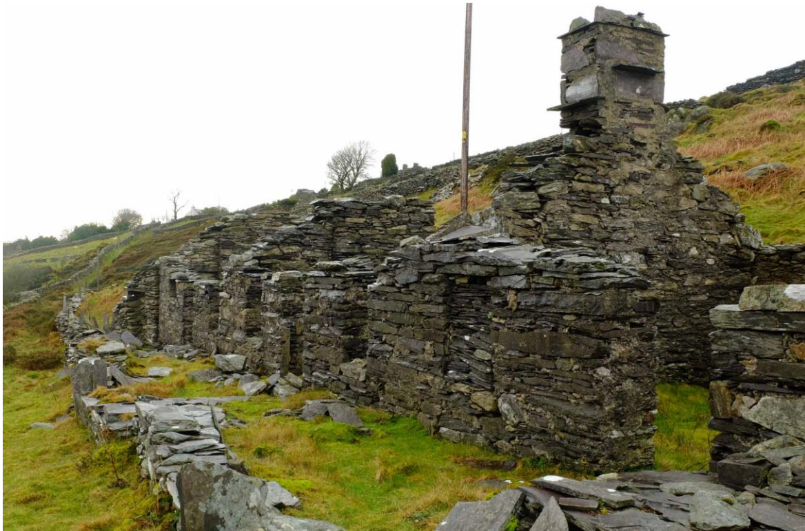
Fig 18 Greenland, Cilgwyn, a row of three single-storey cottages built between 1840 and 1889, constructed mainly of roughly coursed slate blocks from the quarry.
