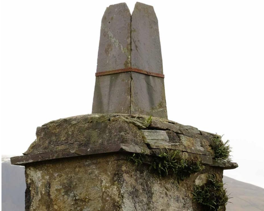
Fig 20 Slate chimney pot, Cilgwyn
