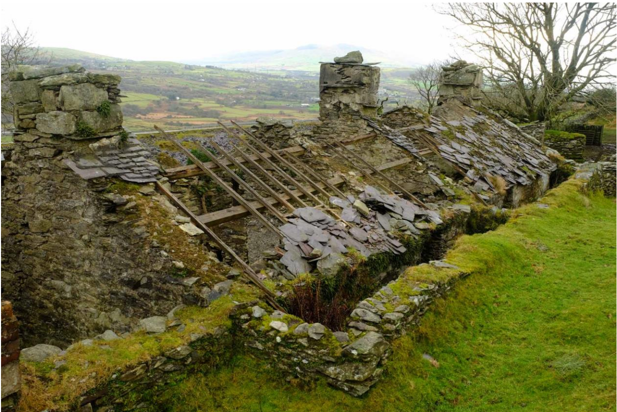
Fig 11 A row of four single-storey cottages at Pen-ffynnon-wen in Cilgwyn, built in the period 1840-1889. The steep bank is retained by a retaining wall and the cottages are offset from it, an unusual arrangement seen elsewhere in North Wales. Note that the chimney stack is constructed of large blocks, larger than the stones in the gable end below it.
