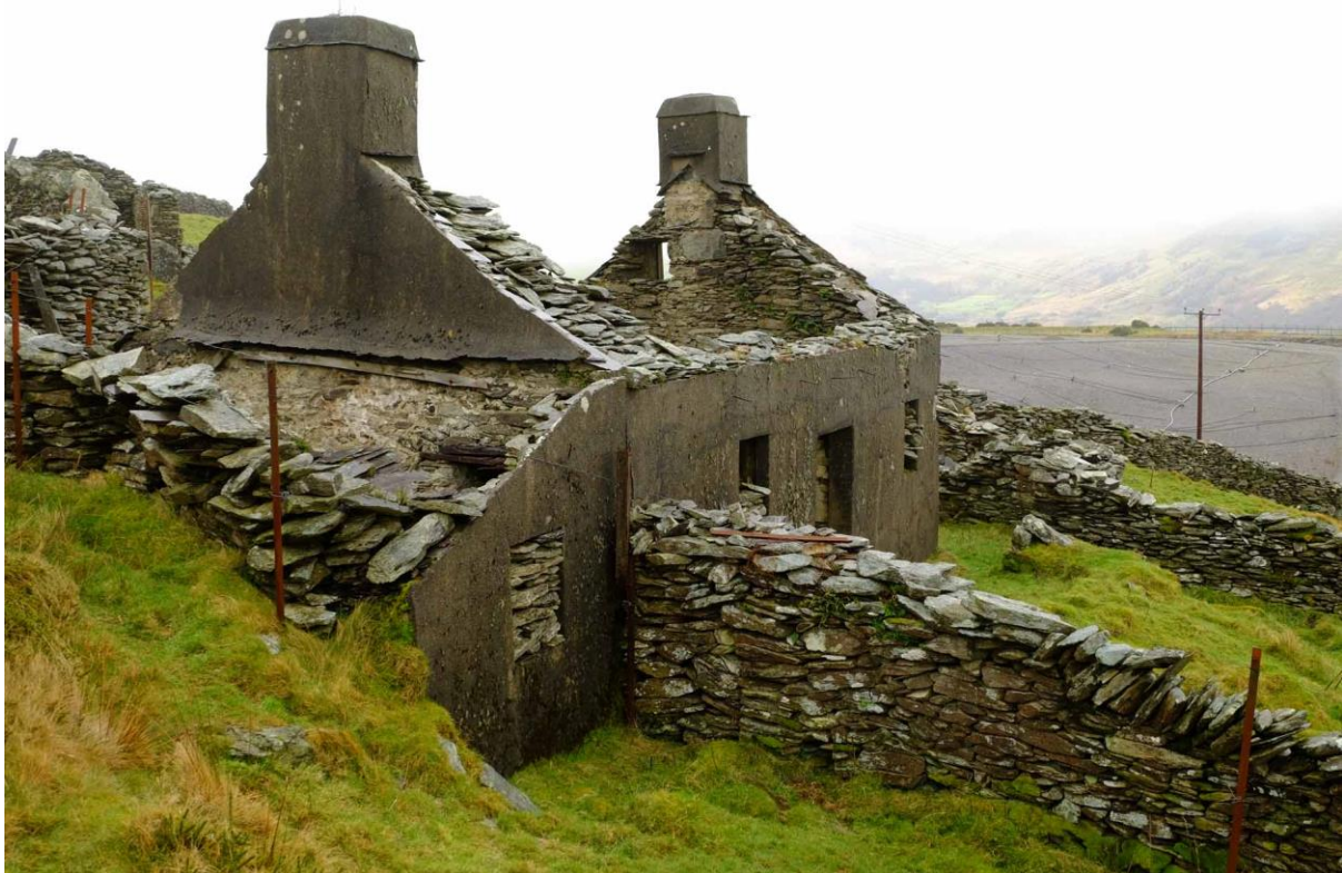
Fig 9 Samaria in Cilgwyn, built by 1840. In the far gable end is a small window that lit the croglofft.
