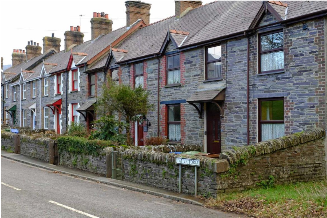
Fig 26 Tai Victoria, Nantlle. The terrace features brick dressings and stacks, and bracketed canopies above the doorways.
