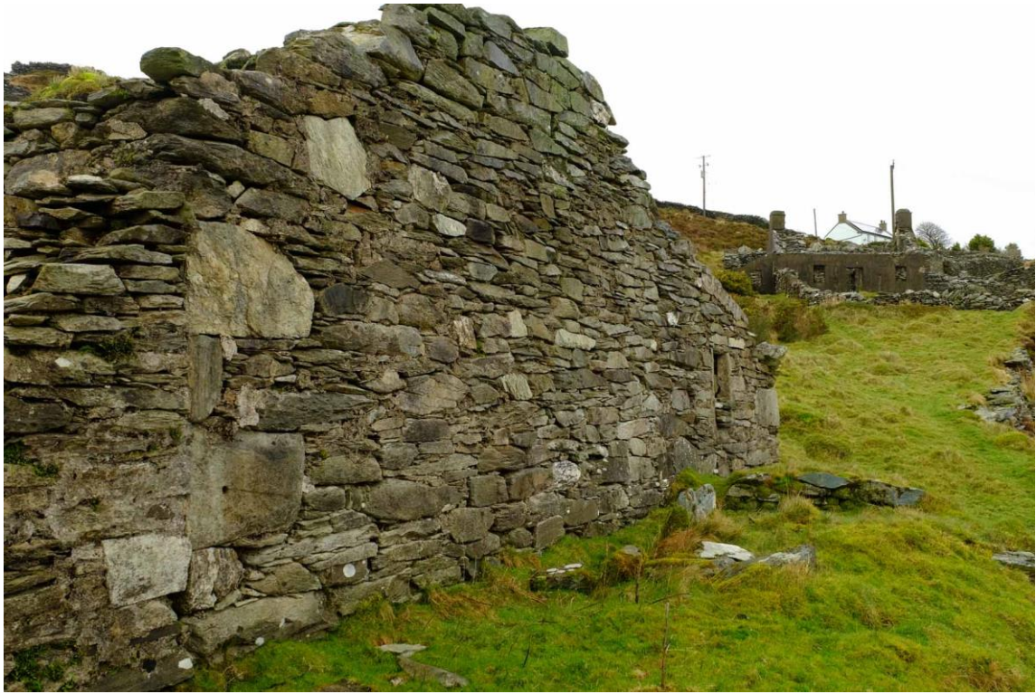
Fig 16 Gable end of a cottage in Cilgwyn, built of field stone of varying sizes, with large quoins.
