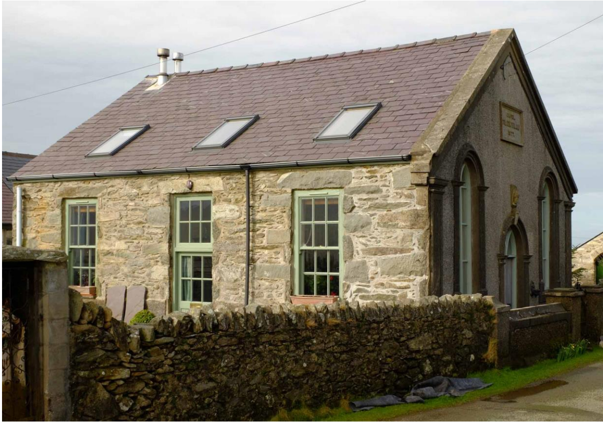
Fig 15 Cilgwyn Independent chapel, rebuilt in 1877. It has a gable-end façade and round-headed windows, characteristic of nonconformist chapels of the latter half of the nineteenth century.
