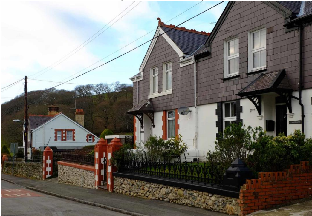
Fig 27 Semi-detached houses opposite Tai Victoria, clearly of superior social status to the quarrymen's houses. The houses have the most prominent display of slate hanging in the village.
