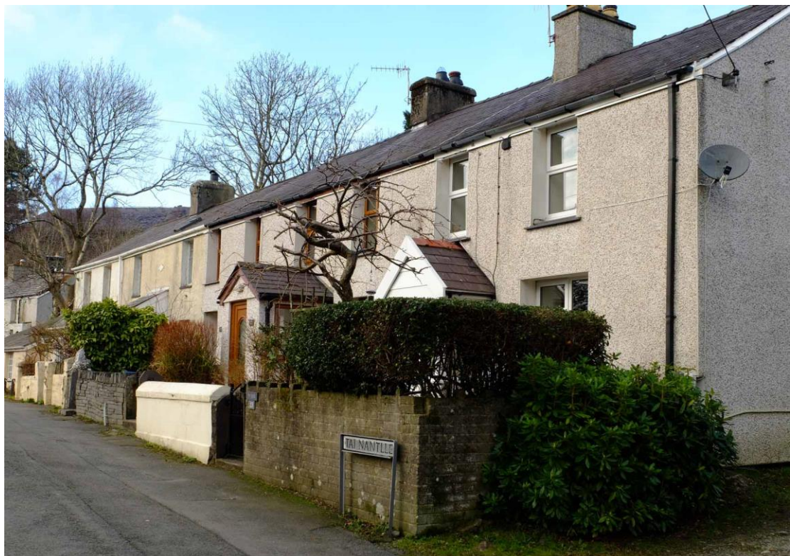
Fig 34 Tai Nantlle, a terrace built in two phases, with a mixture of rebuilt and rendered garden walls.
