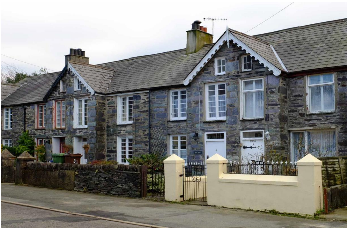
Fig 30 Tai Baladeulyn, a terrace of mirrored pairs under gables with barge boards.
