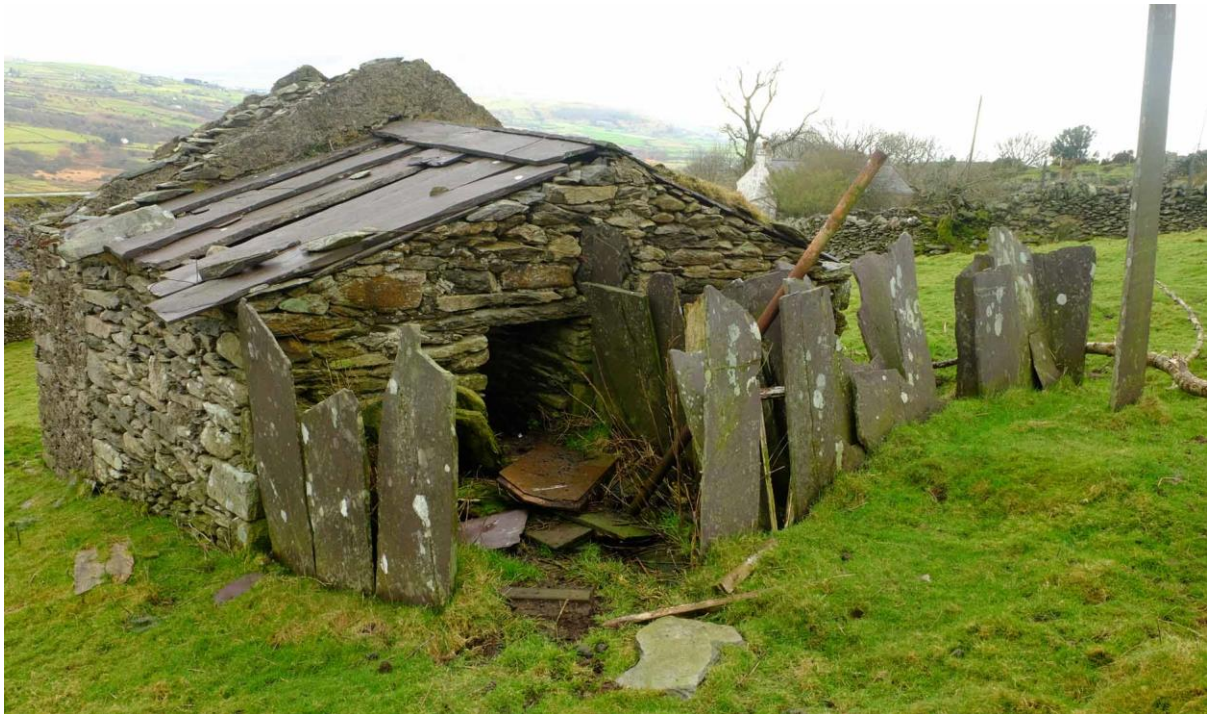
Fig 21 Slate slabs used in a pigsty at Pen-ffynnon-wen, Cilgwyn.
