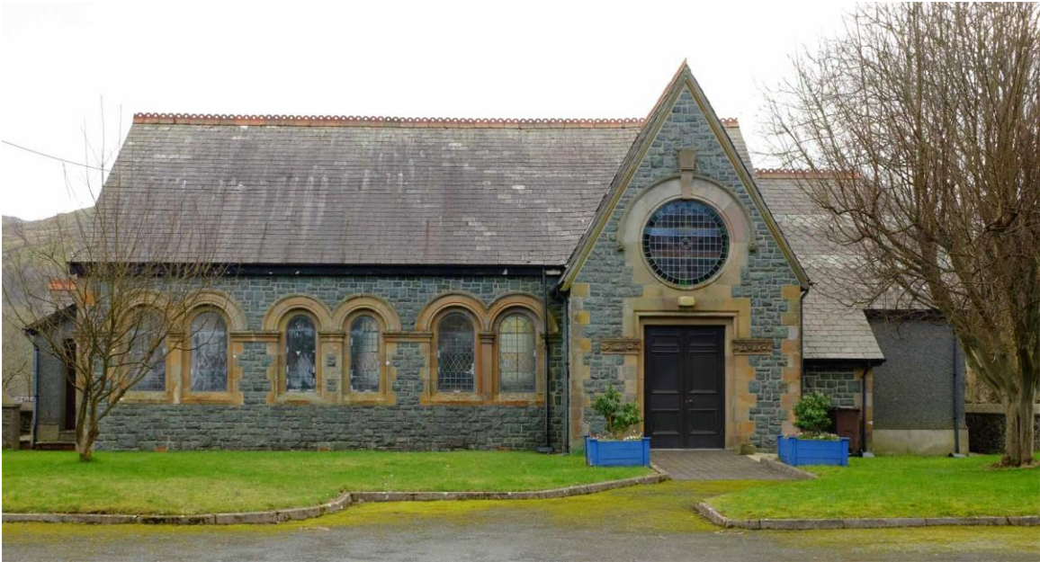
Fig 23 The vestry at Capel Baladeulyn, built of snecked quarried stone with sandstone dressings.
