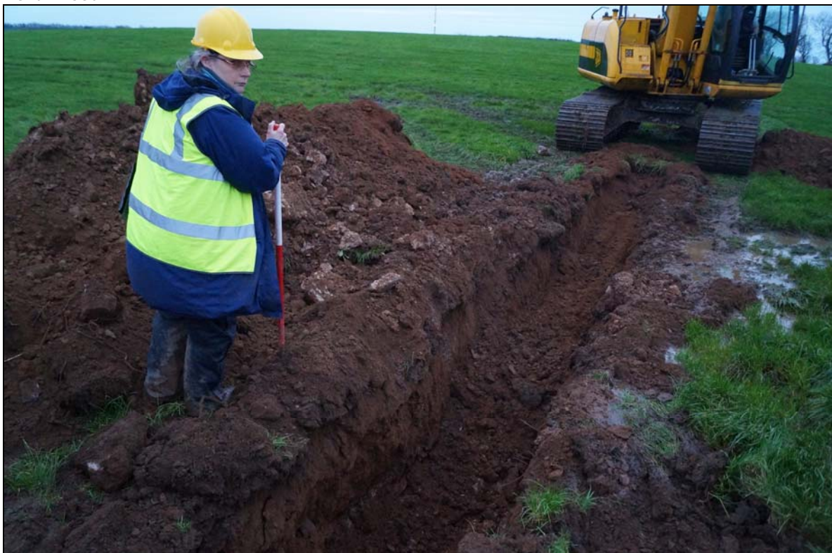
Plate 14: MYW2015_114, excavated cable trench, looking southwest
