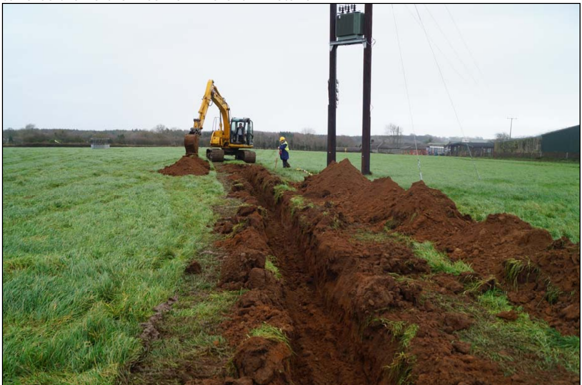
Plate 8: MYW2015_108, excavating cable trench, looking east.
