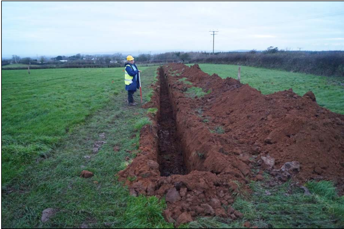
Plate 13: MYW2015_113, excavated cable trench in western field, looking north northwest.
