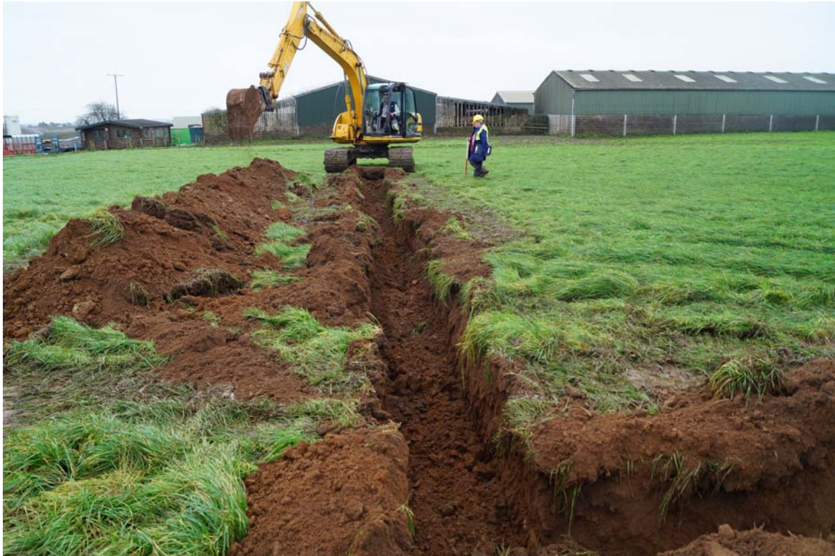
Plate 9: MYW2015_109, excavating cable trench, looking southeast.
