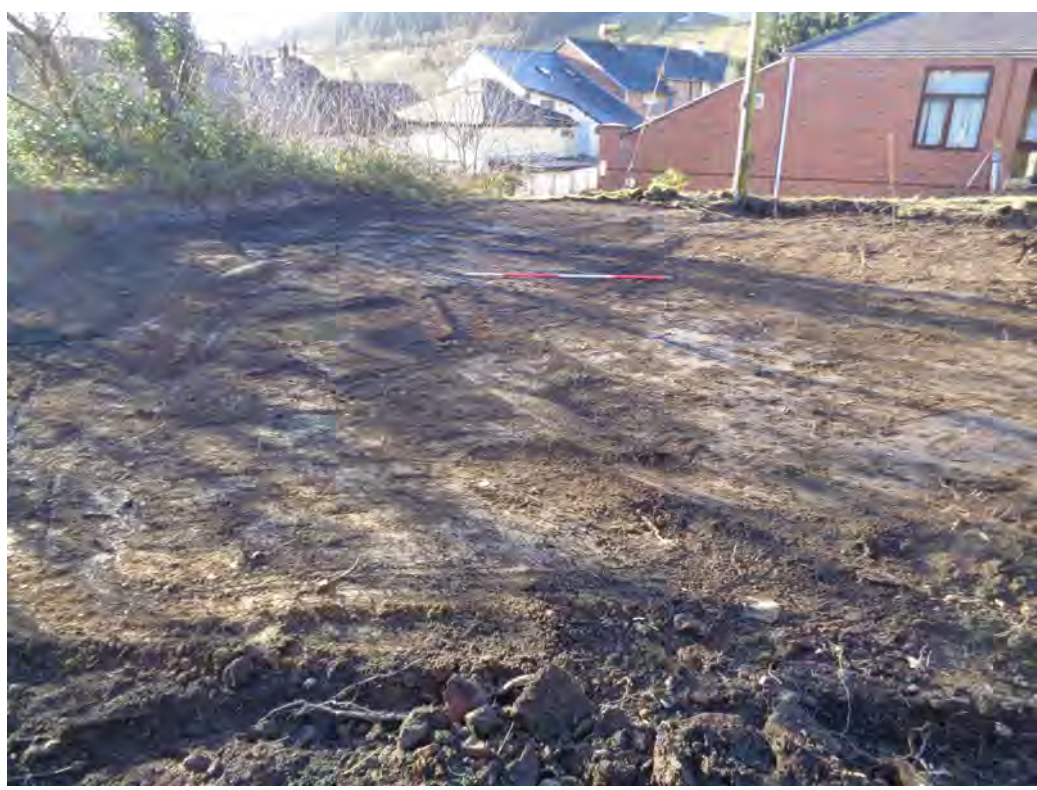
Plate 5. Site after levelling ground, looking south-west. Scale 2m
