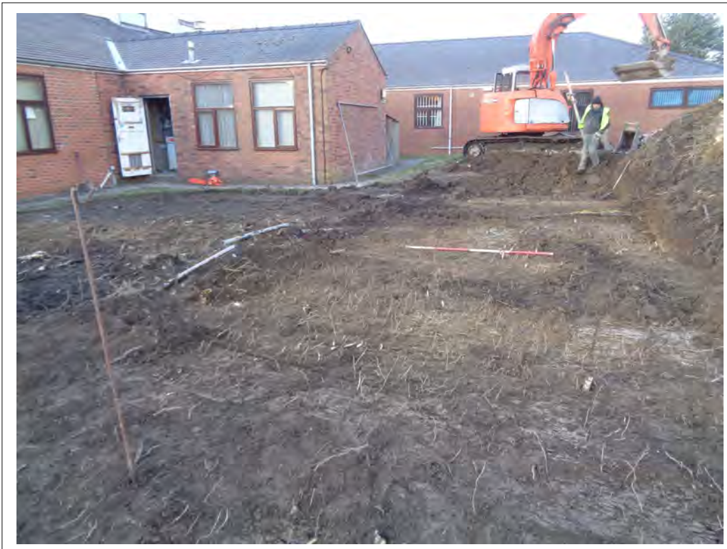
Plate 6. Site after levelling ground, looking north-east. Scale 2m
