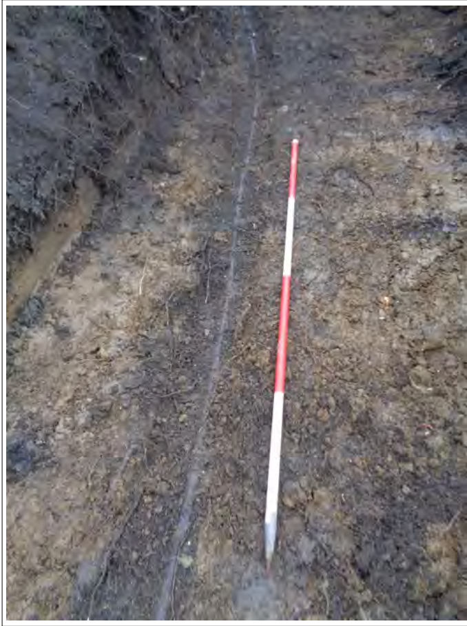
Plate 1. Exposed power cable, looking south. Scale 2m
