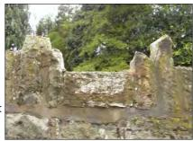
will increase the rate of deterioration of sandstone in particular. Lime mortar would have been used historically and should be used in place of a hard cement mortar.
