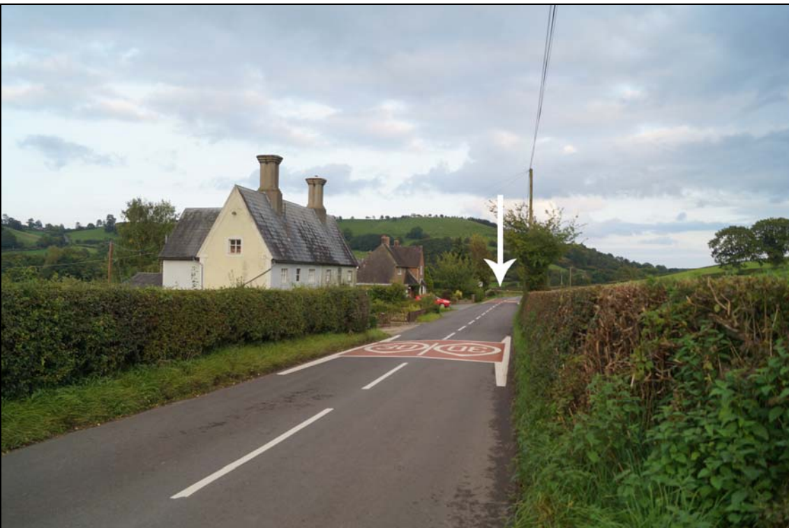
Plate 4: A view looking east along the B4389 towards the proposed development site, which is marked with an arrow. The Concrete Cottages (ID numbers 11 & 19) stand to the left of the road.
