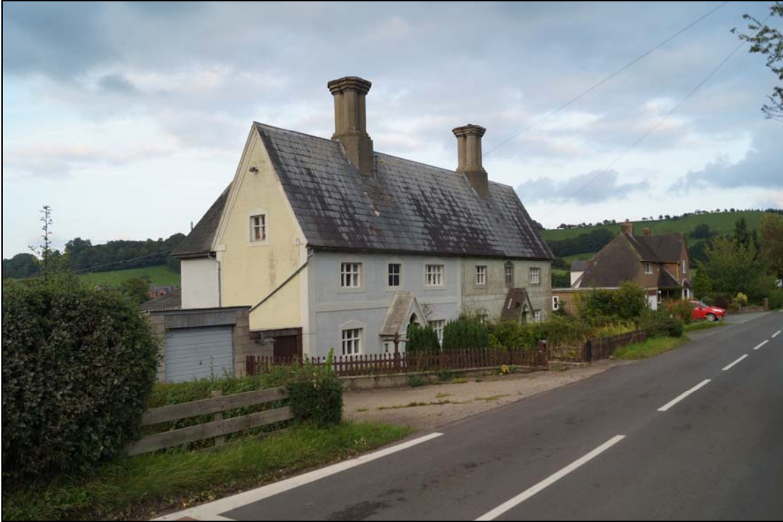
Plate 5: A view of the Concrete Cottages (ID number 11 & 19) looking northeast from the B4389 road. The proposed development would not interfere with this key view of the listed building.
