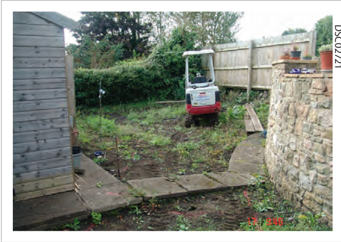
Plate 01: Position for trench 1
