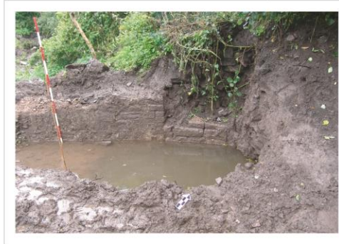
Plate 06: Test pit 4, road revetment
