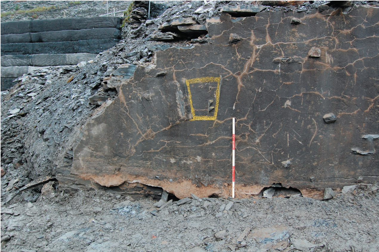
Plate 14 Site 3(32) Road causeway: Blocked incline arch in E side of causeway
