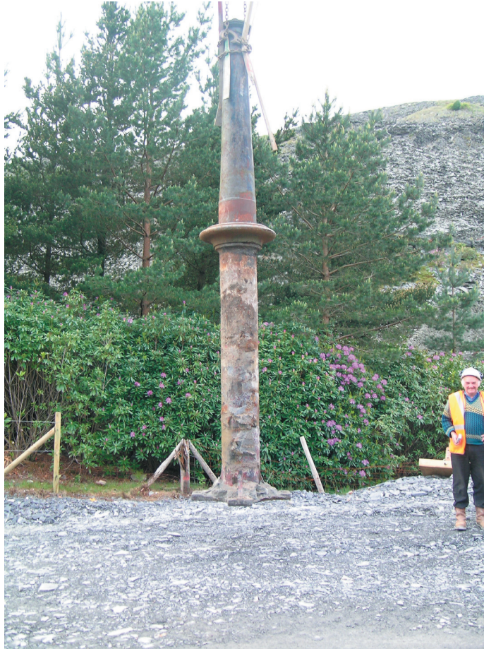
Plate 9 Site 1(13) The crane pillar
