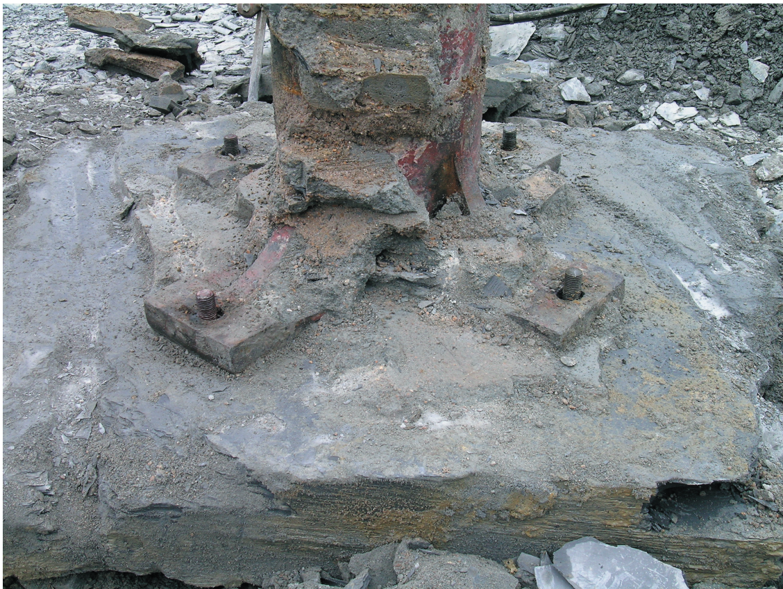
Plate 10 Site 1(13) The crane pillar: flanges and block
