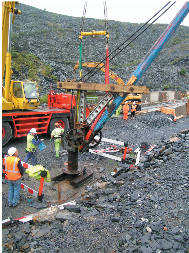
Plate 8 Removal of the upper part of Crane 3(13)
