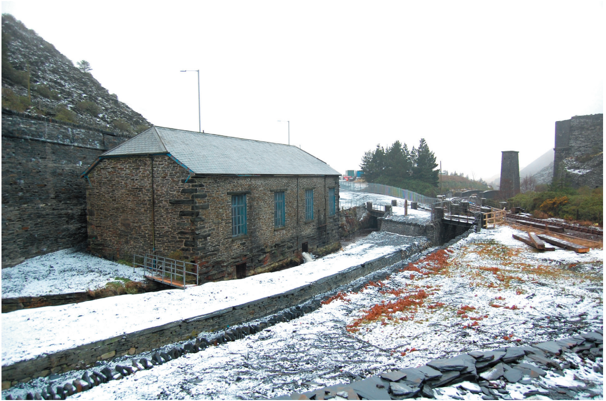
Plate 23 Llechwedd exchange sidings after reinstatement
