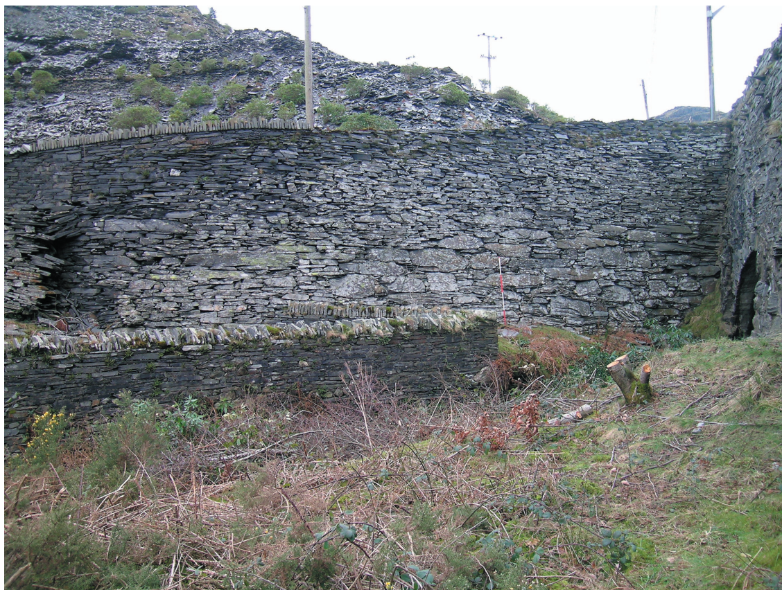
Plate 6 Site 3(17) Slate retaining wall
