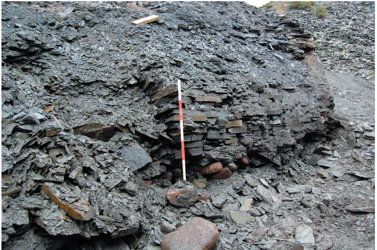
Plate 15 Site 3(5) incline tunnel after removal of road causeway, joint in masonry
