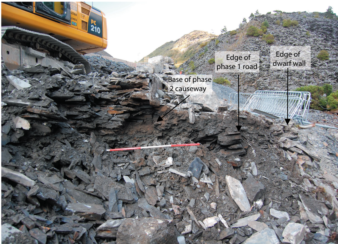
Plate 13 Site 3(32) Road causeway: Section through causeway and phase 1 road, N of Barlwyd tunnel
