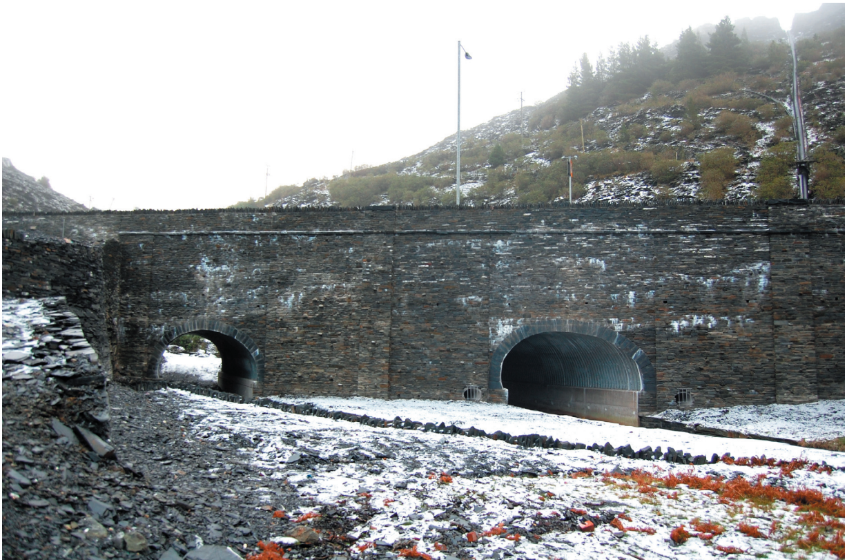
Plate 24 The replacement road causeway, west side
