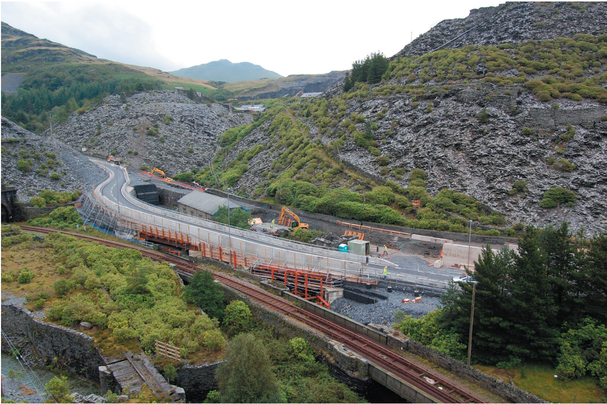
Plate 19 The temporary diversion
