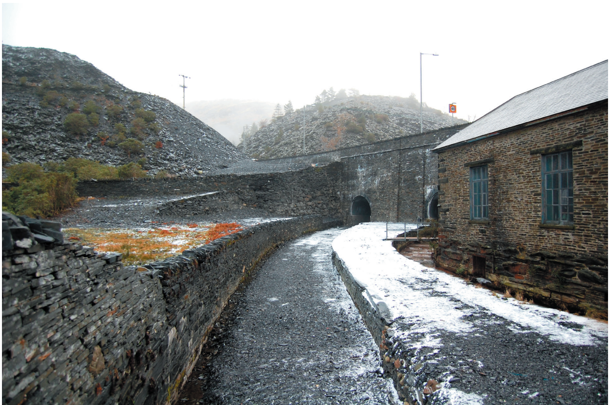
Plate 20 Llechwedd Quarry to Ffestiniog Railway Link 3(16). Trackbed after reinstatement
