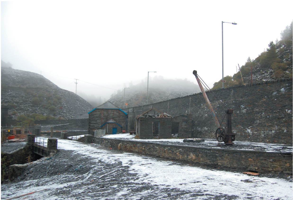
Plate 22 Llechwedd exchange sidings after reinstatement
