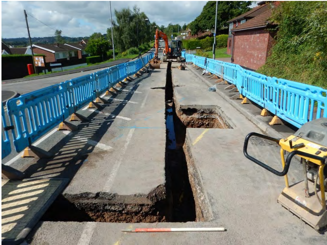
Photo 1: View west of the excavations along Lodge Road (Phase 1). 1m scale.
