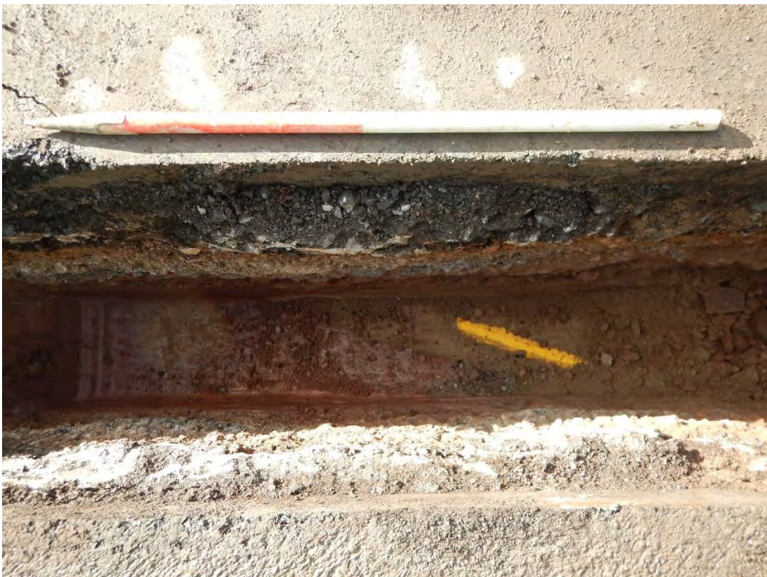
Photo 8: View in plan of Lodge Road (Phase 1) excavation. 1m scale.
