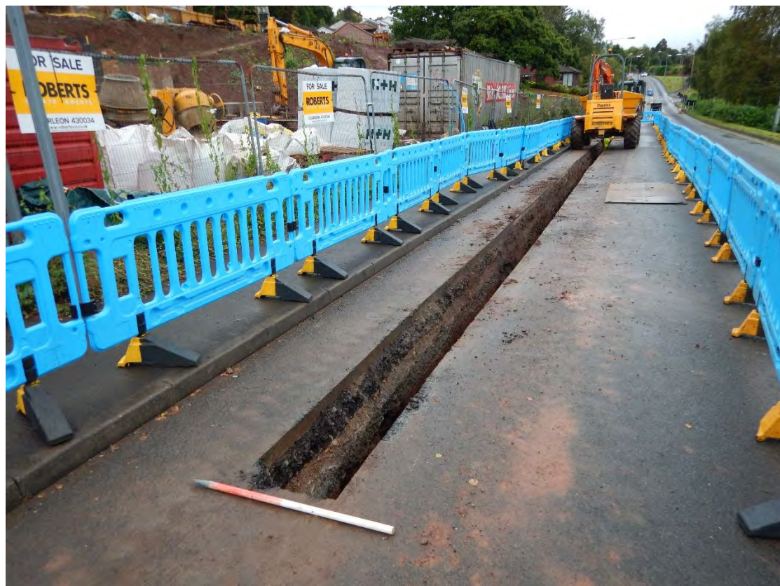
Photo 2: View northeast of the excavations along Lodge Road (Phase 1). 1m scale.
