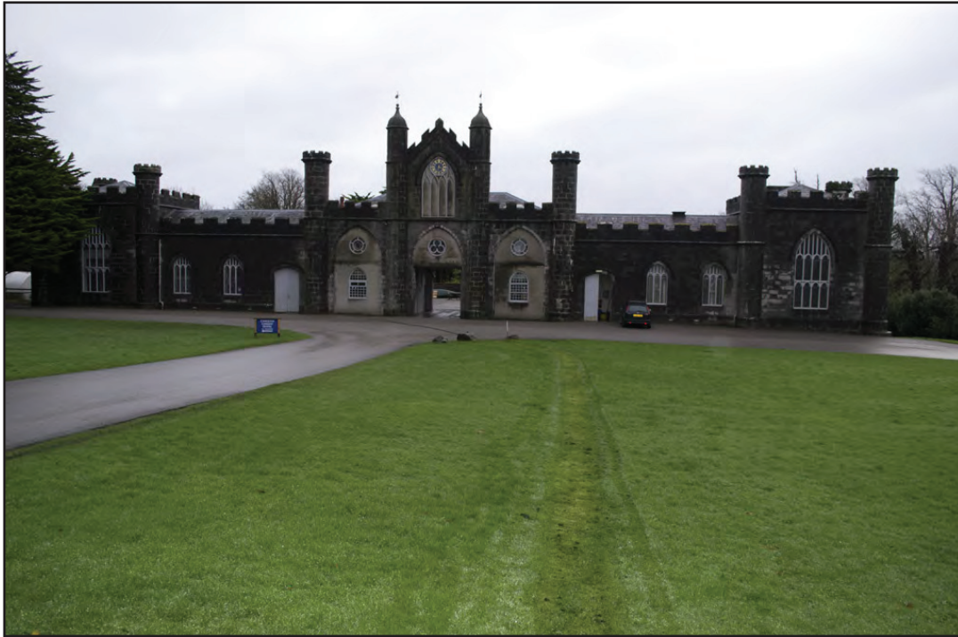
Plate 5: General view along cable route from parkland towards stable block; scale: 1x1m (archive reference: G2542_005).
