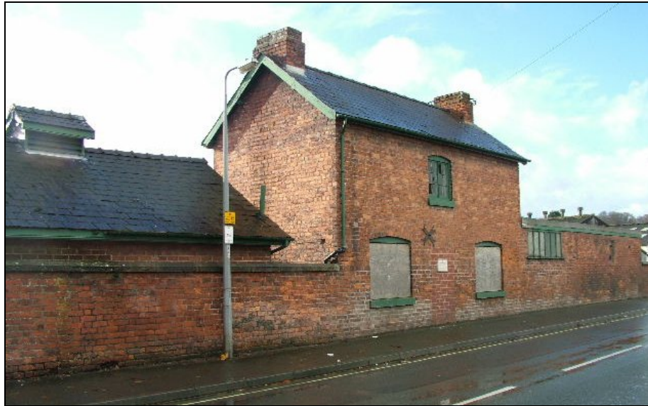
Fig. 3 The former Smithfield office and stables viewed from the north-east. Photo CPAT 2989-0059
