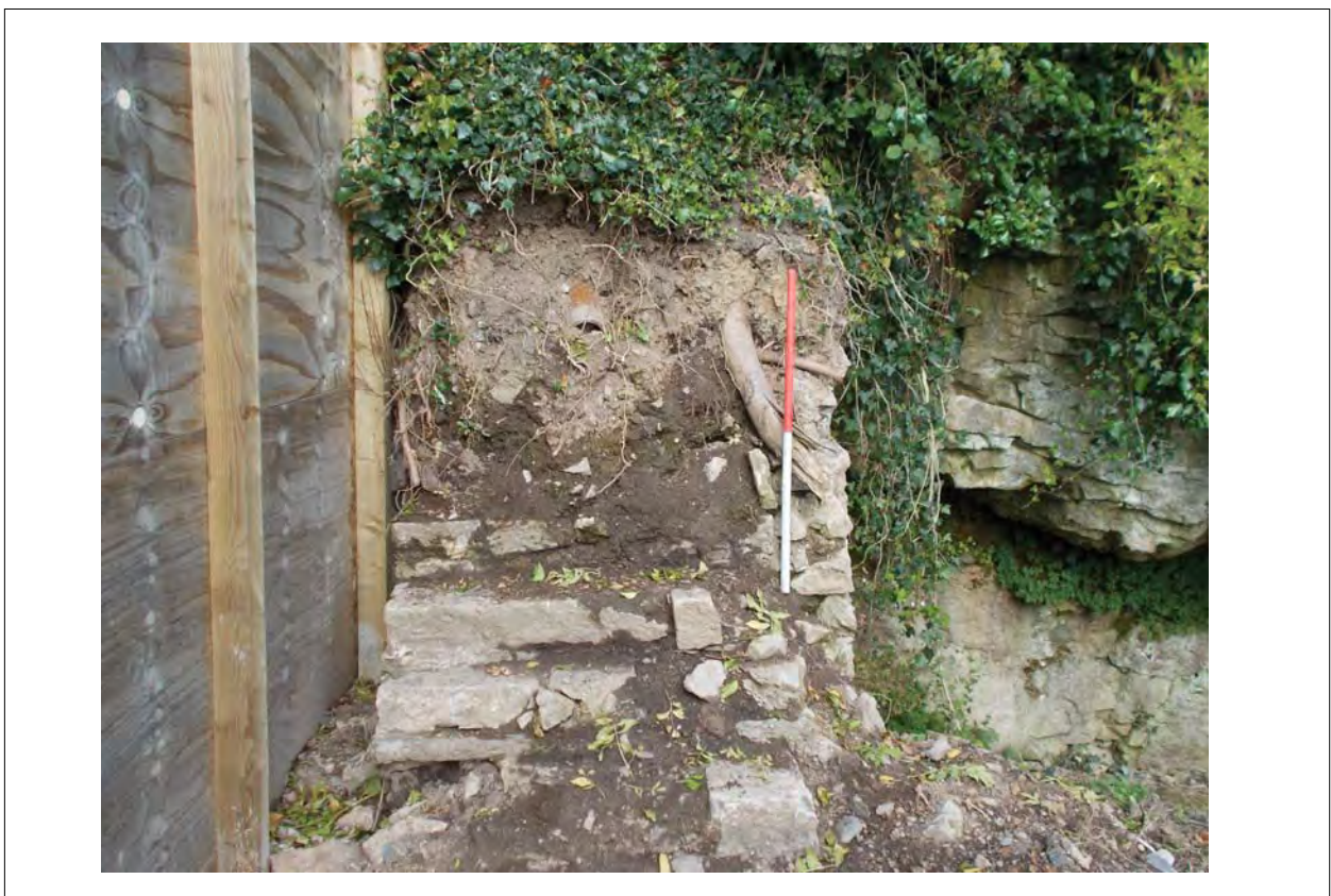
Plate 22: View north east toward north west wall buttress
