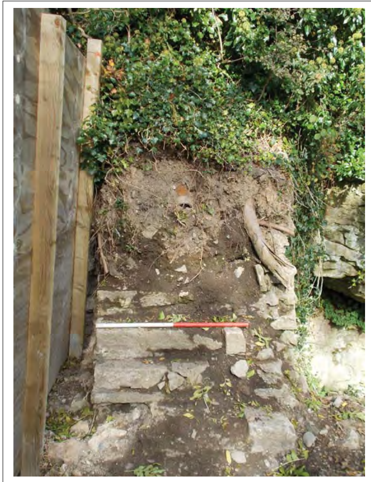
Plate 21: View north east toward north west wall buttress
