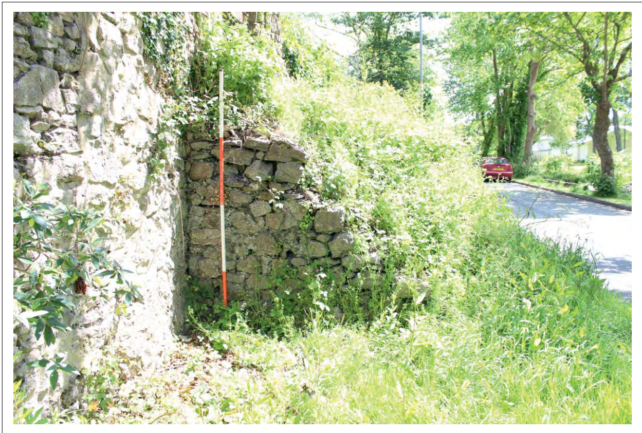
Plate 5: View south east toward entrance ramp retaining wall
