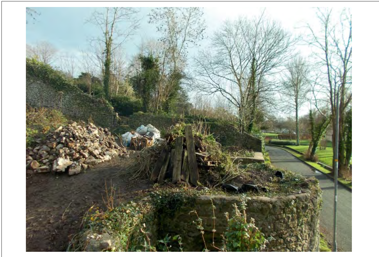
Plate 39: View south east toward east wall
