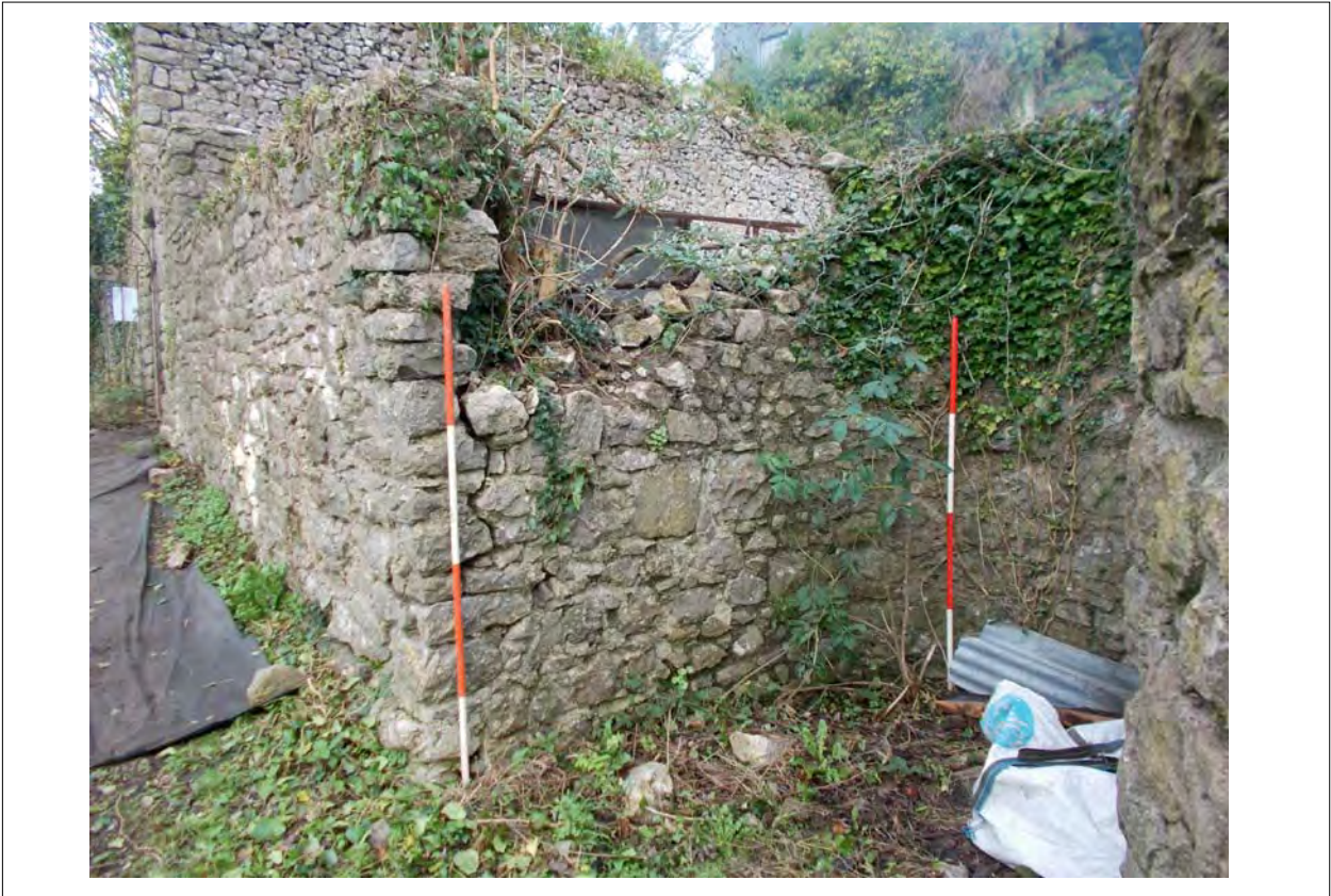
Plate 11: View north toward south external wall
