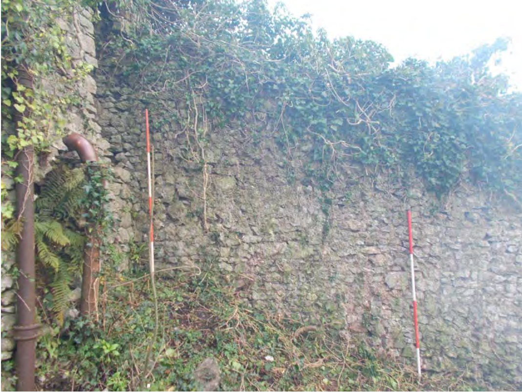
Plate 41: View south east toward east wall
