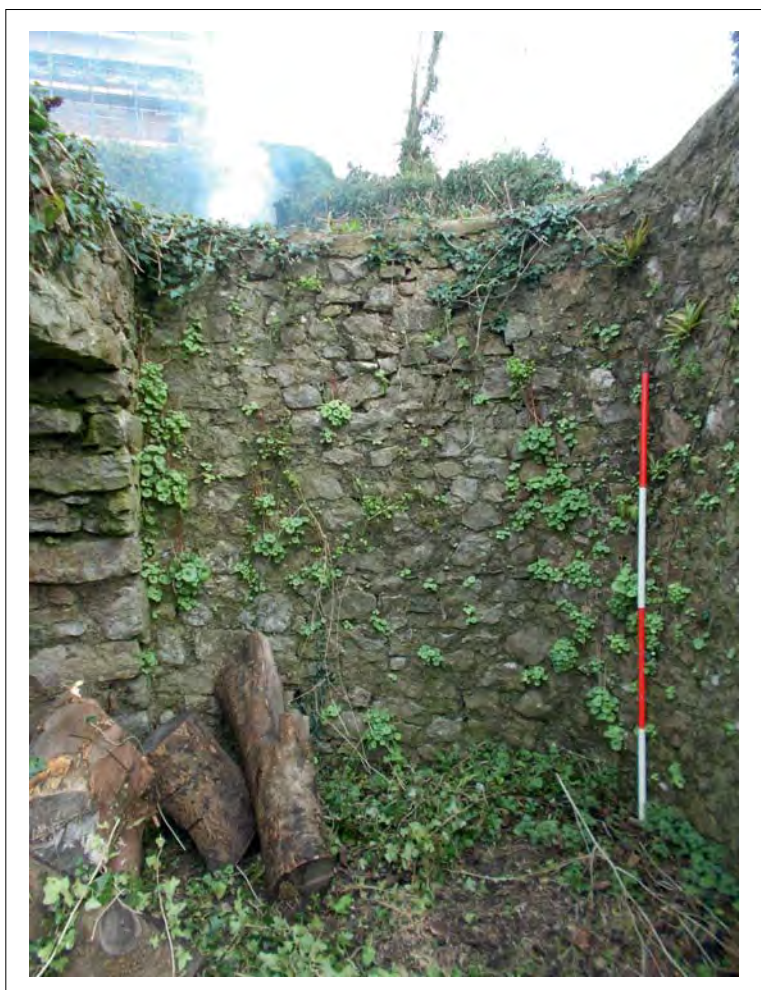
Plate 14: View north east toward south external wall
