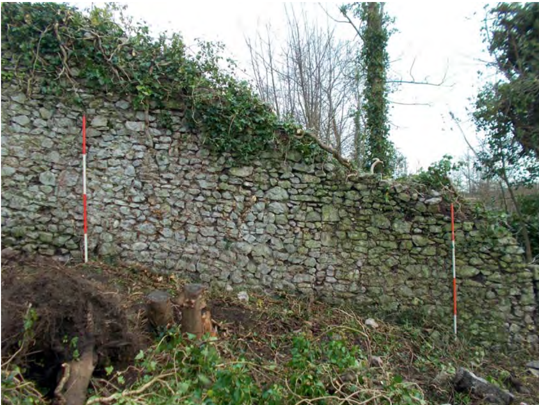
Plate 44: View south east toward east wall
