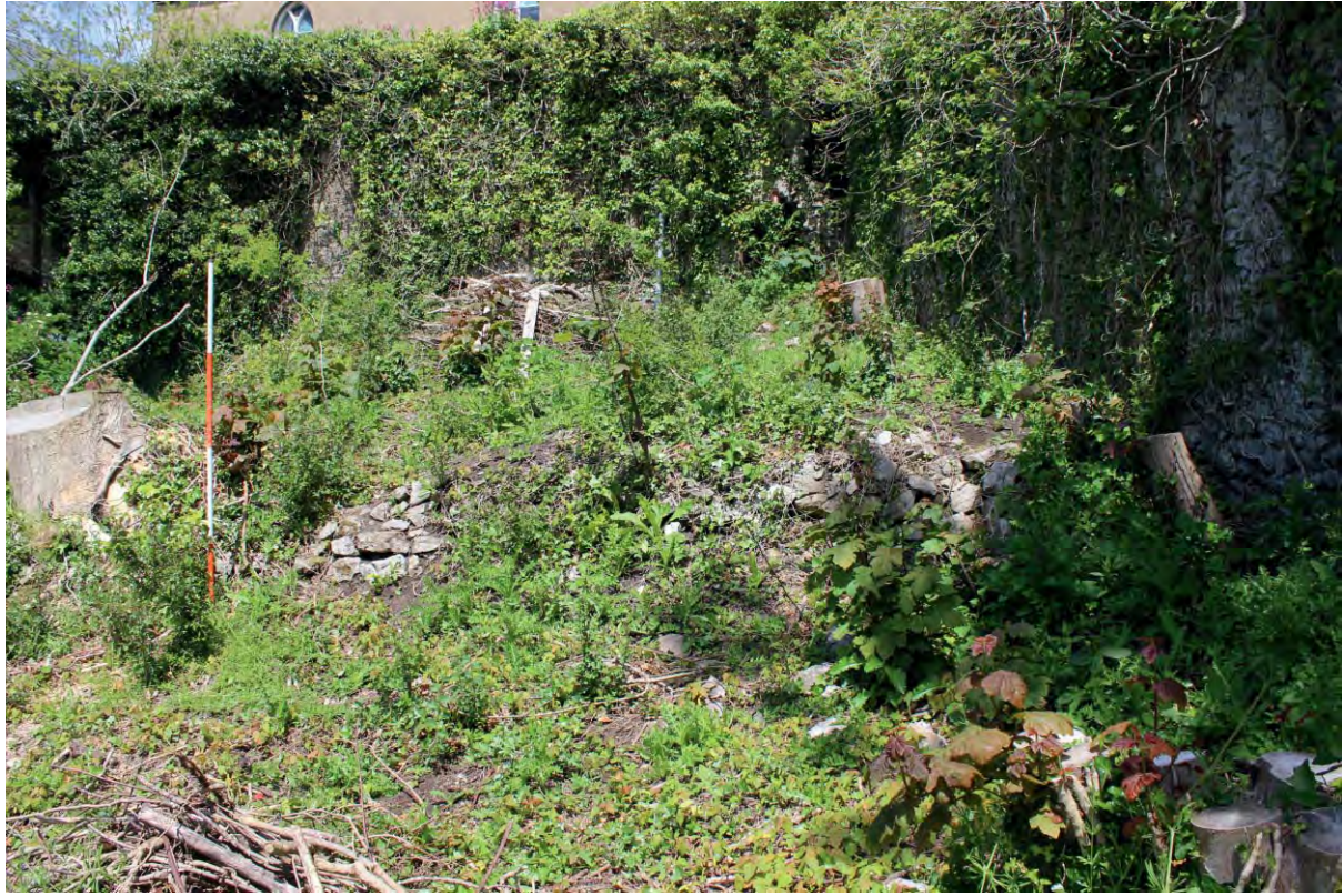
Plate 35: View north east toward stone terrace walls
