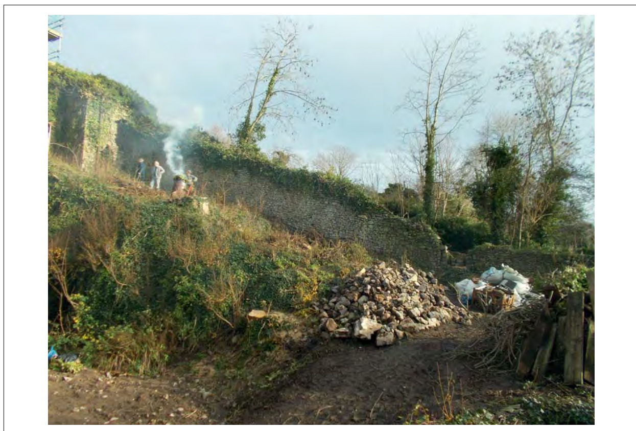
Plate 40: View south east toward east wall
