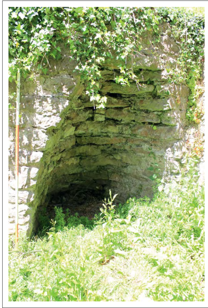
Plate 9: View west toward lime kiln drain hole
