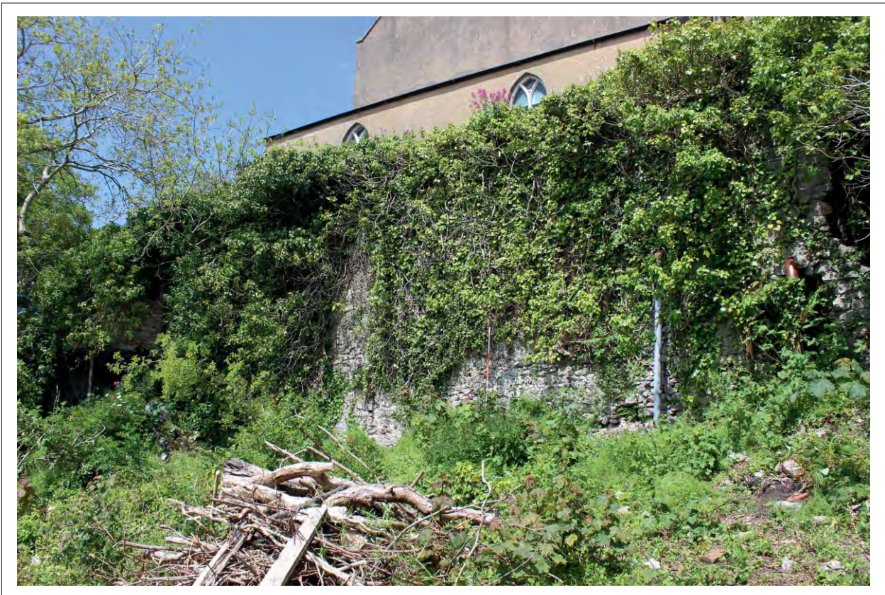
Plate 30: View north toward north wall
