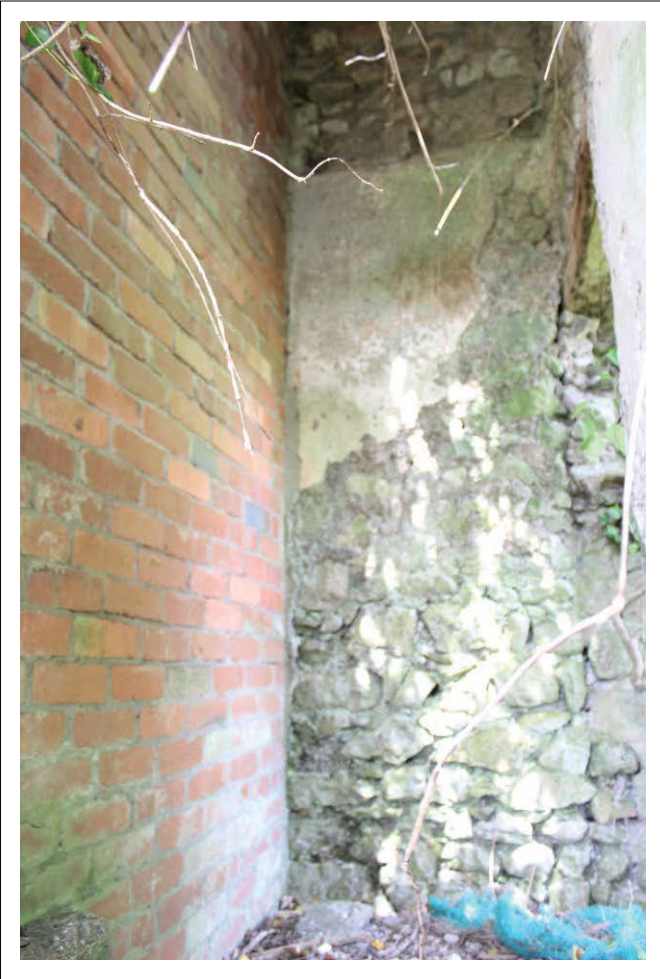
Plate 33: View north east showing internal view of later extension in north wall
