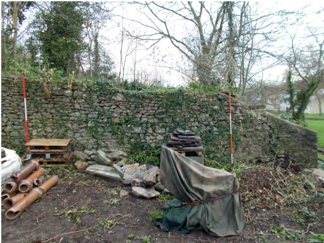
Plate 46: View south east toward east wall
