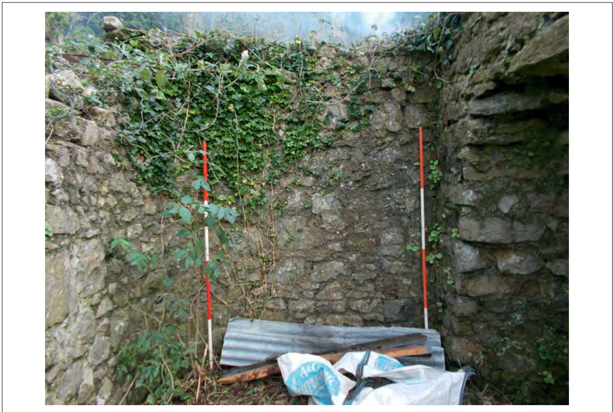
Plate 10: View north east toward south external wall
