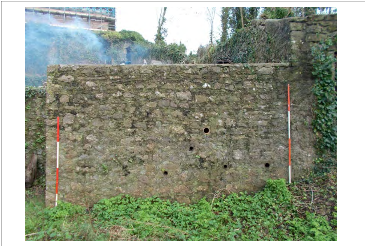
Plate 15: View north east toward south external wall
