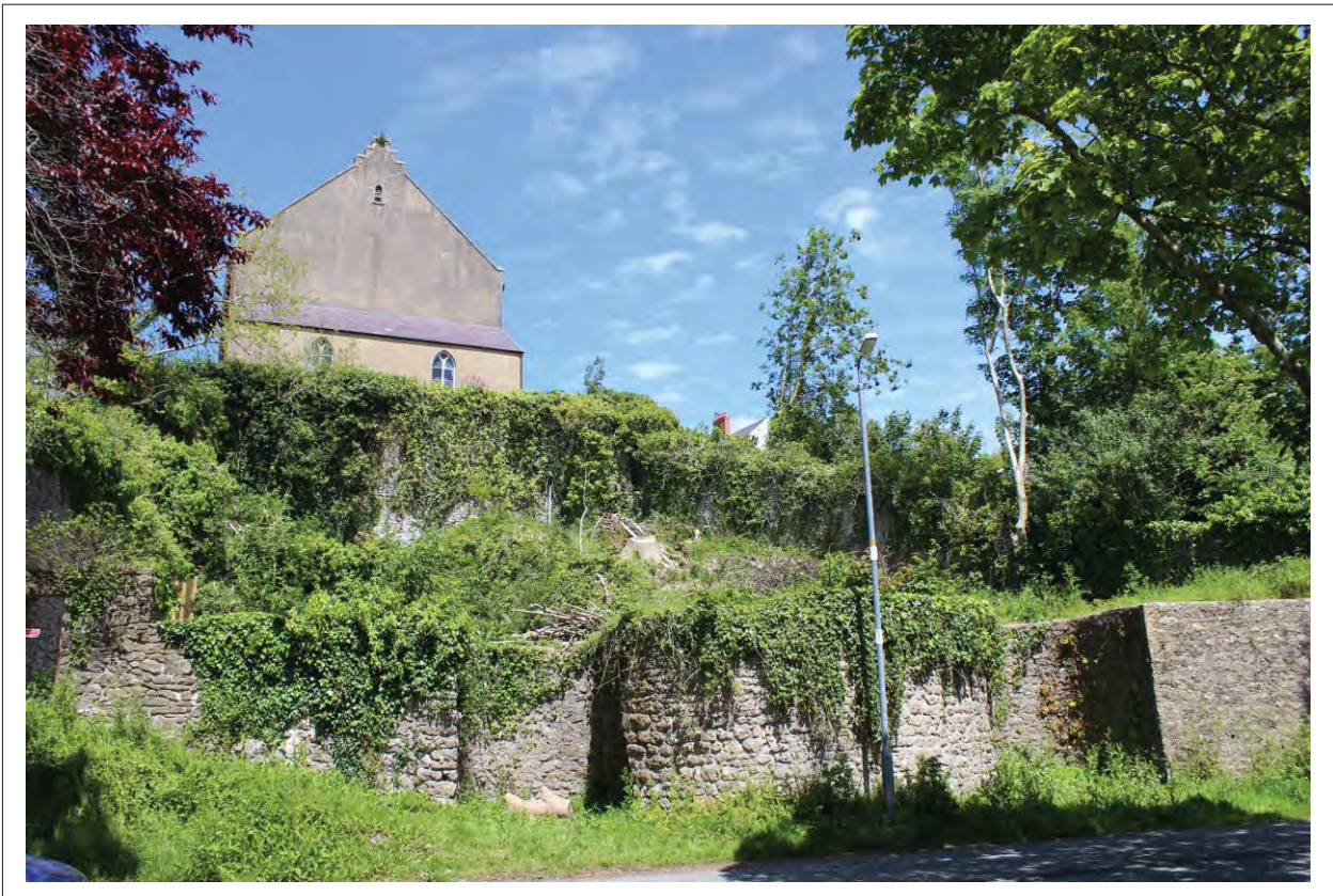
Plate 2: View north east toward south wall external elevation
