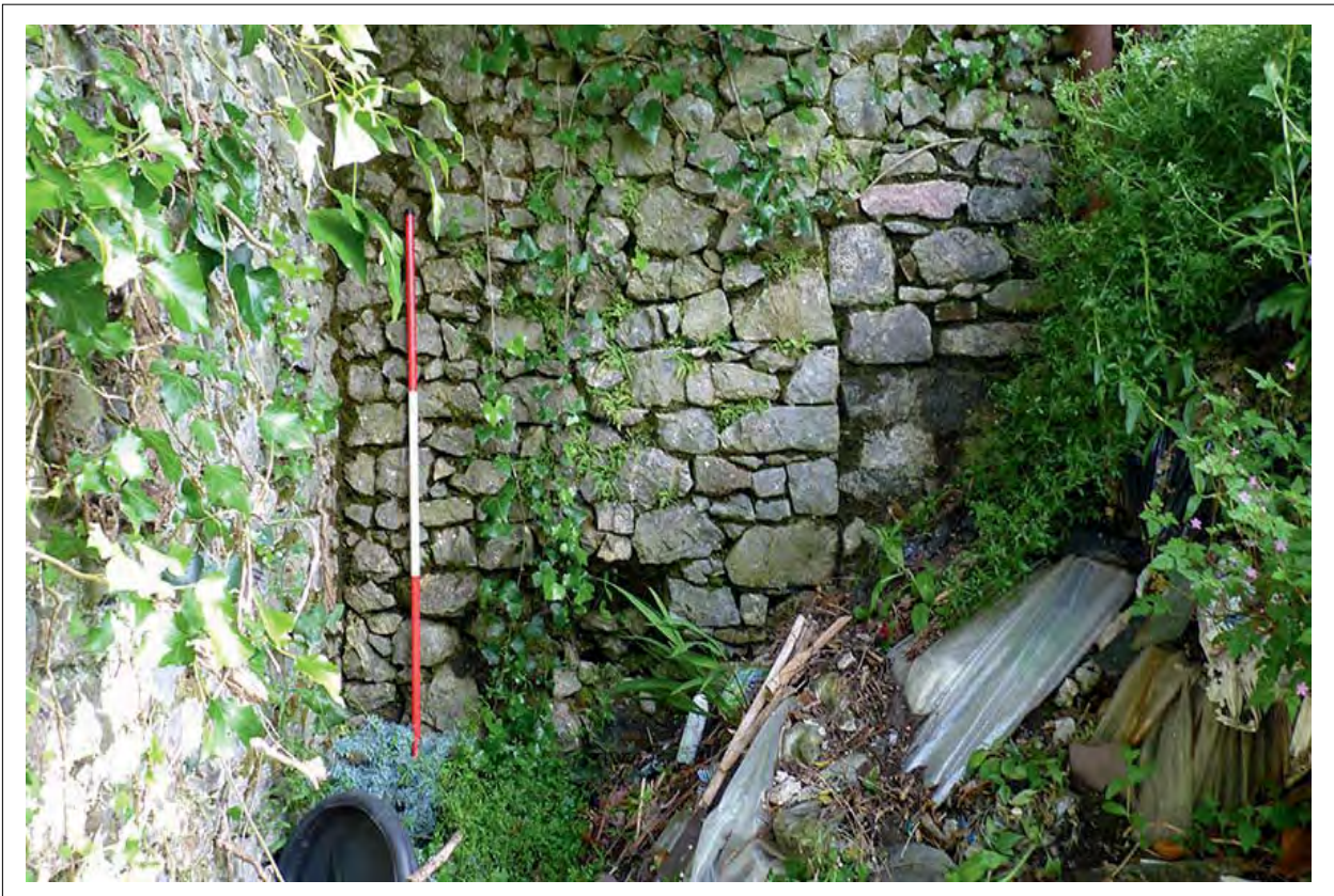
Plate 28: View north east toward north wall
