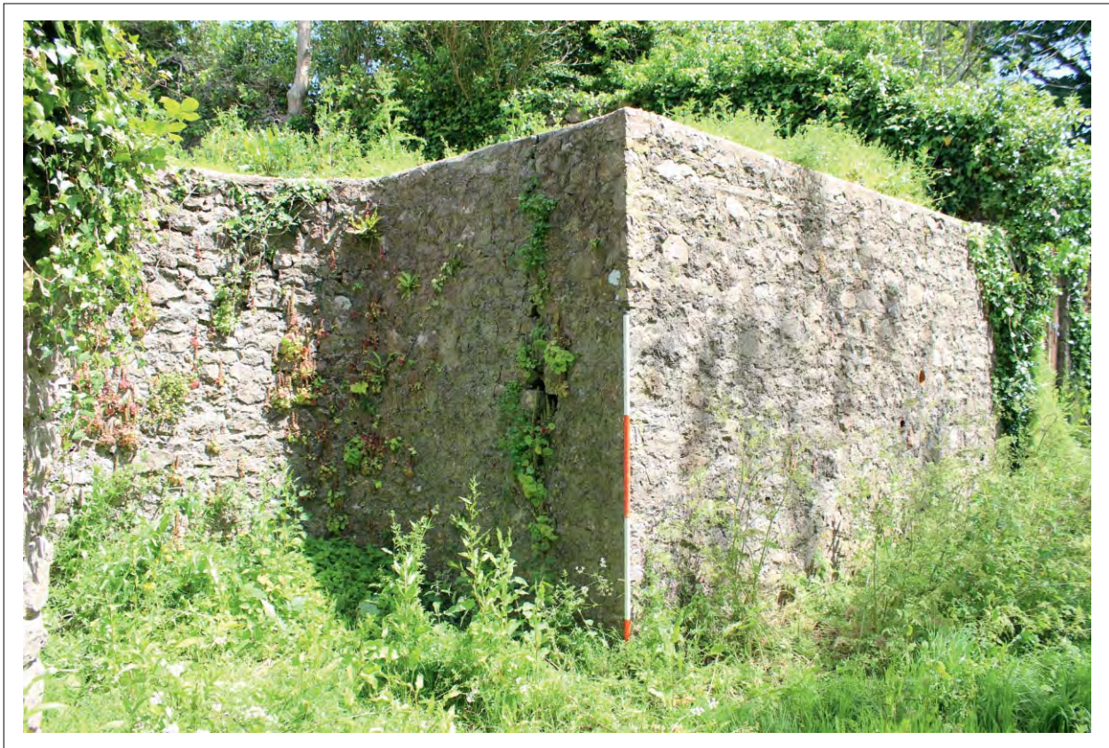
Plate 13: View east toward south external wall
