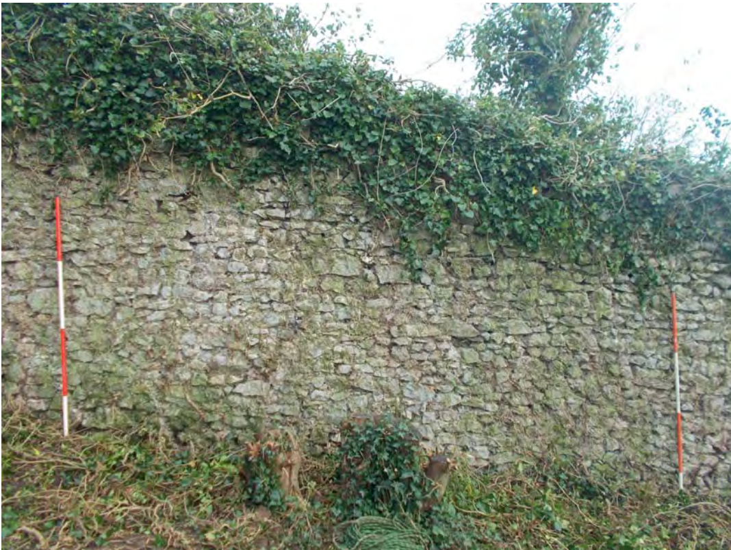
Plate 42: View south east toward east wall
