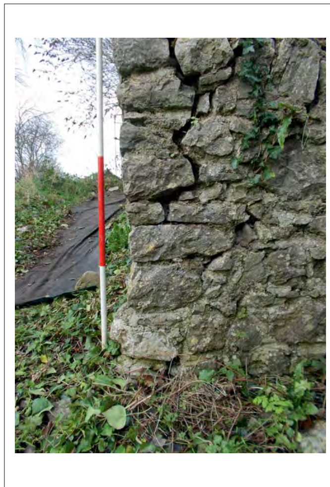
Plate 12: View north west toward detail of south external wall
