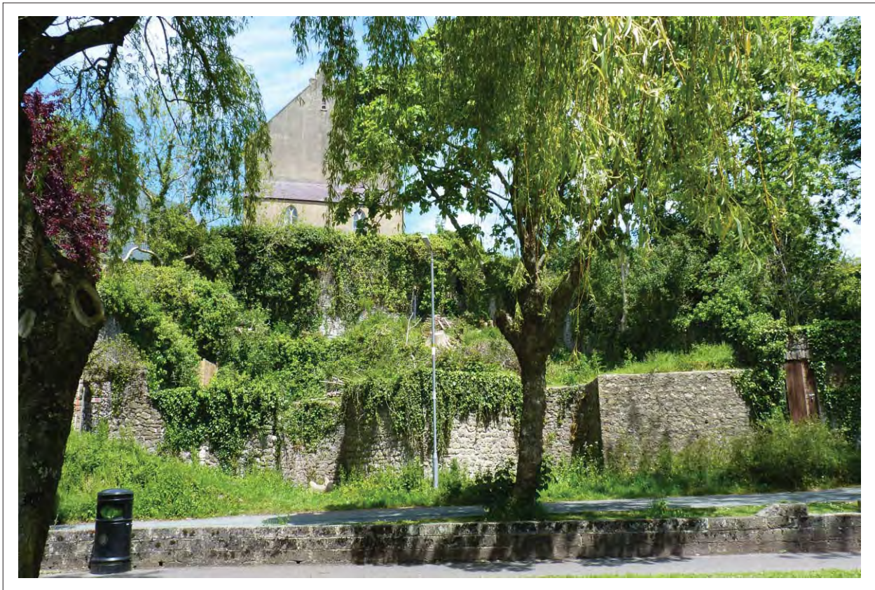
Plate 1: View north east toward south wall external elevation
