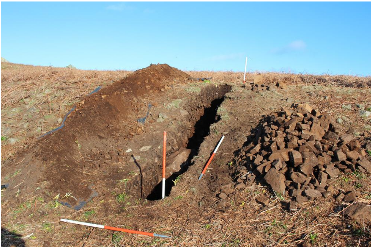
Figure 7. Post excavation view of the trench from the south-east with 1m scales. The quantity of stone removed from this very narrow trench can be appreciated. (DS2016_078_010)
