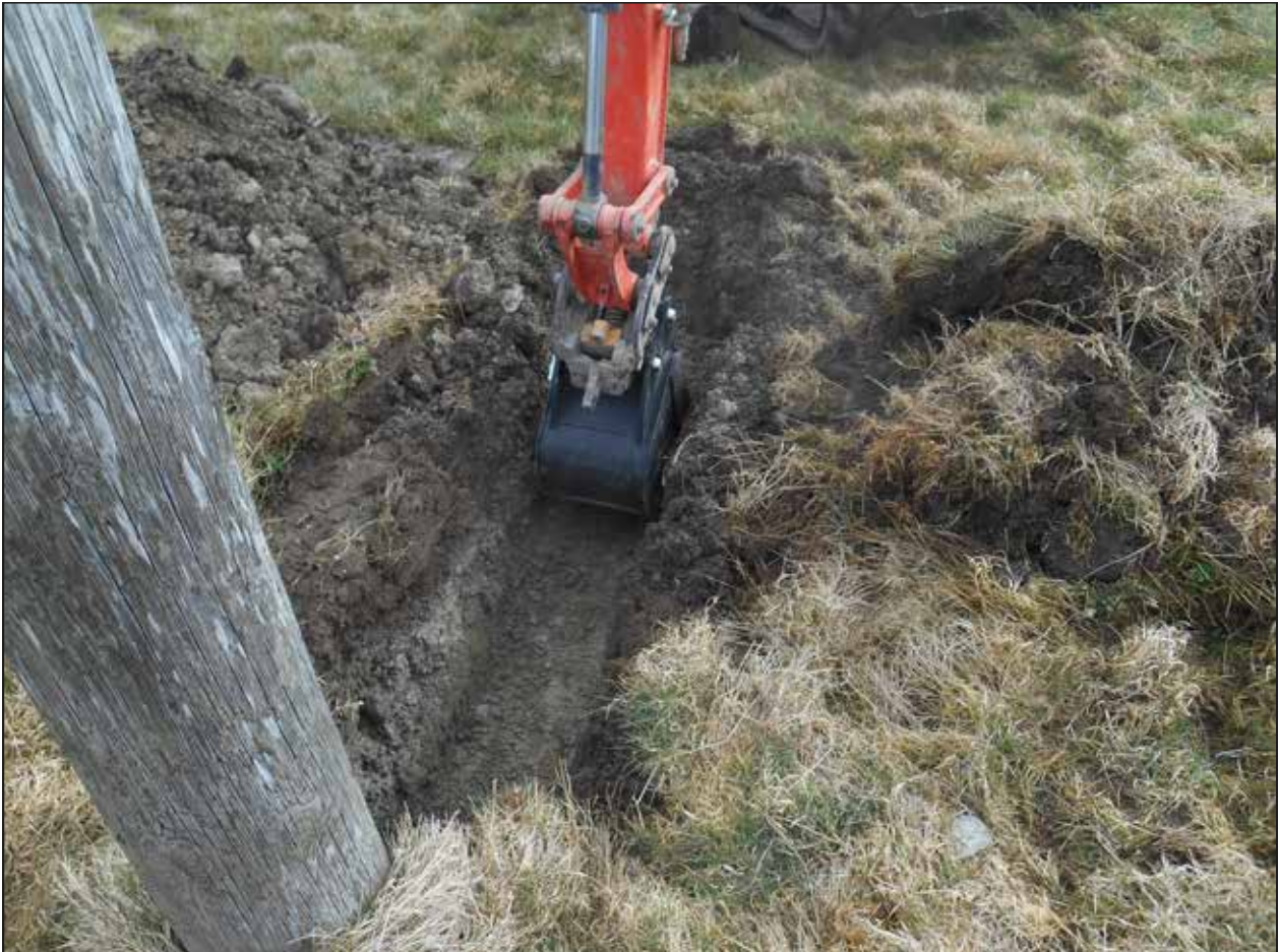
Plate 4. Working shot of Trench 1, looking south.
