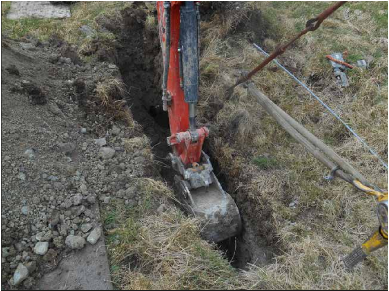
Plate 9. Working shot, Trench 2, looking north-east.
