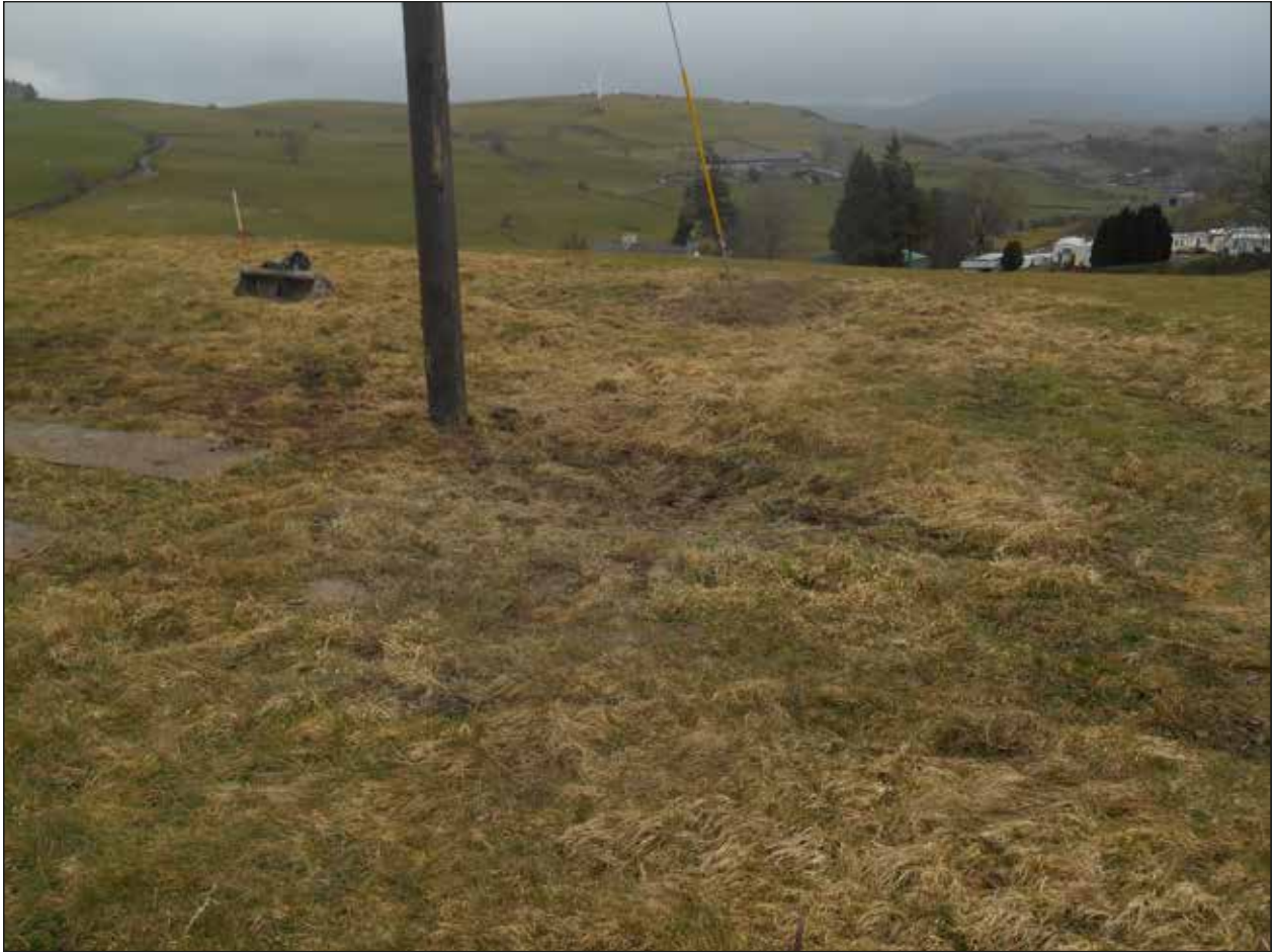
Plate 11. Pole and stay after backfill, looking south.
