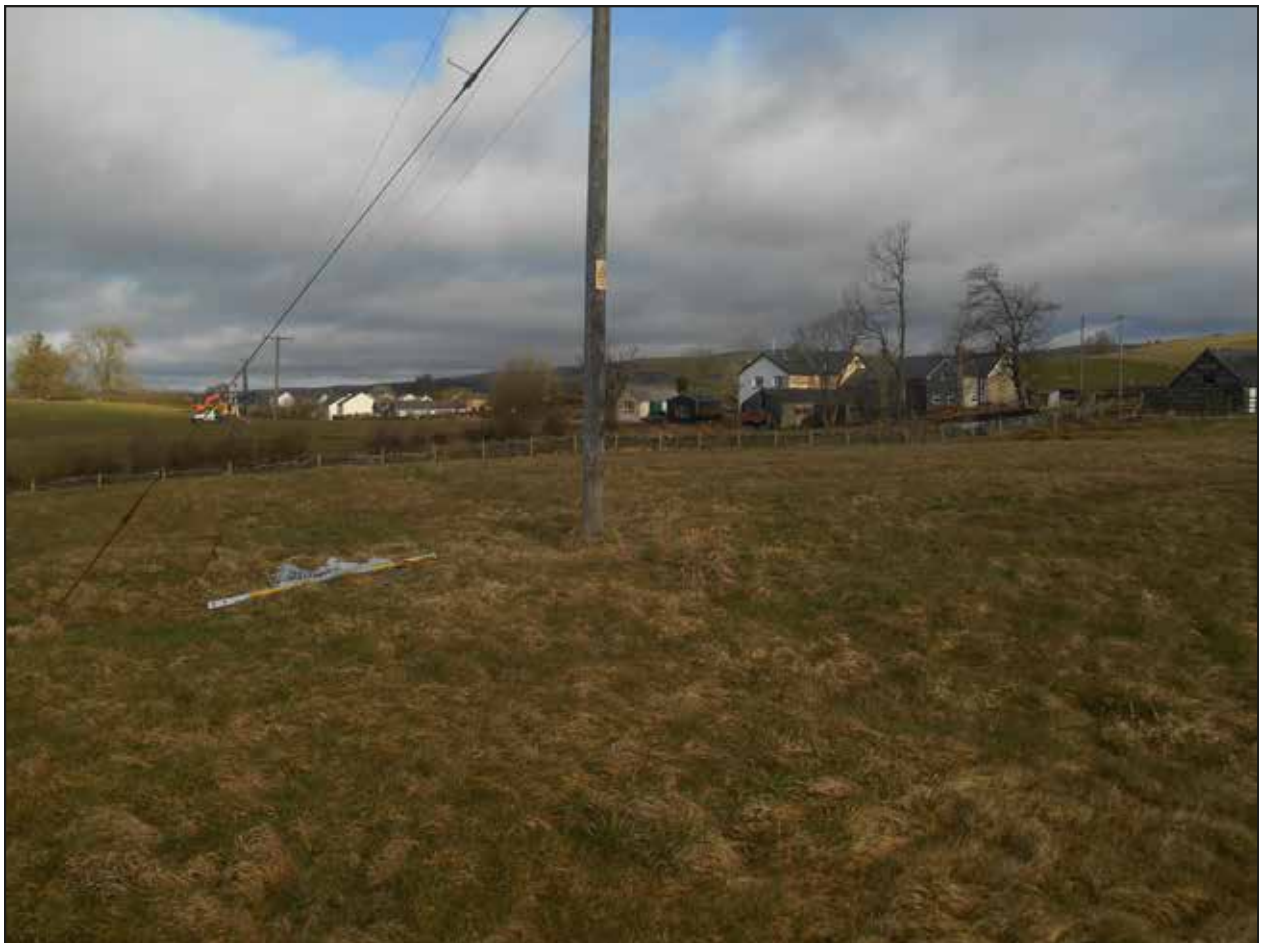
Plate 2. Original pole and stay before their removal, looking north.
