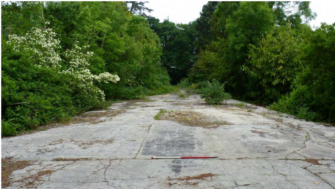
Photo 30: View north along the same modern concrete footings.
