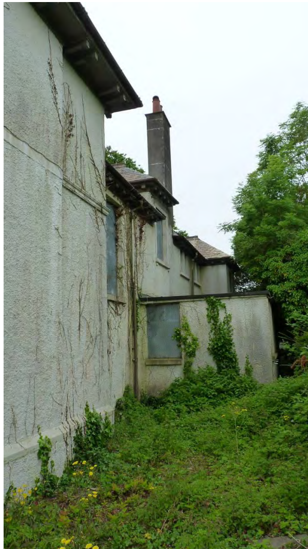
Photo 10: Rear of Coed Parc, view southwest.
