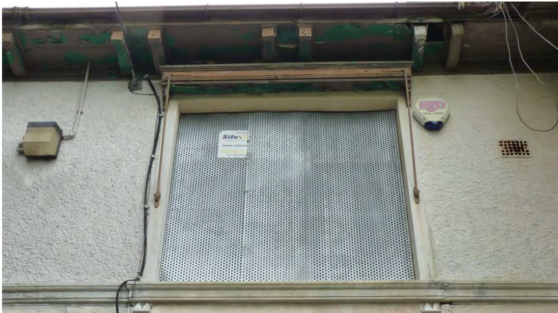
Photo 6: Detail of overhanging eaves and external roller blinds on windows.
