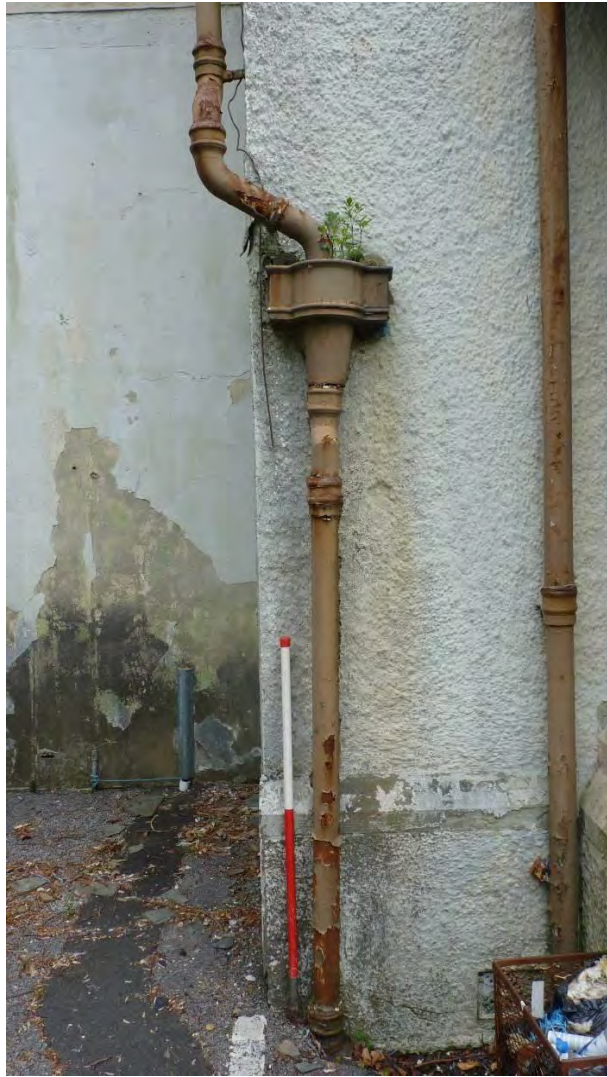
Photo 7: Detail of cast iron drain pipes on Coed Parc. 1m scale.
