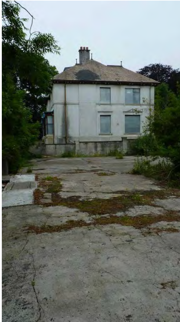
Photo 31: View west across the concrete footings towards Coed Parc.
