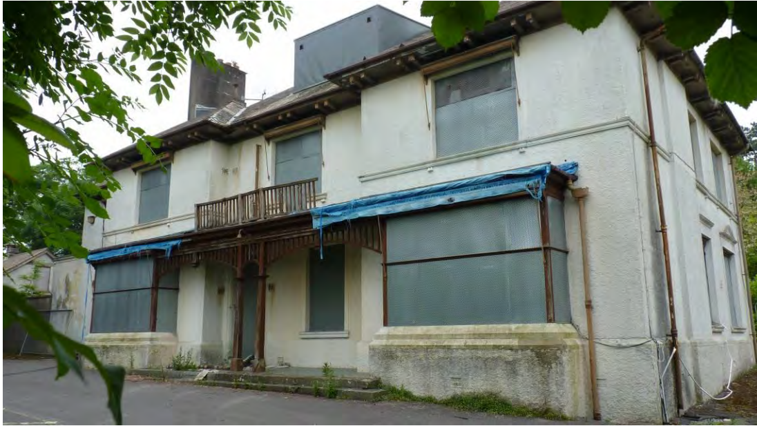
Photo3: Current condition of Coed Parc, facing northwest.
