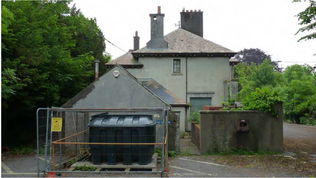
Photo 9: Western elevation of Coed Parc.
