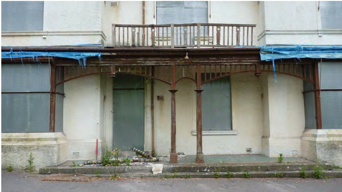
Photo 4: Front entrance to Coed Parc, showing wooden veranda.
