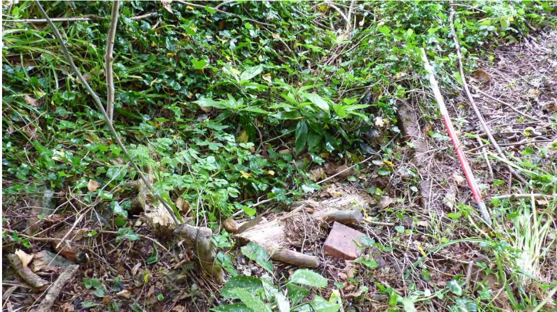
Photo 25: Wall footings for the former greenhouse and vinery in the northwest corner of the walled kitchen garden. Brick footings are visible just to the left of the 1m scale.
