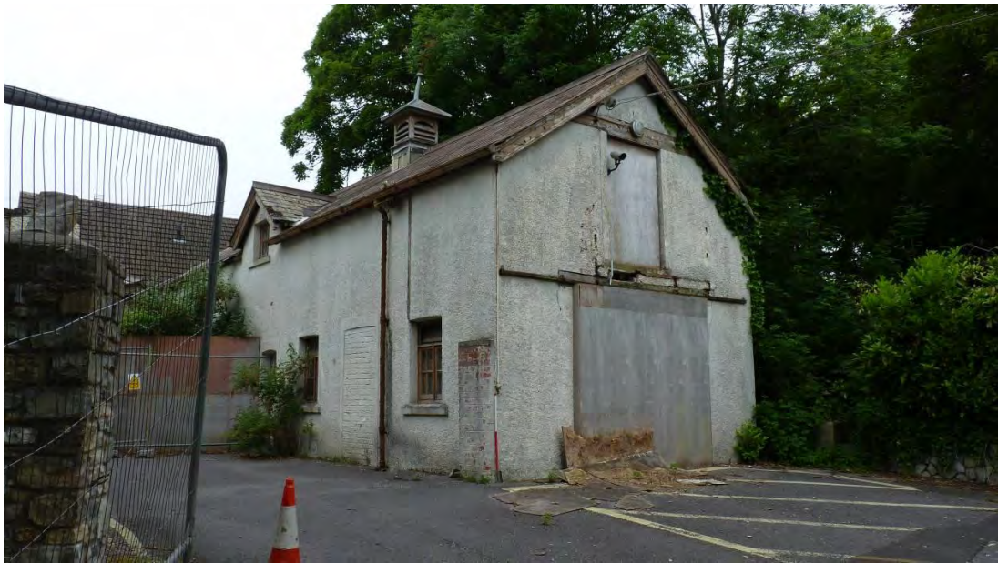
Photo 18: View northwest of the former Coach House. 1m scale.
