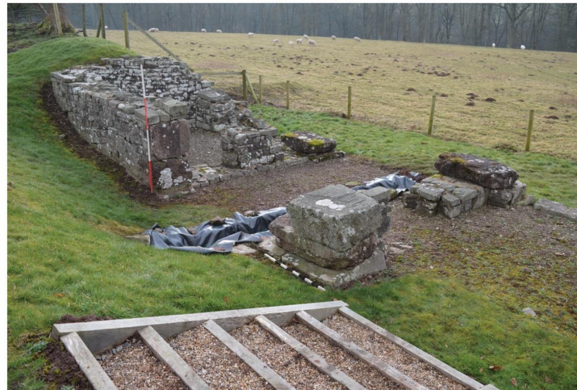
Fig. 16 South Gate: East Guardroom, view from the north-west c. 1925 (Wheeler 1926) and 2017 (Photo CPAT 4291-0056)
