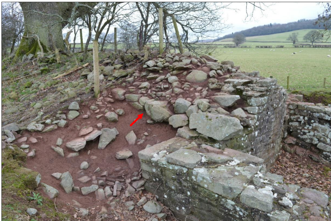
Fig. 5: The investigation of the rampart adjacent to the East Gate. Note the stone revetment (arrowed) thought be Wheeler to represent post-Roman rebuilding.
