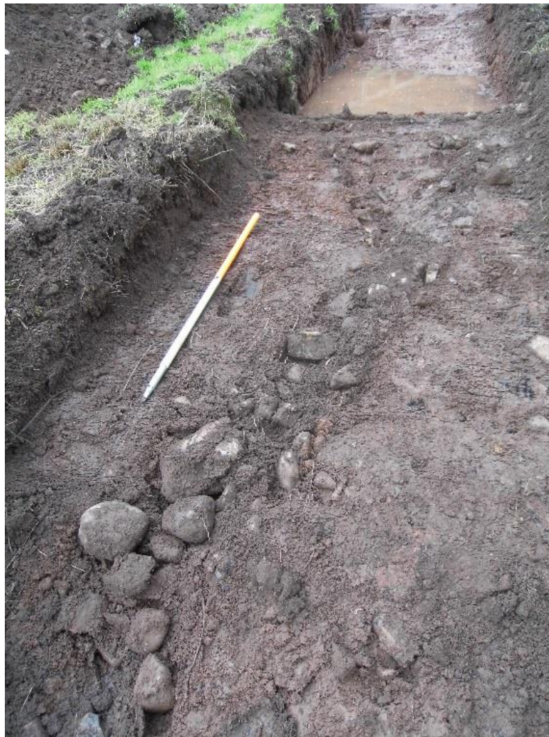
Plate 8: Detail of stone-filled land drains [806] and [808]
