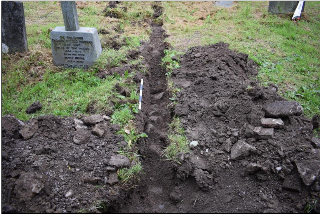
Fig. 4: Stone rubble at the change in direction of the trench
