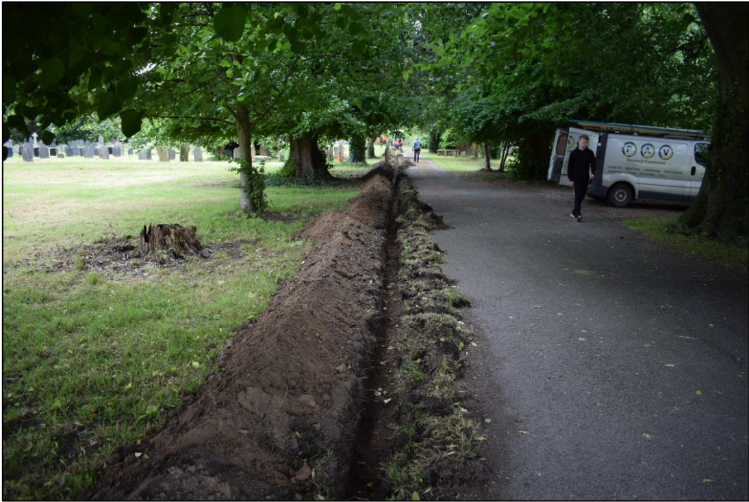
Fig. 2: Main section of trench alongside access path
