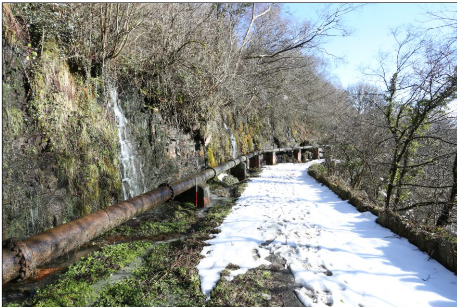
Plate 2: Pipeline section on low piers, viewed from west. Scale 1m
