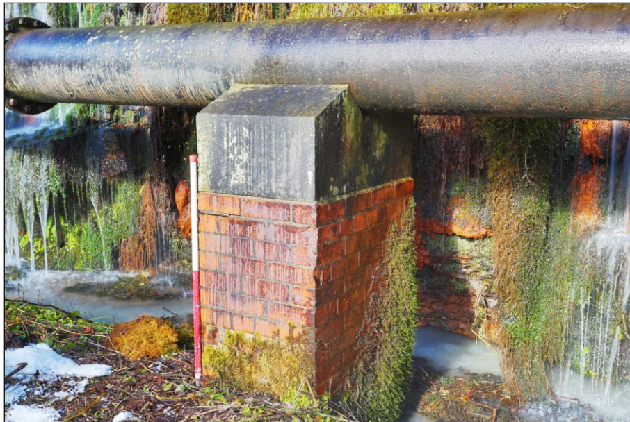
Plate 5: Typical small support pier and pipe cradle. Scale 1m
