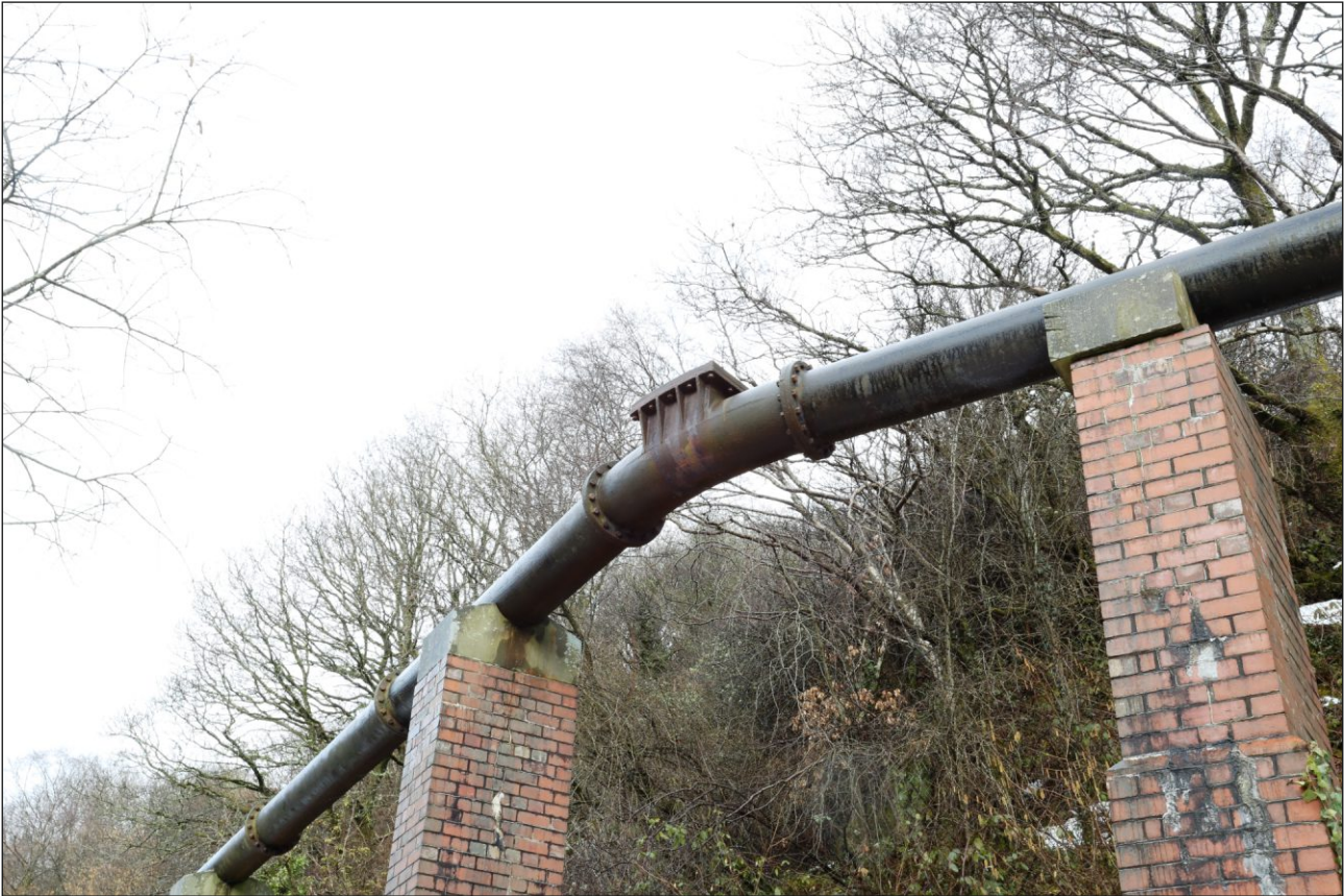
Plate 11: Angled connector and rodding hatch
