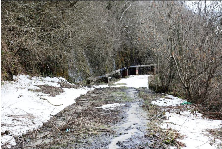
Plate 1: Pipeline emerging from ground at west end, viewed from west
