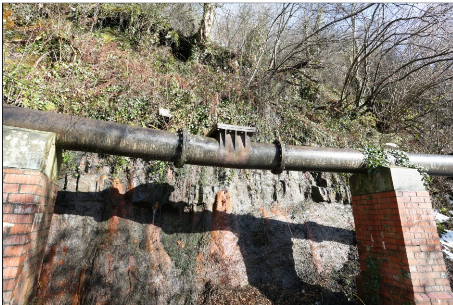
Plate 10: Angled connector and rodding hatch
