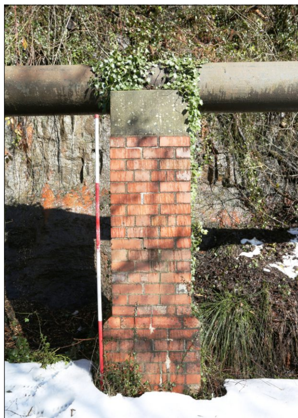
Plate 6: Typical intermediate pier with chamfered step in profile. Scale 2m
