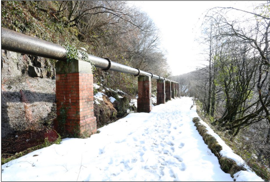
Plate 3: Pipeline on intermediate piers, viewed from west. Scale 2m
