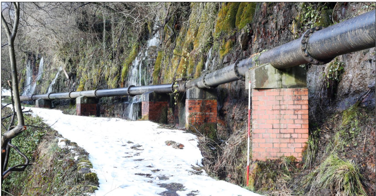
Plate 8: Pipe sections connected with bolted flanges
