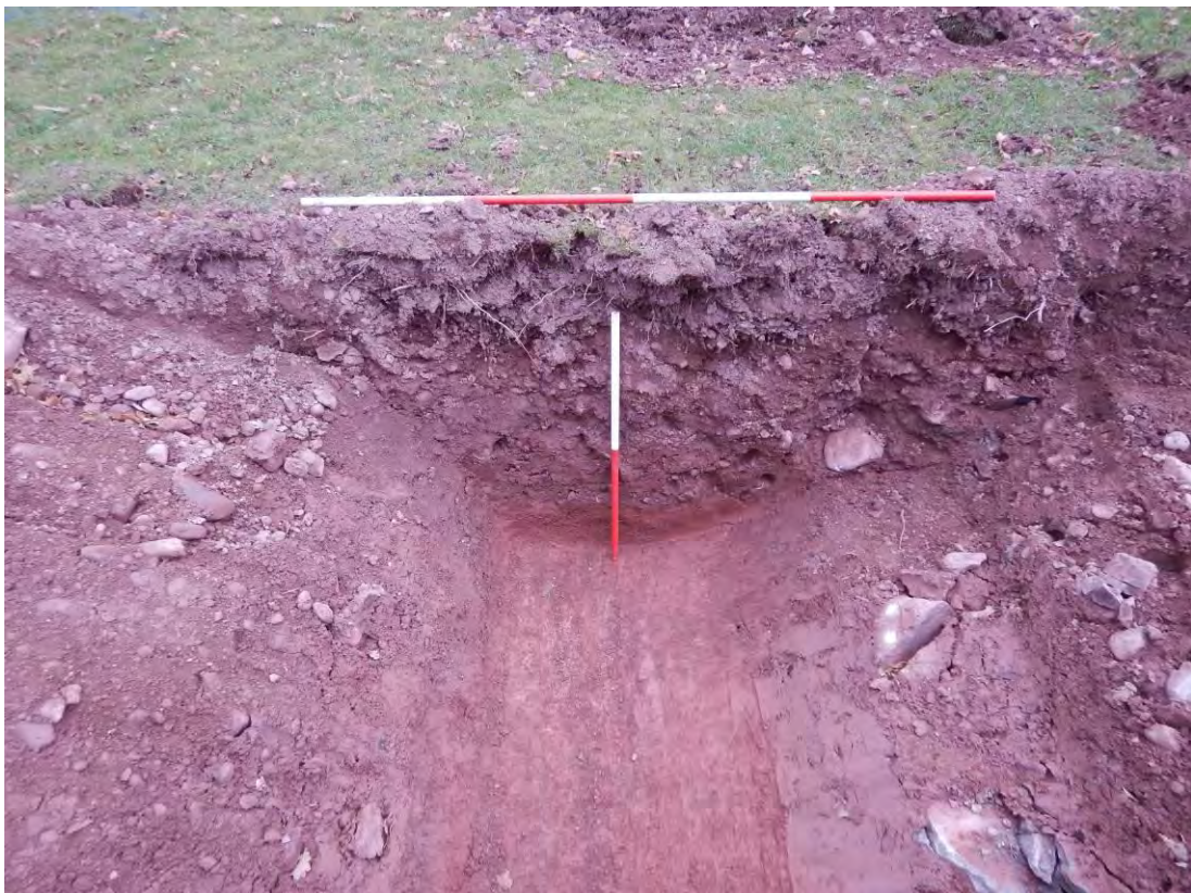
Photo 73: Trench 21, post-excitation, facing northeast. Machine excavated sondage to test the nature of the natural deposits. 1m & 2m scale.
