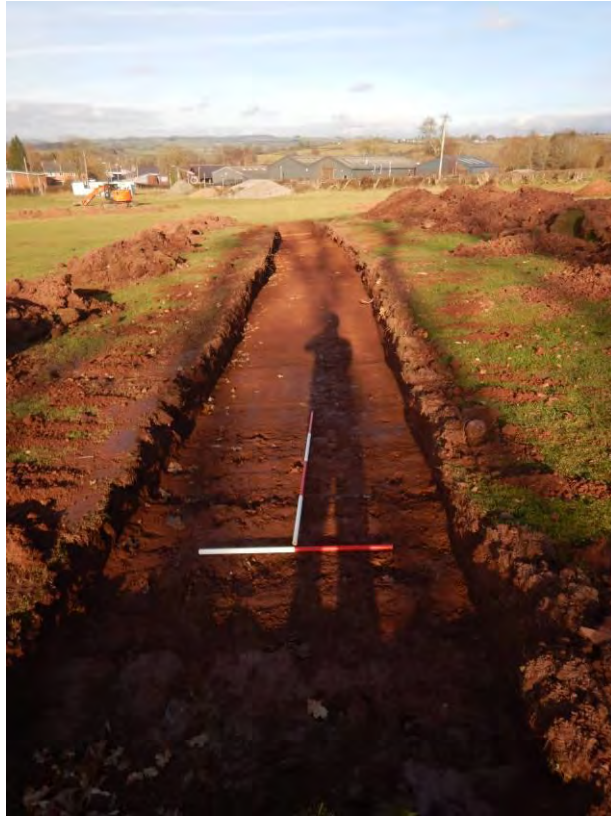
Photo 13: Trench 6, during excavation, facing north. 1m & 2m scale.
