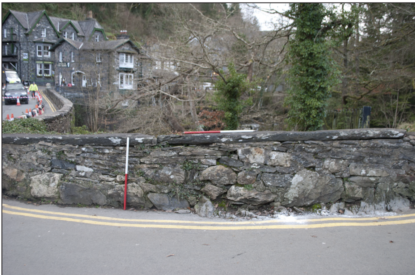
Plate 4: View of the northwest damaged coping stone area; scale: 2x1m (archive reference: G2587_027).
