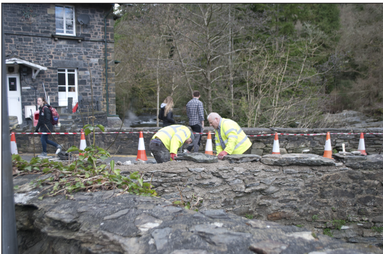
Plate 12: Placing capping stones; scale: not used (archive reference: G2587_029).
