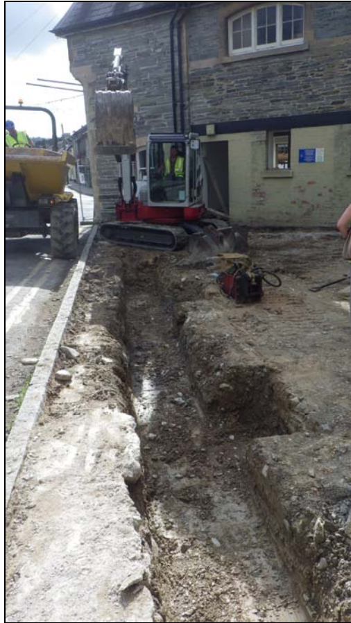
Plate 30: CHN2014_129: Mechanically excavated foundation trench, looking southwest.
