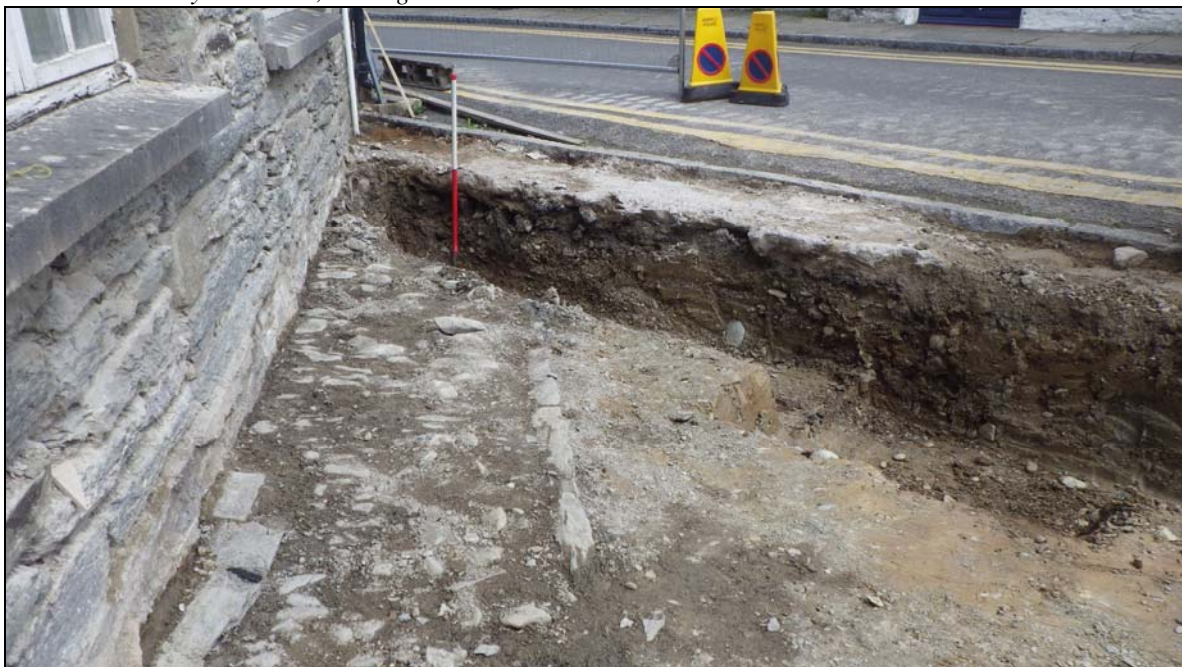
Plate 27: CHN2014_126: Eastern end of the cobbled pavement, 007, after the foundation trench for the new structure had been mechanically excavated, looking east southeast
