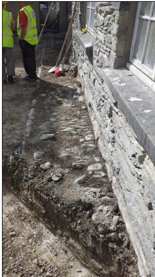
Plate 29: CHN2014_128: The foundation trench cutting cobbled pavement 007, looking west northwest.
