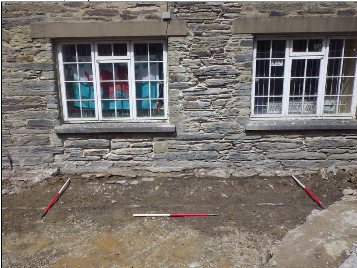
Plate 9: CHN2014_108: The eastern part of cobbled pavement 007, looking north northeast.
