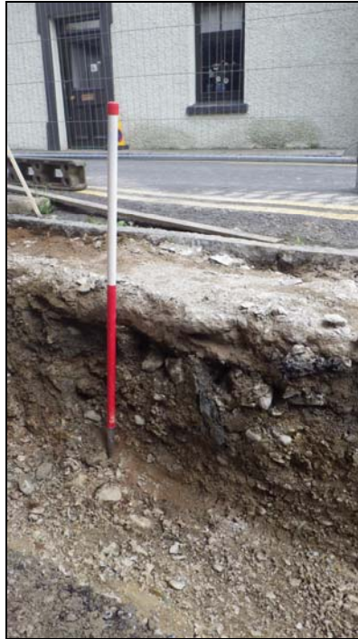
Plate 28: CHN2014_127: Detail of where the foundation trench cut the cobbled pavement 007, showing 003, 004, 005, looking east.
