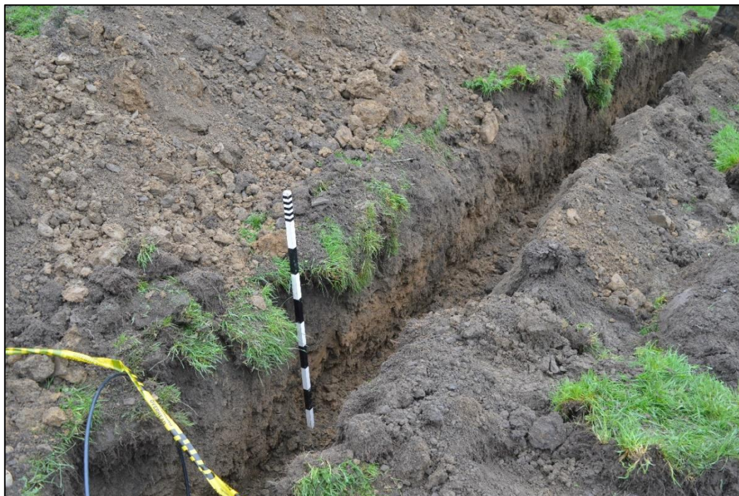
Fig. 6 View from the north along cable Trench 2/7 Photo CPAT 4499-0032
