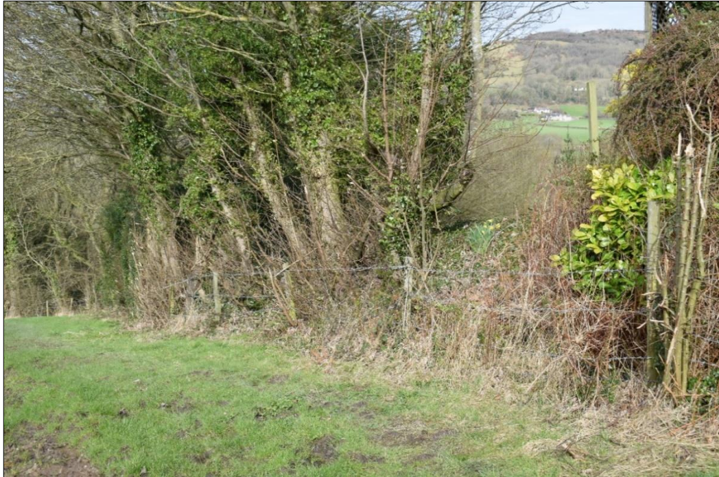
Offa's Dyke Unit 1: View from the south the escarpment with fence and trees CPAT 4315-0005
