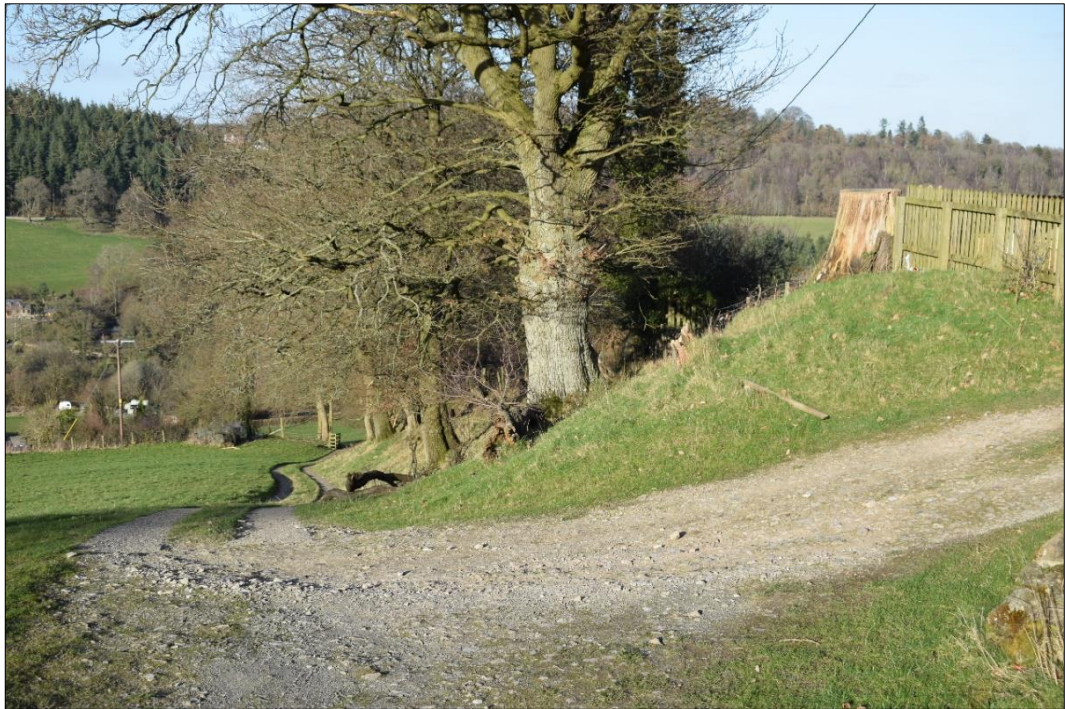
Offa's Dyke Unit 17: View from south-south-west of the vehicle erosion (Issue 3). CPAT 4315-0019
