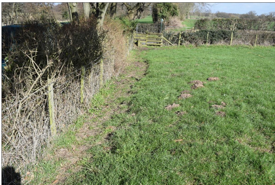
Wat's Dyke Unit 12: View form south of stock erosion (Issue 1) alongside the boundary. CPAT 4317-0069
