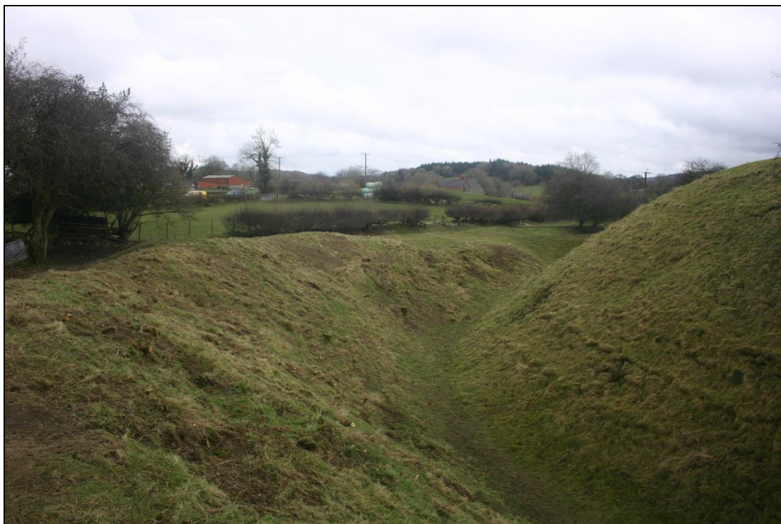
Fig. 8 View of the outer defences, after conservation. Photo CPAT 3791-0219
